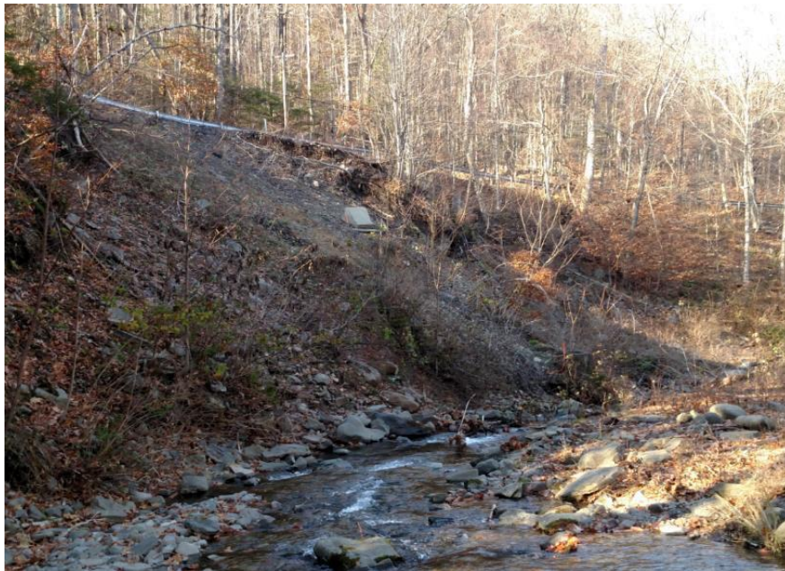
Figure 4.9 Bush Kill at Watson Hollow before construction.
