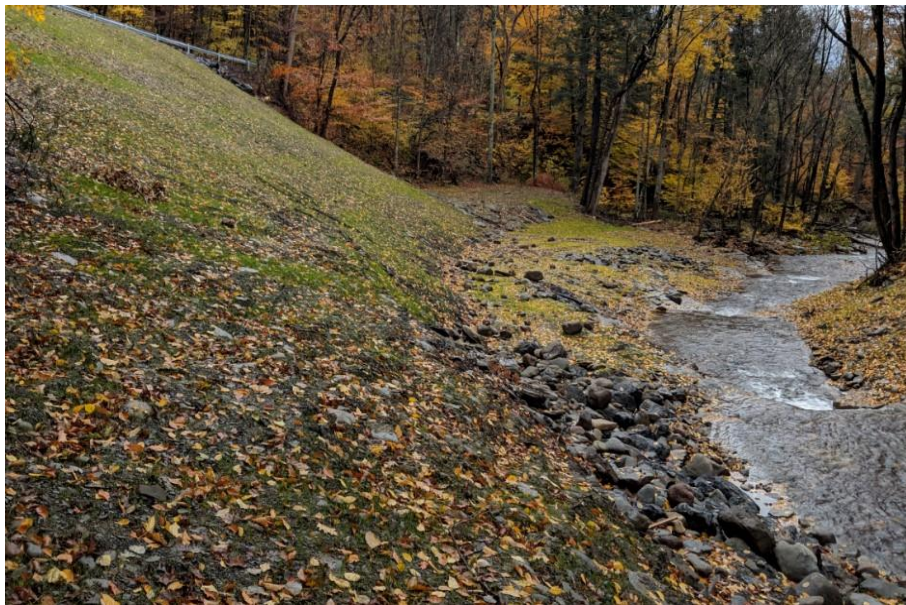
Figure 4.10 Bush Kill at Watson Hollow after construction.
