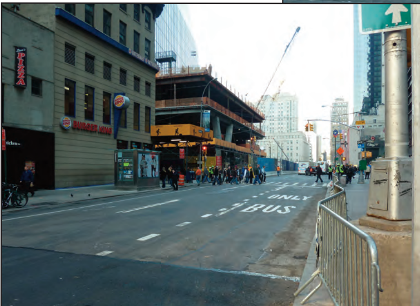
3. View north along Church Street from Cedar Street.
