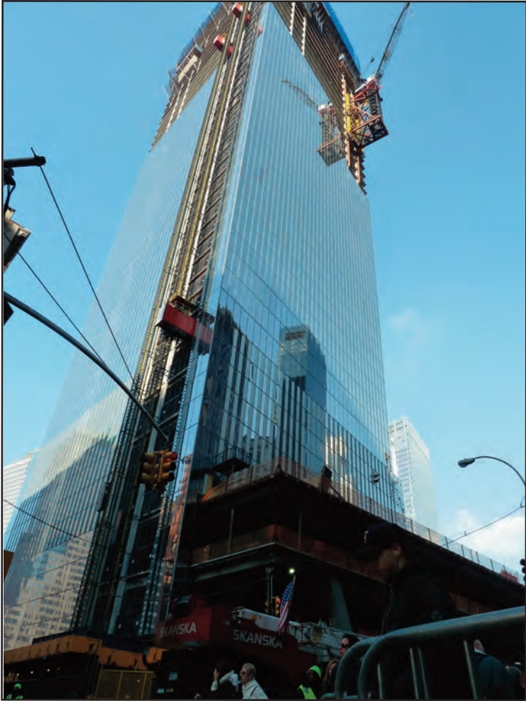
4. View west across Church Street from Liberty Street.
