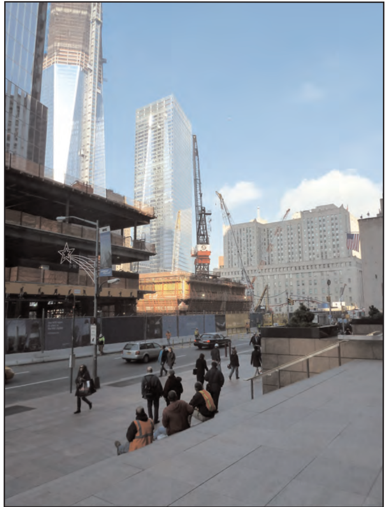
5. View northwest across Church Street from Liberty Street.
