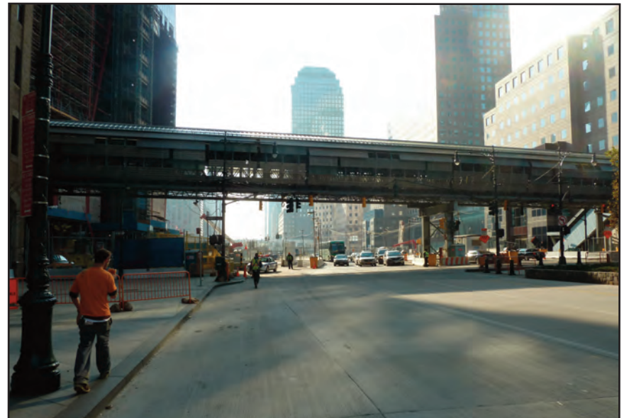
14. View south along West Street/Route 9A from Barclay Street.
