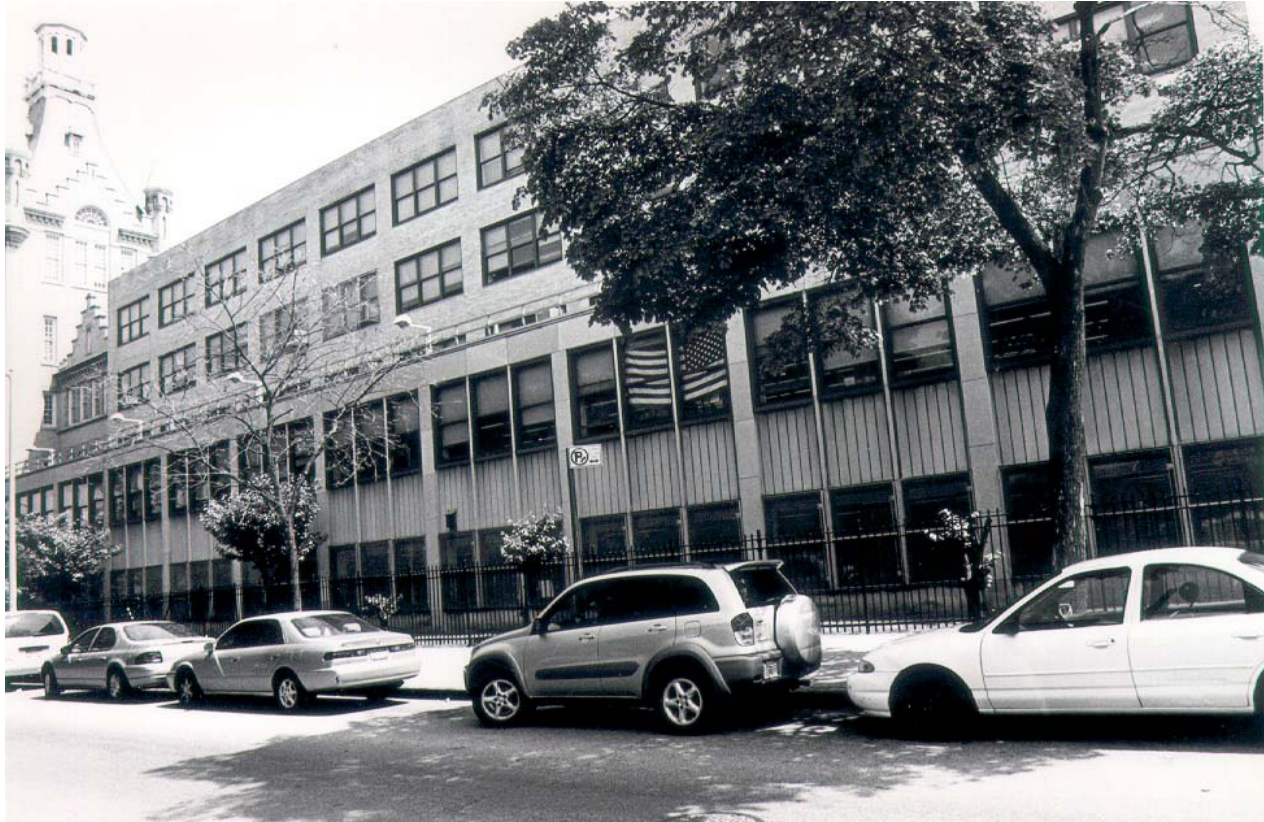
Newtown High School, Borough of Queens Southwest wing (1956-58)
