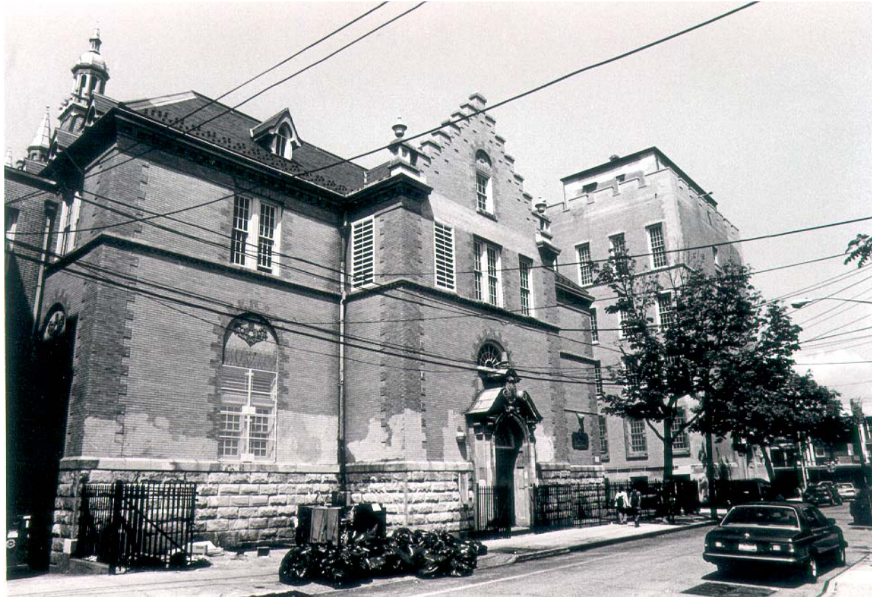
Newtown High School, Borough of Queens Auditorium wing (1920-21)
