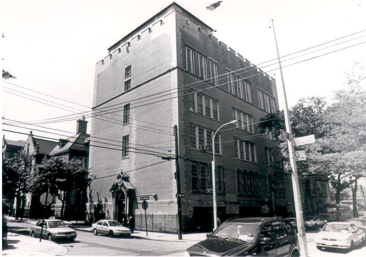
Newtown High School, Borough of Queens Northeast wing (1930-31)
