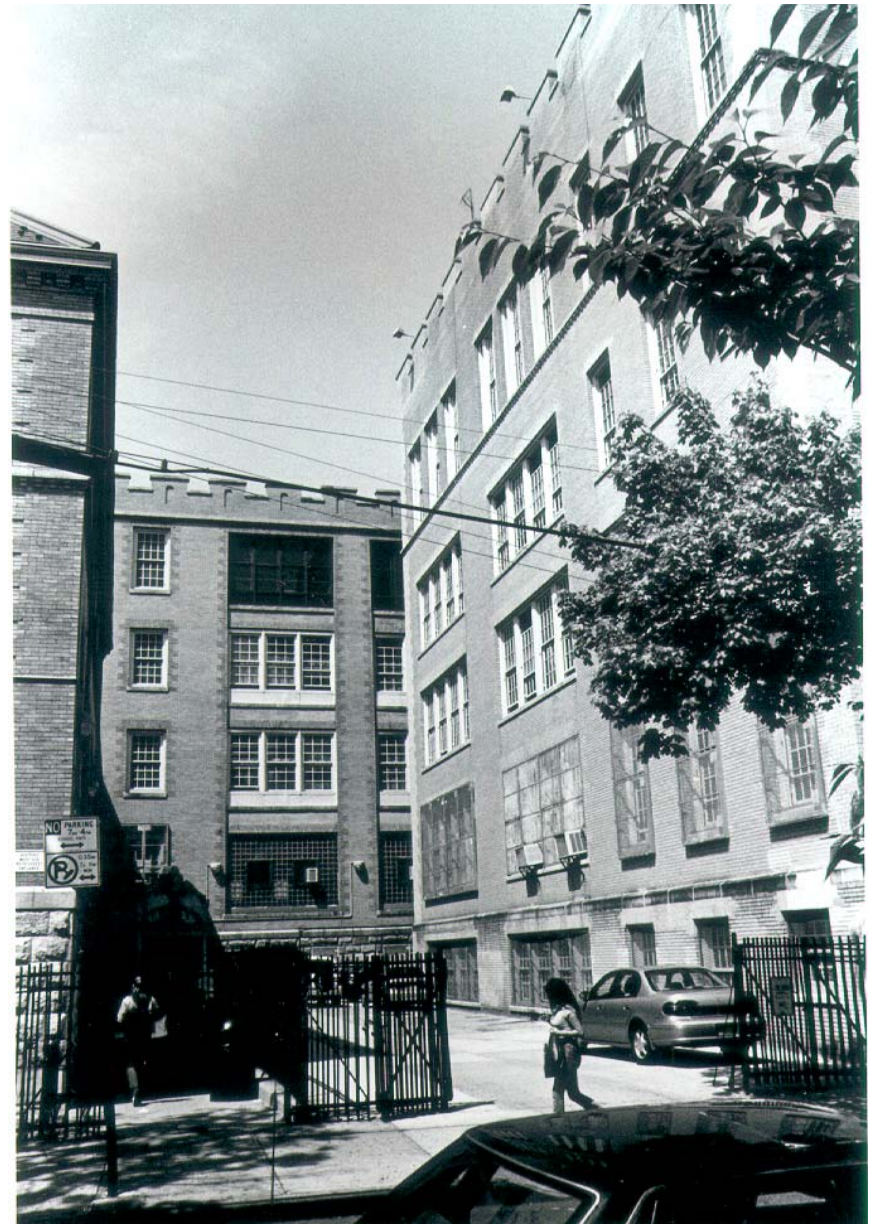
Newtown High School, Borough of Queens Northeast wing (1930-31)
