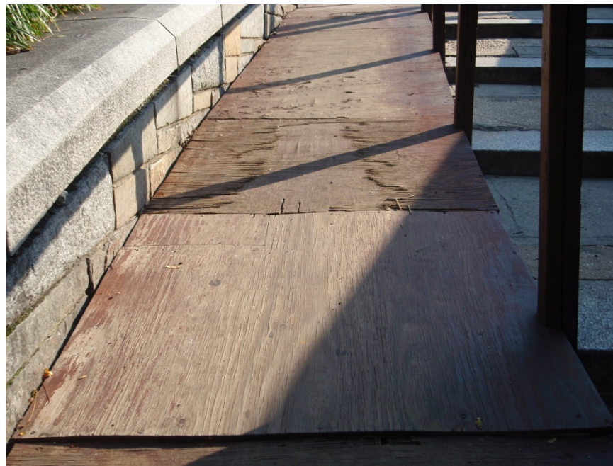
Photograph #4. West 79th Street Boat Basin Café. Deteriorated, uneven, and excessively sloped ramps.
