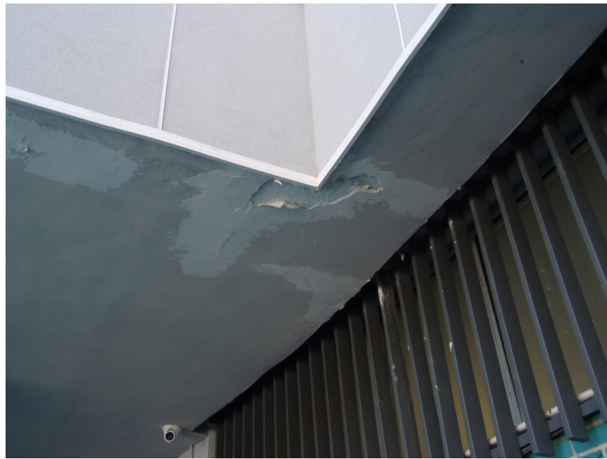
Photograph #6. Lasker Rink. Water damaged soffits at parapet walls.
