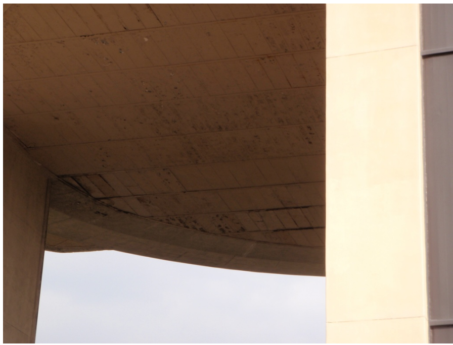
Photograph #8. Terrace in the Park. Water damaged panels at exterior soffit.
