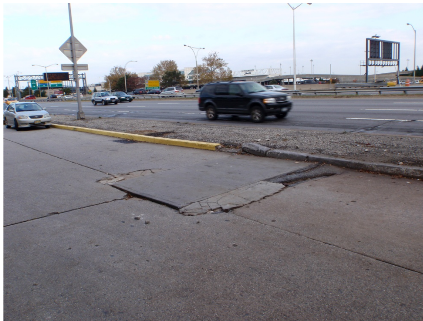
Photograph #2. Grand Central Parkway Gas Station. Cracks and deteriorated concrete pavement.
