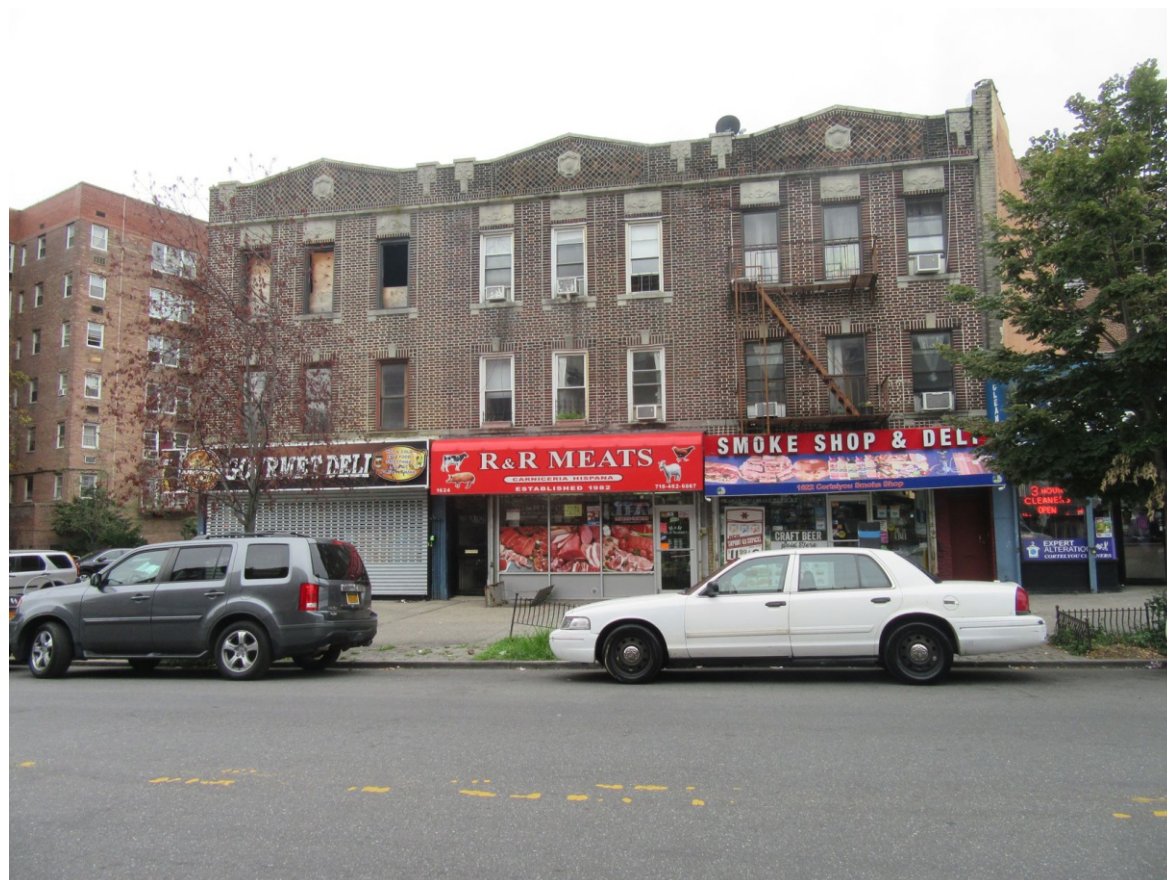
9. View of the Project Area facing south from Cortelyou Road.
