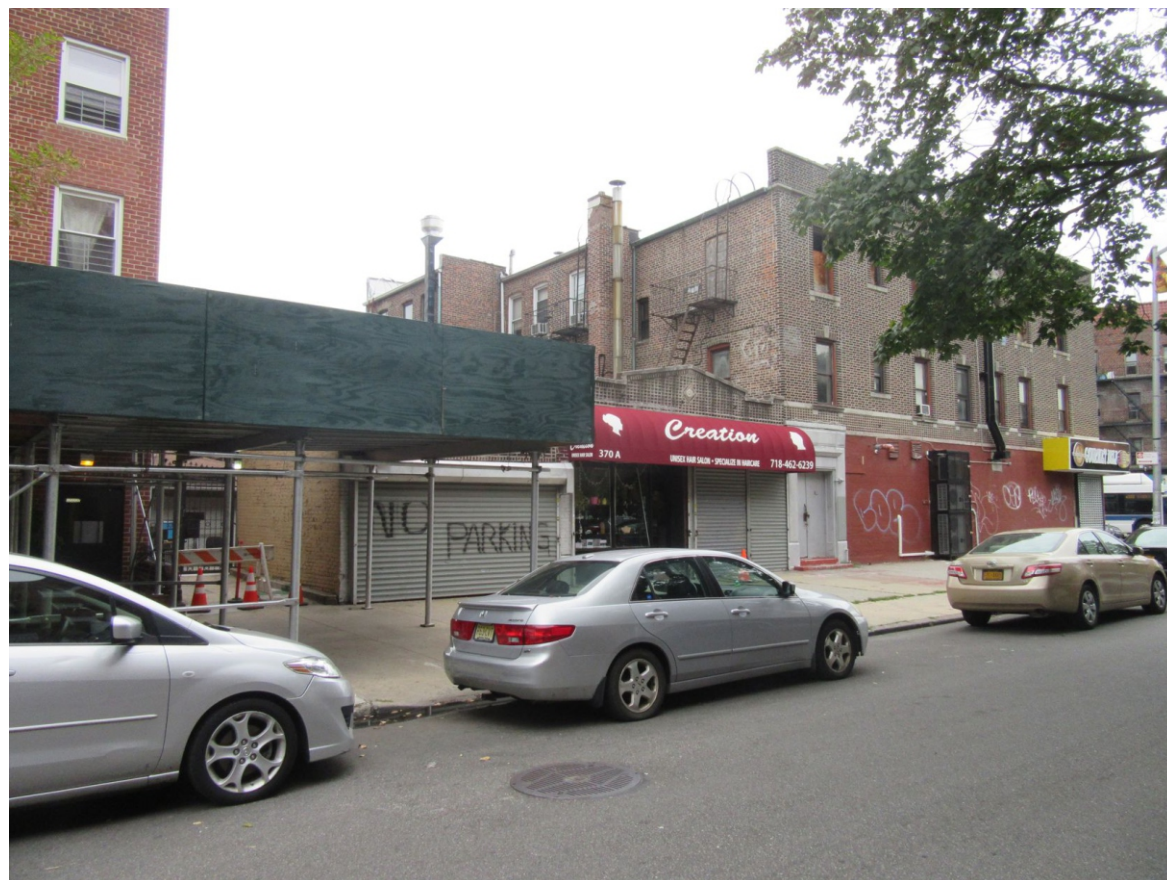
15. View of the Project Area facing northwest from East 17th Street.
