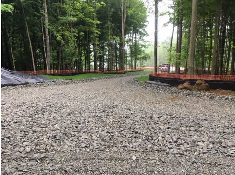
Figure 1: Construction Driveway at Drewville Road
