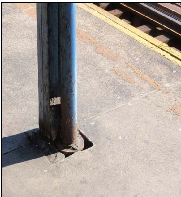
Concrete Broken Away at Base of Drain Pipe at the Elder Ave Station
