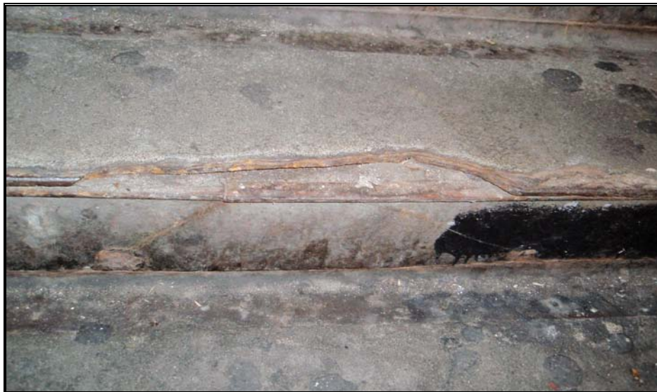
Photograph 6 Damaged Step Tread at the Smith and 9 th Streets Station
