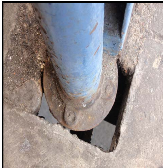
Concrete Broken Away at Base of Drain Pipe at the Elder Ave Station
