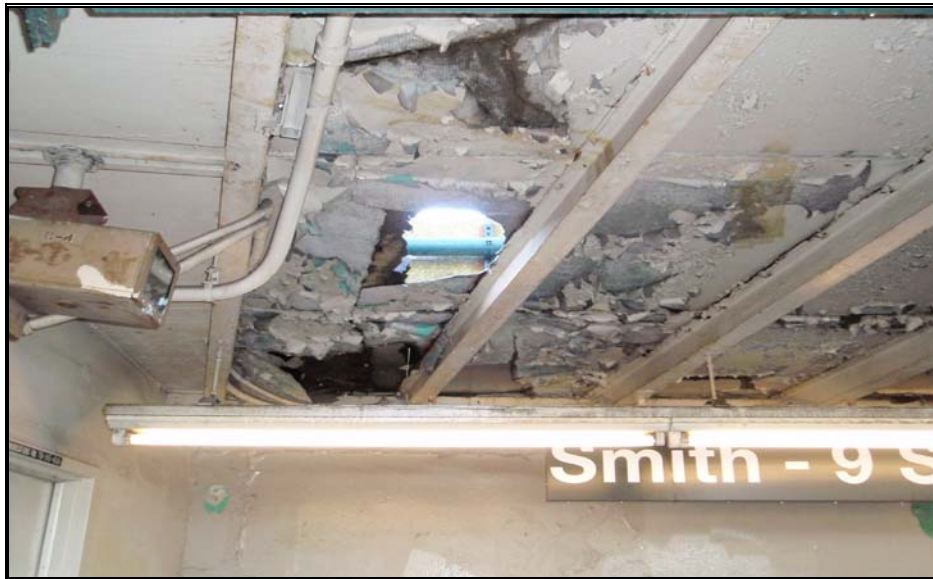
Photograph 6 Damaged Step Tread at the Smith and 9 th Streets Station
