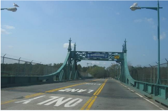
City Island Road Bridge, looking west
