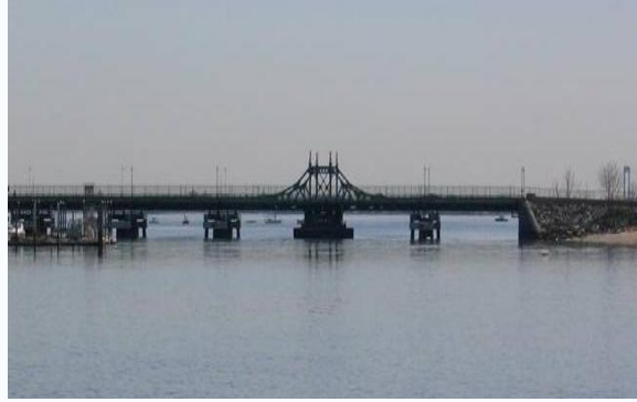
City Island Road Bridge, looking north
