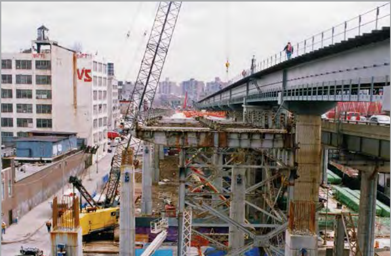
Williamsburg Bridge reconstruction in the 1990s
