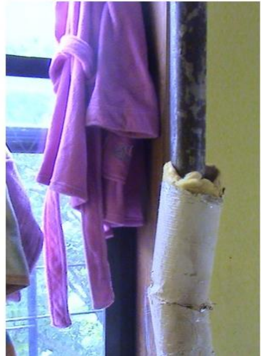
Figure 7: Mike's House (hotel): A 5th floor apartment. Evidence of mold in the bathroom (left): exposed heating pipe in the resident's children's room (right). The exposed portion would be reachable by the children (ages 3, 5, and 7).
