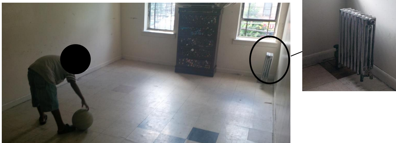
Figure 4: A cluster resident's empty living room (left). According to the resident, the caseworker and the superintendent took all the furniture from the apartment and she did not know why. Additionally the resident's radiator was uncovered and protruding from the wall, easily accessible to her six children (close-up, right).
