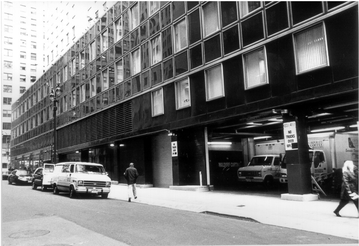
Socony-Mobil Building 41 st Street façade, loading docks, looking west
