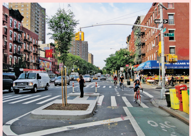
Pedestrian refuge islands on First Avenue between Houston and 34th Streets shorten crossing distances and provide physical protection for the bicycle lane.
