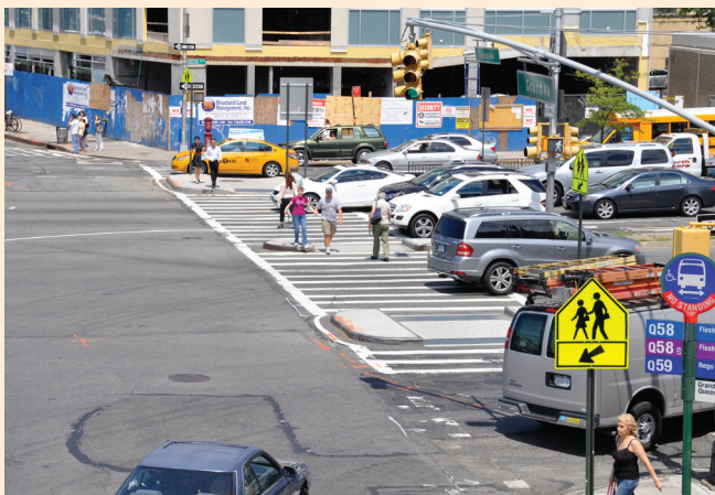
Extending and widening the median tips at Queens Boulevard and Broadway reduced crossing distance for pedestrians.
