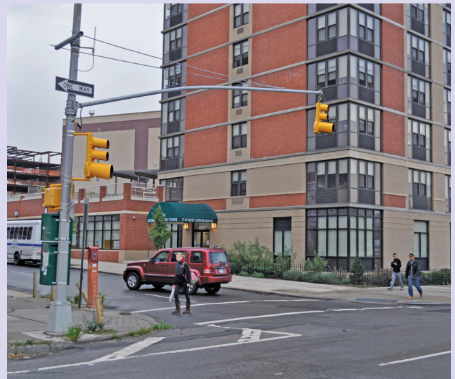
A new signal and crosswalk were added at the intersection of Hoyt Avenue South and 29th Street to improve safety in front of a newly constructed senior housing facility.
