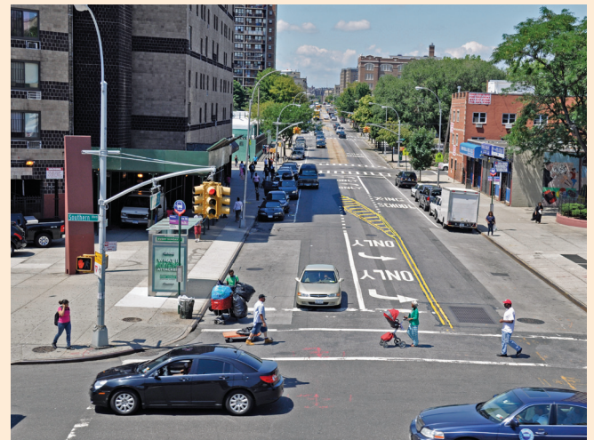
Left-turn lanes were added at 21 locations along the East 180th Street corridor to improve safety and traffic operations.
