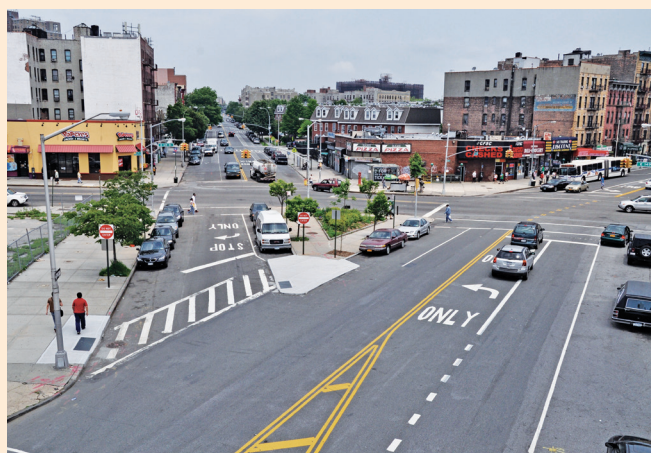
The Greenstreets triangle at Southern Boulevard and Prospect Avenue was extended by removing an un-used bus-only lane.
