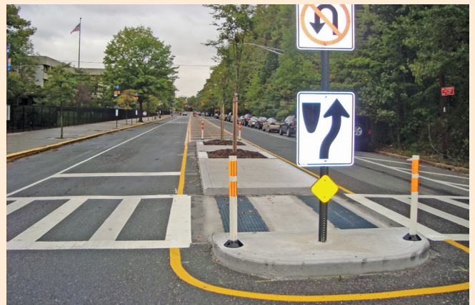
A pedestrian safety island was installed in the north crosswalk of Luten Avenue at Eylandt Street to improve safety specifically for the Tottenville High School students and all pedestrians at this intersection.
