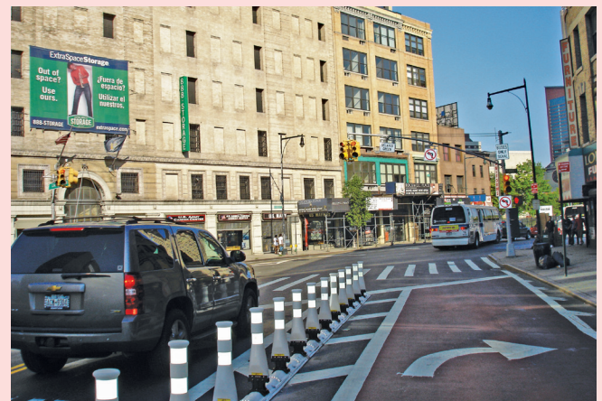
Right-turning vehicles were separated from buses on eastbound Livingston Street at Flatbush Avenue by bollards and a dedicated bus signal was installed to allow buses a five second head start to make the turn onto Flatbush Avenue.
