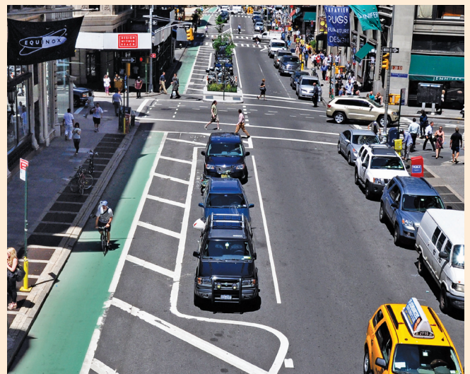
A parking protected bicycle path and landscaped, pedestrian safety islands were added along Broadway between 23rd Street and 18th Street.
