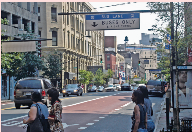
Bus lanes were painted red and large overhead signs were installed along the corridor to increase the visibility of the bus lanes.
