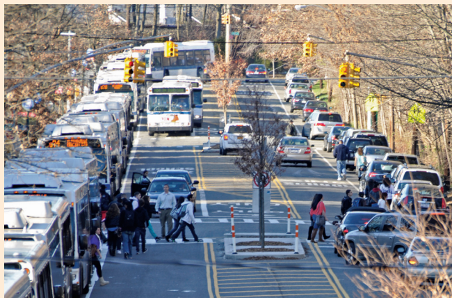
A painted center median with left-turn bays and pedestrian safety islands were installed along Luten Avenue from Amboy Road to Hylan Boulevard to calm traffic and enhance safety for all road users.
