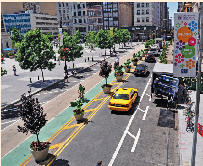
17th Street between Union Square West and Park Avenue South was converted from two-way to one-way westbound. New sidewalk connections, a bike lane and farmers' market parking were added to improve safety, mobility and curb-side access.
