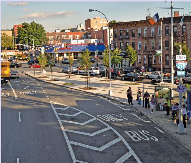
Two new landscaped crosswalk connections were added on Astoria Boulevard between 31st Street and 33rd Street to improve safety and enhance the streetscape.
