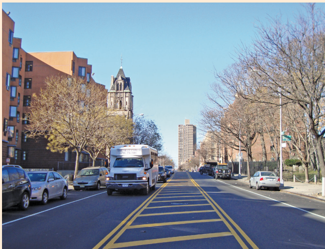
Traffic calming measures applied on East 180th Street included the narrowing of the travel lanes from 17 feet to 11 feet and the addition of painted center medians and parking lanes.
