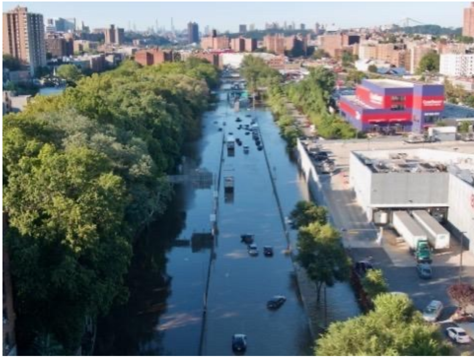
Areas across the city experienced flooding, including highways like the Major Deegan Expressway in the Bronx.
