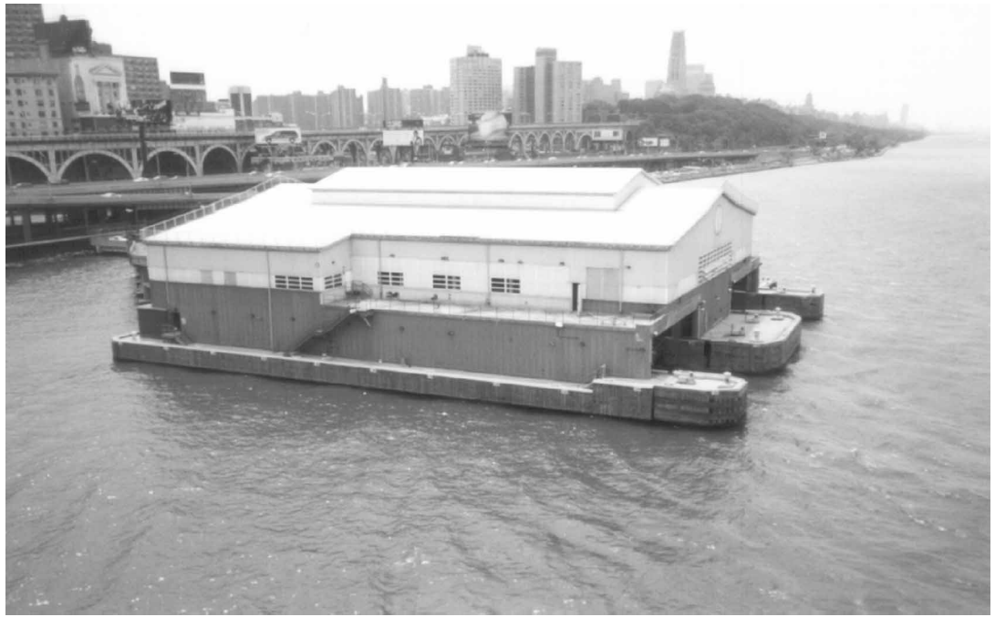
Figure 21.7-5 : View of the MTS and site from the southern edge of Riverbank State Park. (Photo 2000)
