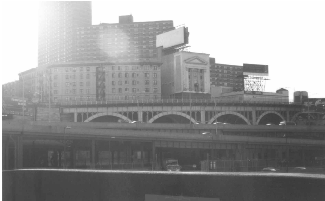
Figure 21.7-4 : View looking east from the site. (Photo 2000)
