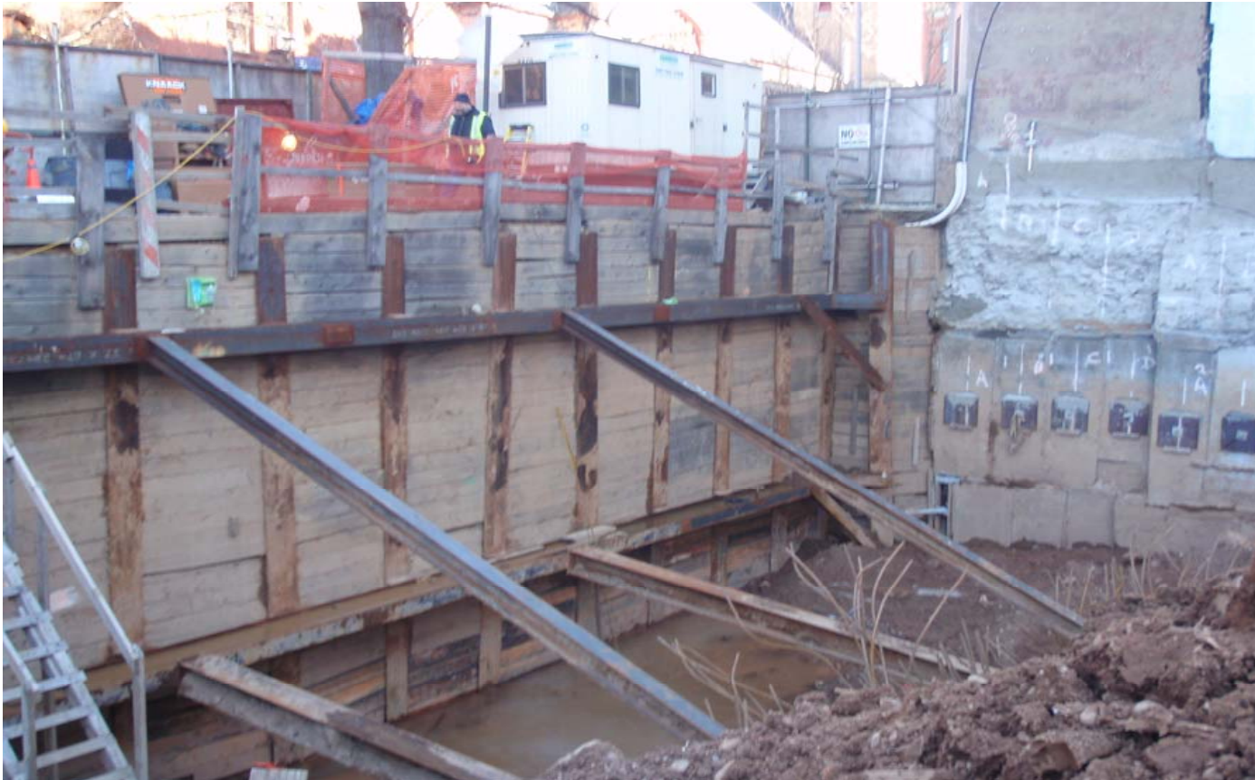
15-foot deep excavation close to the sidewalk
