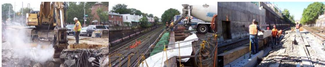
Demolition of the 17<sup>th</sup> Avenue Bridge Deck. Casting the New East Abutment Wall.
