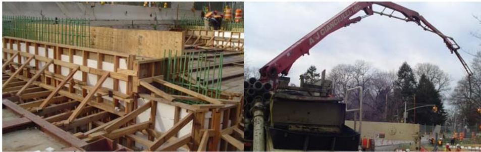
West 252<sup>nd</sup> Street Bridge Formwork and Rebar Fabrication at the Pier and West Abutment.
