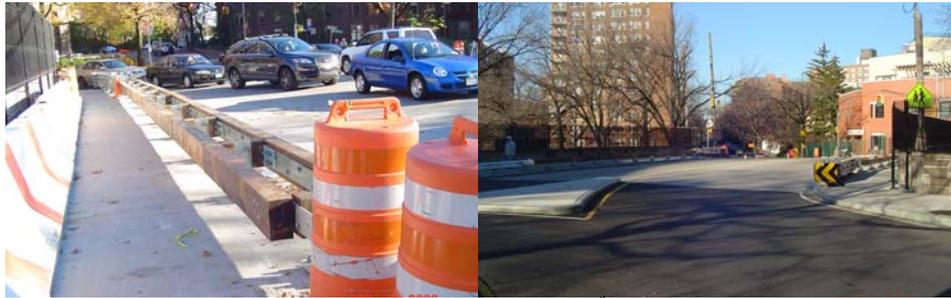
Newly Installed Steel-Backed Timber Guide Rail at West 239<sup>th</sup> Street Bridge. Completed Bridge.
