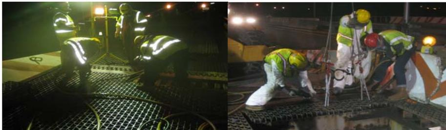
Hand Demolition at Toe Joint.
