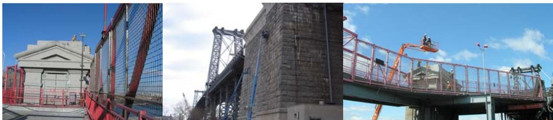
Contract #8 in 2006: North Comfort Station. Manhattan Anchorage Joint Cleaning and Painting. Pointing of Comfort Station Roof.
