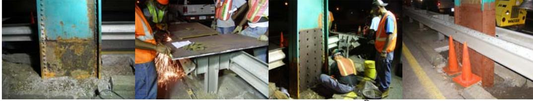
Nighttime Installation of Steel Column Web Reinforcement at the East 111<sup>th</sup> Street Pedestrian Bridge Over the FDR Drive. Completed Repair.
