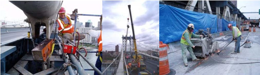
Contract #11 in 2006: Removal of Existing Suspender Rope From Cable Band on Main Span. Sawcutting Lower Roadway Deck on Manhattan Approach Span.
