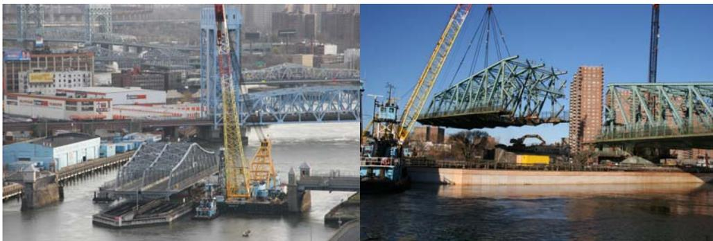
Barge Carrying Crane Passing The Open Madison Avenue Bridge on the Way to Dismantle the Old 145<sup>th</sup> Street Swing Span. Dismantling the Truss.
