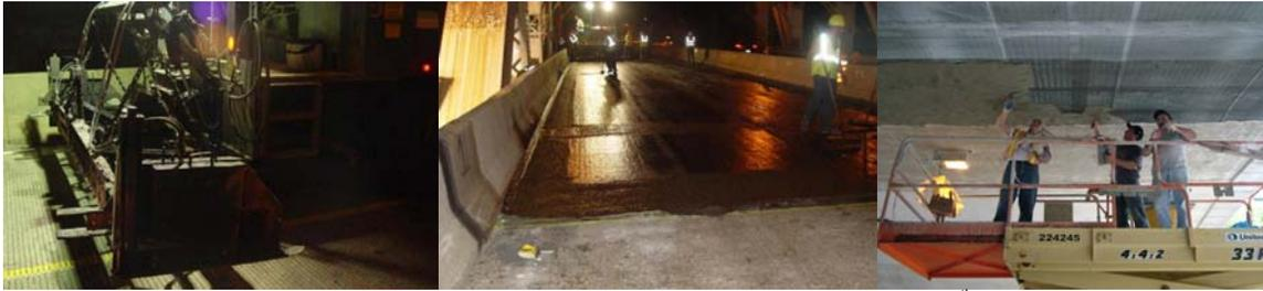
Contract #6 in 2006: Microsurfacing the North Upper Roadway. Repairing the 59<sup>th</sup> Street Overpass.
