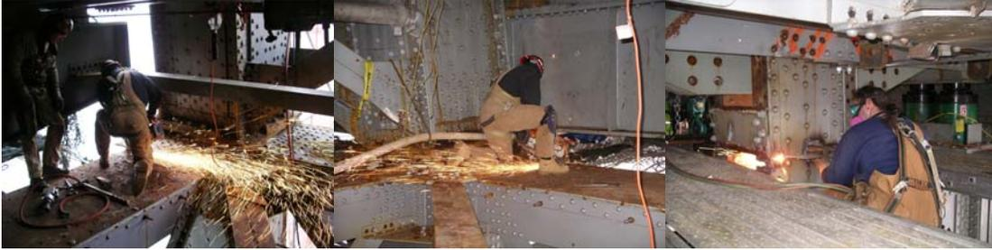
Contract #8 in 2005: Rehabilitation of the Brooklyn Main Tower Steel. Torch Cutting on the Tower.
