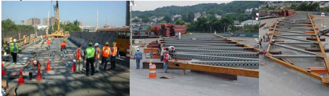
2005: Replacing Span #3. Swing Span Truss Assembly.
