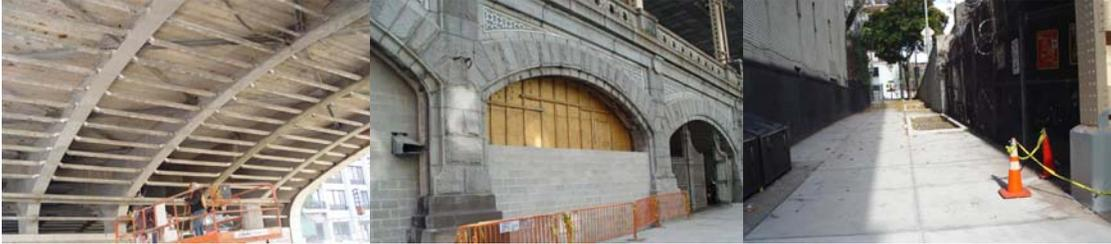
Contract #6 in 2004: Repairing Spalled Concrete at the 59th Street Overpass. Sanitation Arch Infill Work Progressing at 60<sup>th</sup> Street. Repaired Sidewalk Between 61<sup>st</sup> & 62<sup>nd</sup> Streets.
