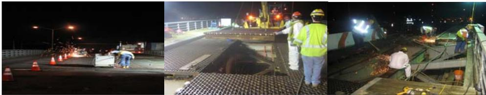
Sawcutting And Removing Deck Panels. Surface Preparation After Panel Removal.
