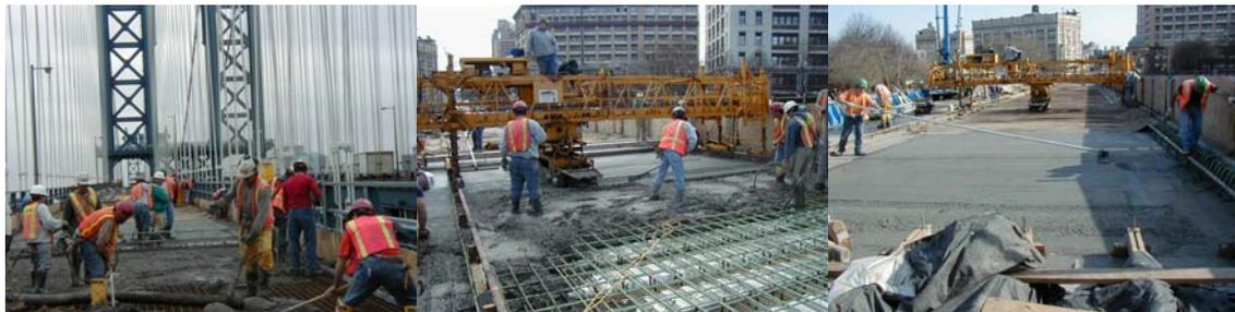
Contract #10 Placing Concrete on the Manhattan Side Span Grid Deck of the North Upper Roadway. Placing and Finishing Concrete on the Grid Deck of the Brooklyn Elevated Structure.
