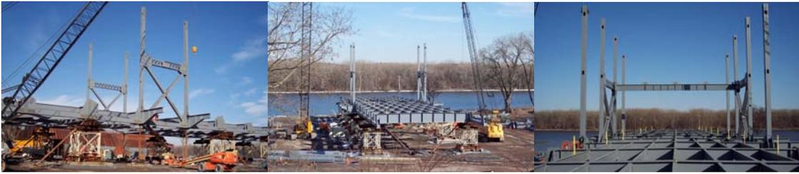
2006: Assembling the New Swing Span in Albany.
