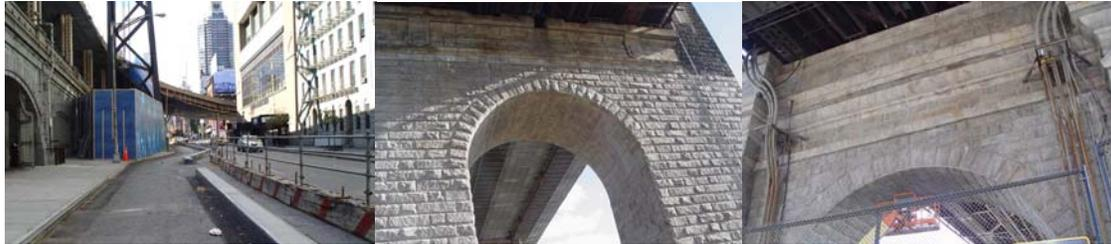
Contract #6 in 2004: Repaired Curb at 60<sup>th</sup> Street. Anchor Pier Granite Cleaning in Progress.
