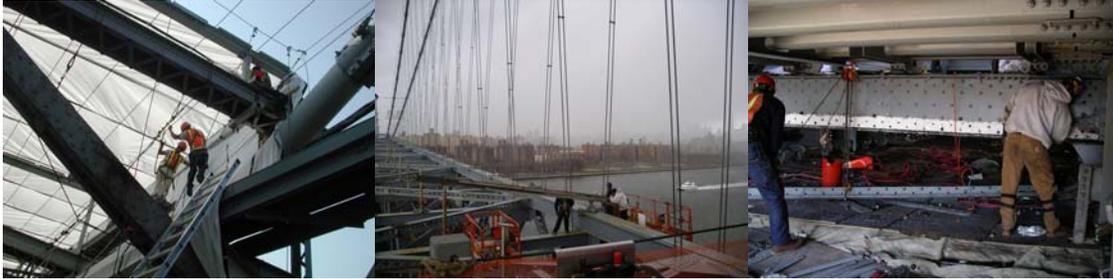
Contract #8 in 2003: North Stiffening Truss Containment Erection and Removal.
