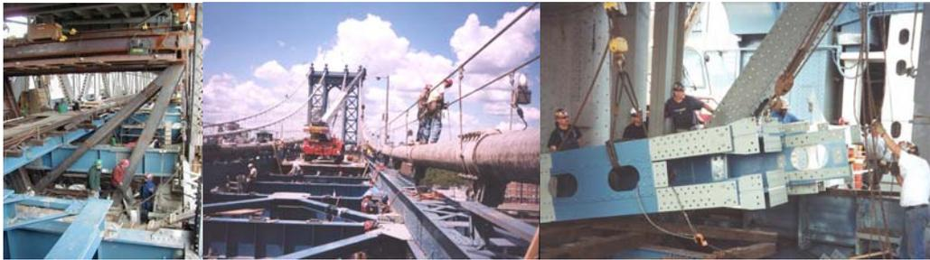
Contract #10 Temporary Truss Jacking Frame Used in the Work to Replace the Existing Truss Bearings.
