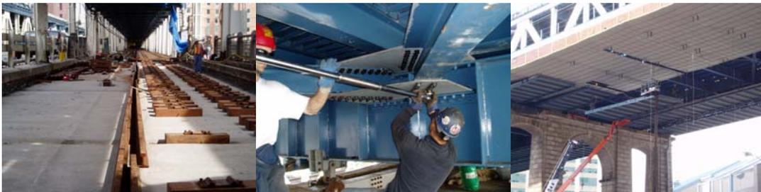
Contract #10 Installation of New Ties for the North Subway Track. Torquing the Bolts for the Installation of the Upper Laterals for the Truss Stiffening System. Installation of a Permanent Maintenance Platform Under the Bridge on the Brooklyn Approach Span.
