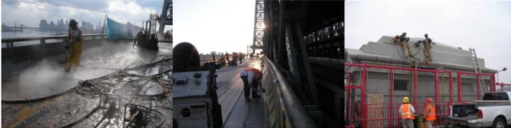
Contract #8 in 2006: Water Blasting. Curb Angle Cleanup and Tack Coat. Core Drilling The Brooklyn North Comfort Station.
