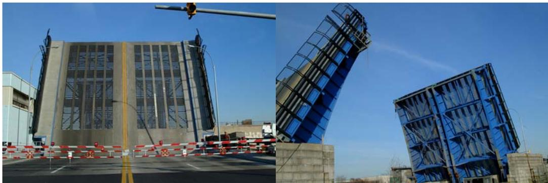
Bridge Opening With New Machinery And New Warning And Safety Gates.
