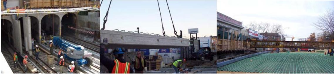
Installing Pier Walls for the 17<sup>th</sup> Avenue Bridge. Installing Precast Deck Panels.
