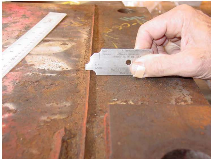
Figure 10 Base Plate/Tie Beam Fillet Weld Size Measurement.
