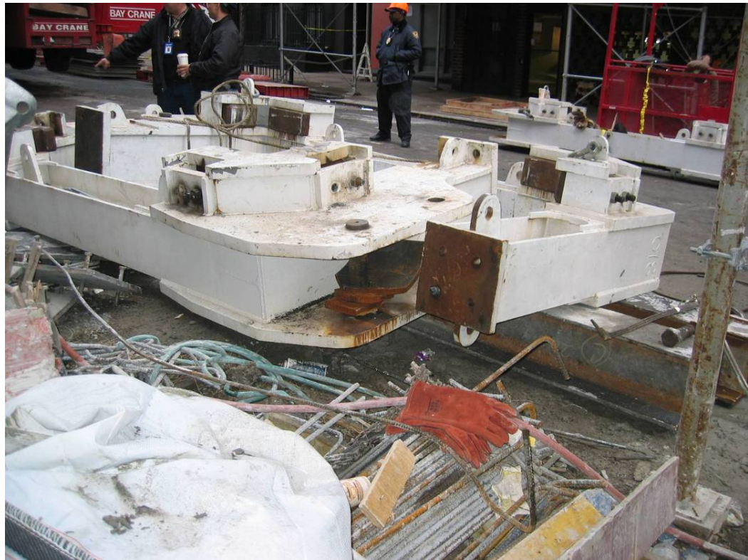
9 th Floor Collar Assembly
