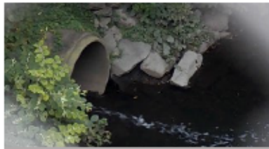
An outfall belonging to Yonkers at Nereid Avenue, discharging during dry weather.
