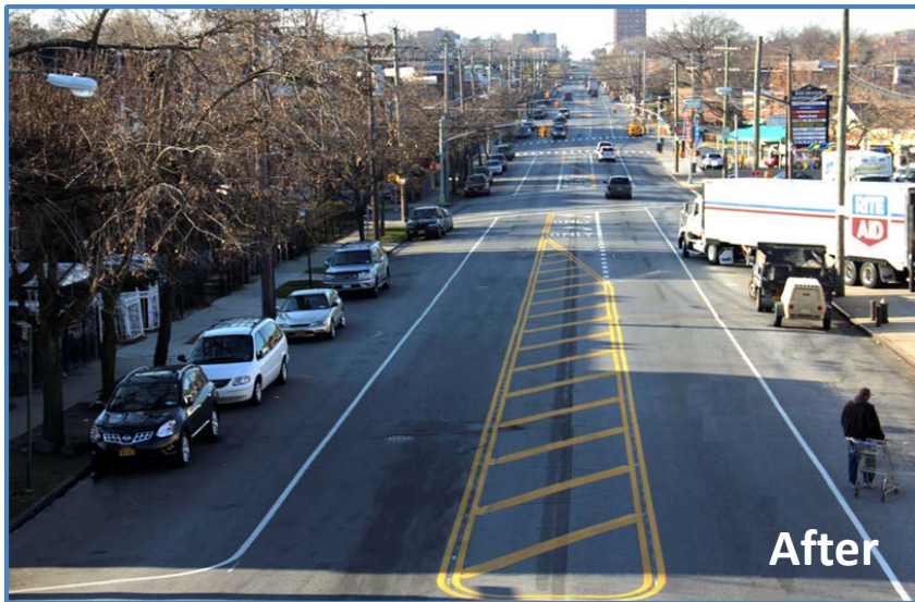
233 rd St at Baychester Ave facing west
