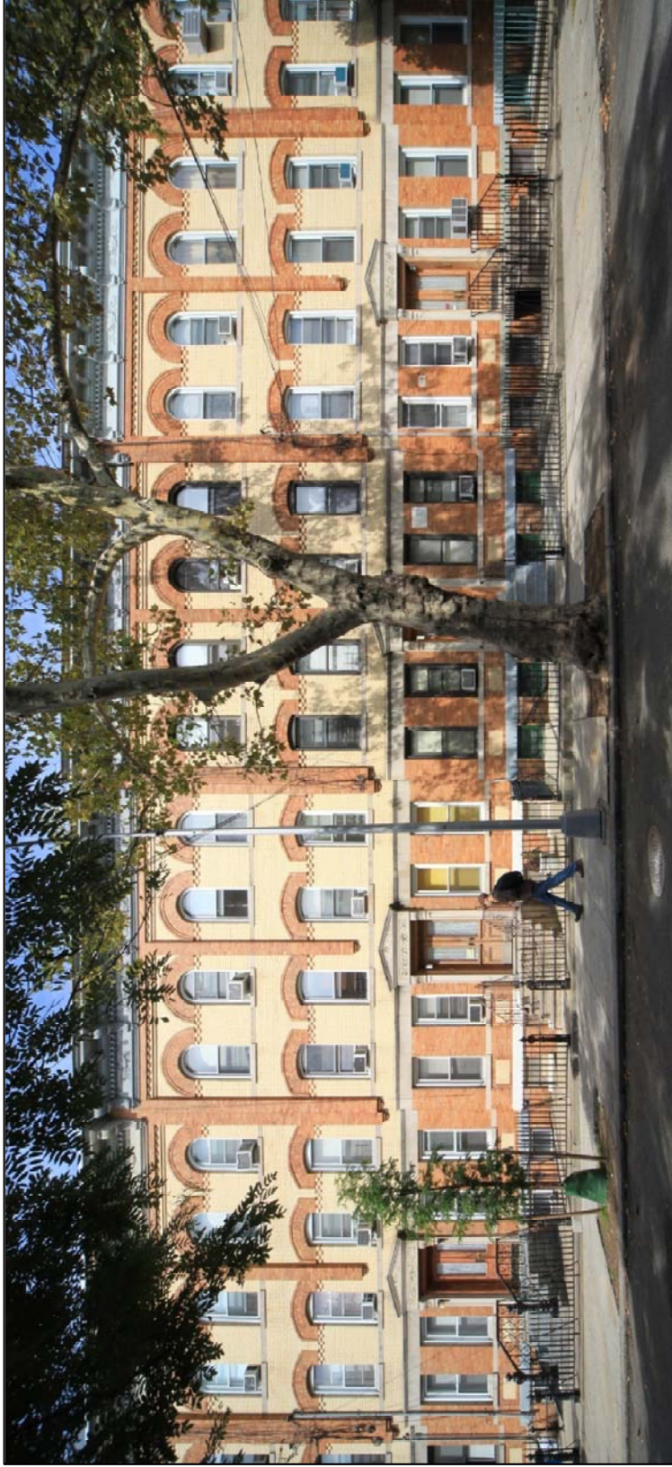
Figure 12 Northwest side of Palmetto Street Photo: Christopher D. Brazeel, 2009
