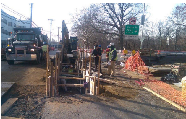
Southeast Queens sewer build out.
