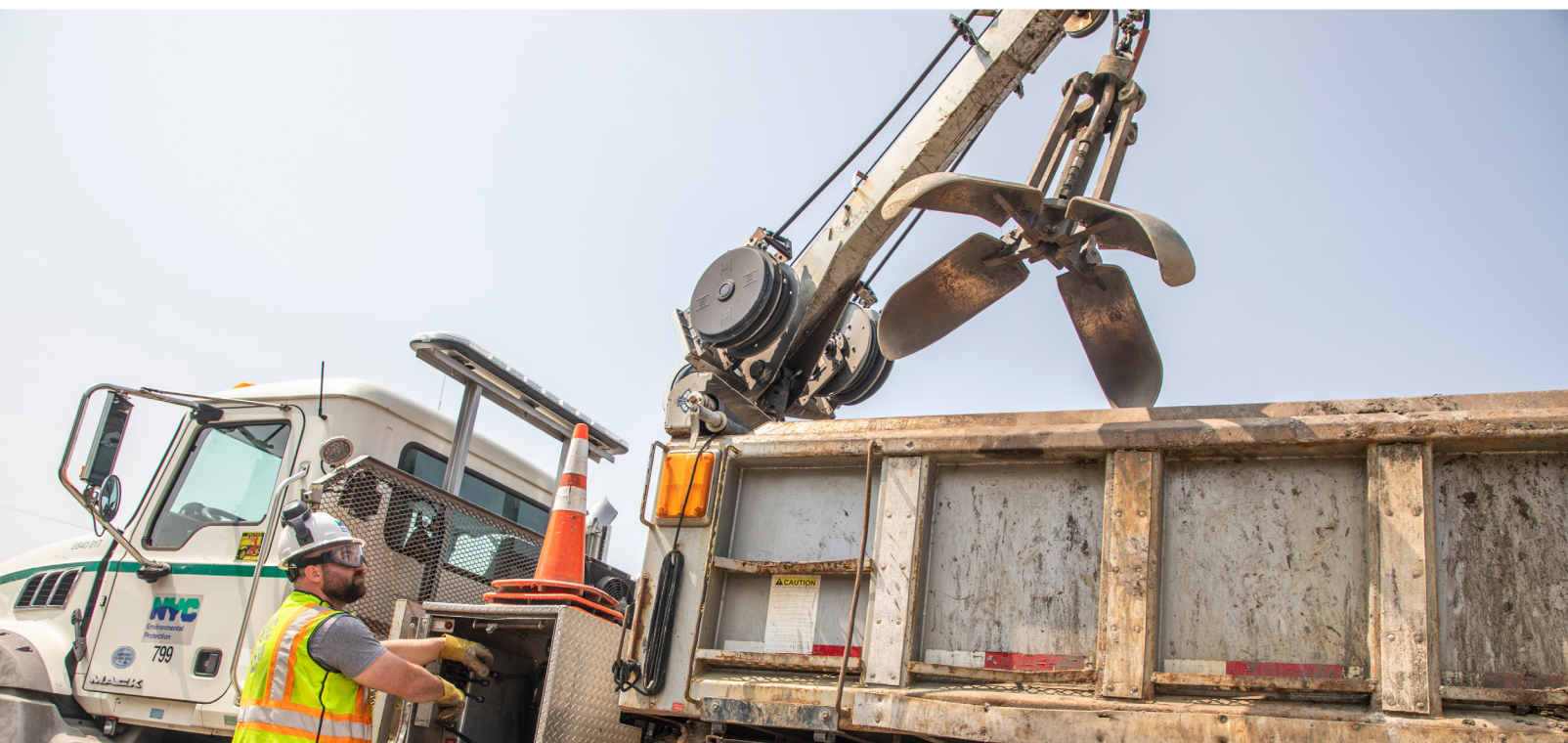
Catch Basin Cleaning Mania Competition.
