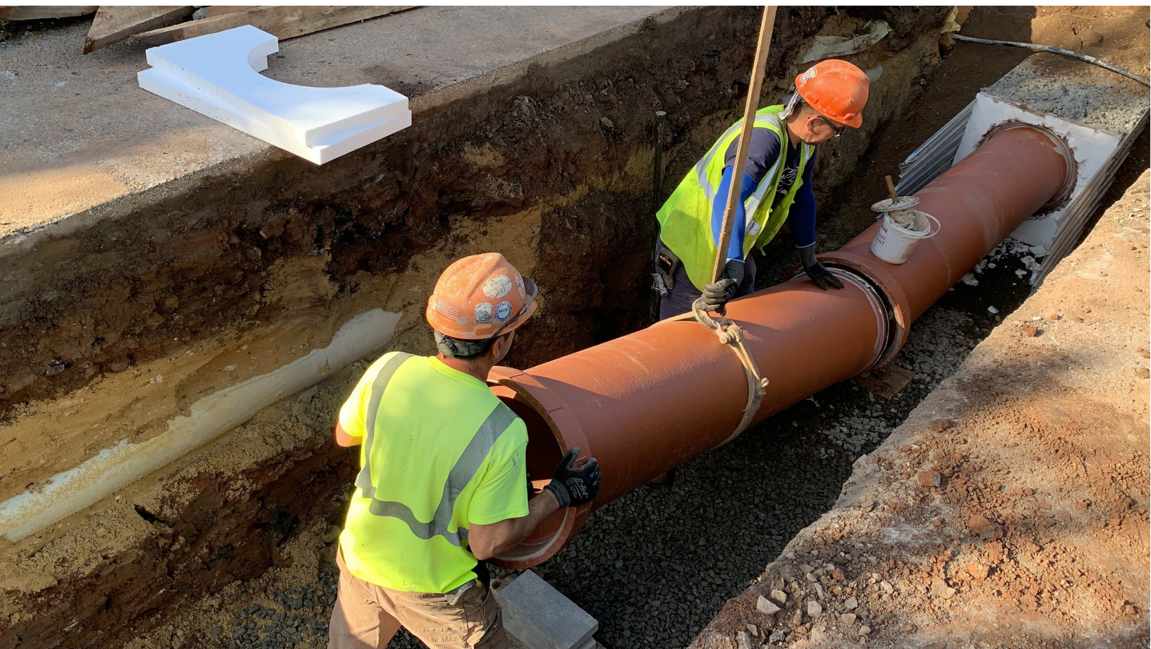
Installation of New Catch Basins for Willowbrook/Westerleigh.
