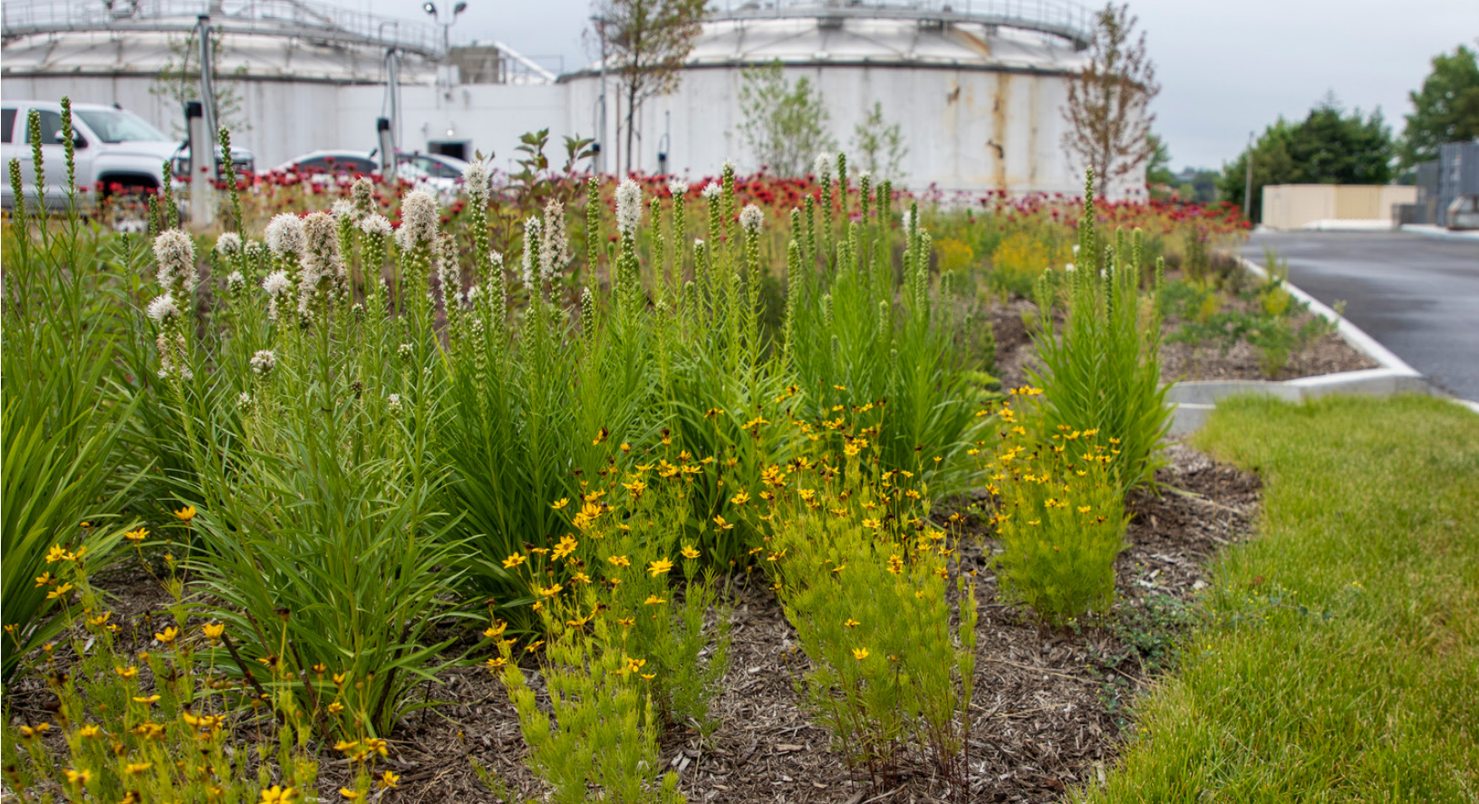
Tallman Island landscaping and green infrastructure for storm water management.
