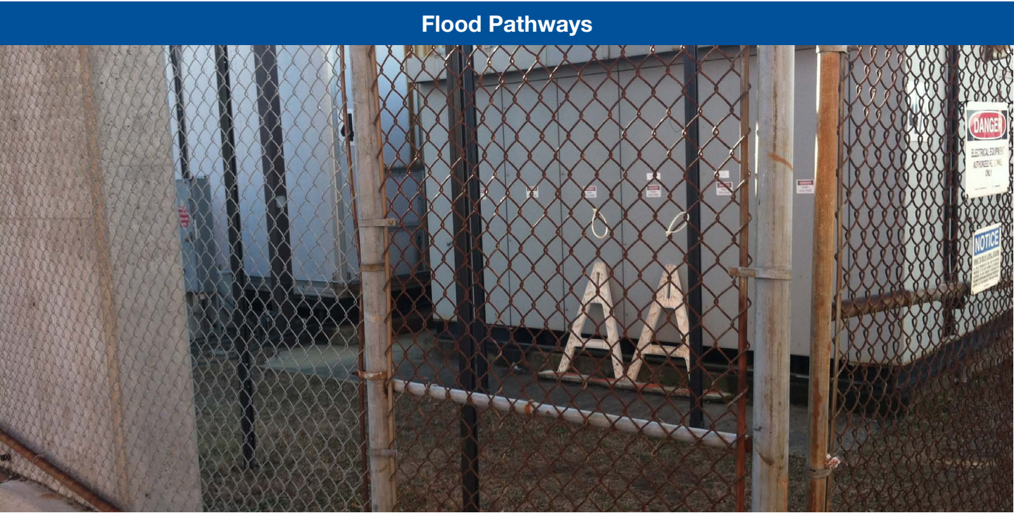
The Unit Substation adjacent to the Return Sludge Pump Station #3 would be flooded at grade level during the critical flood event.
