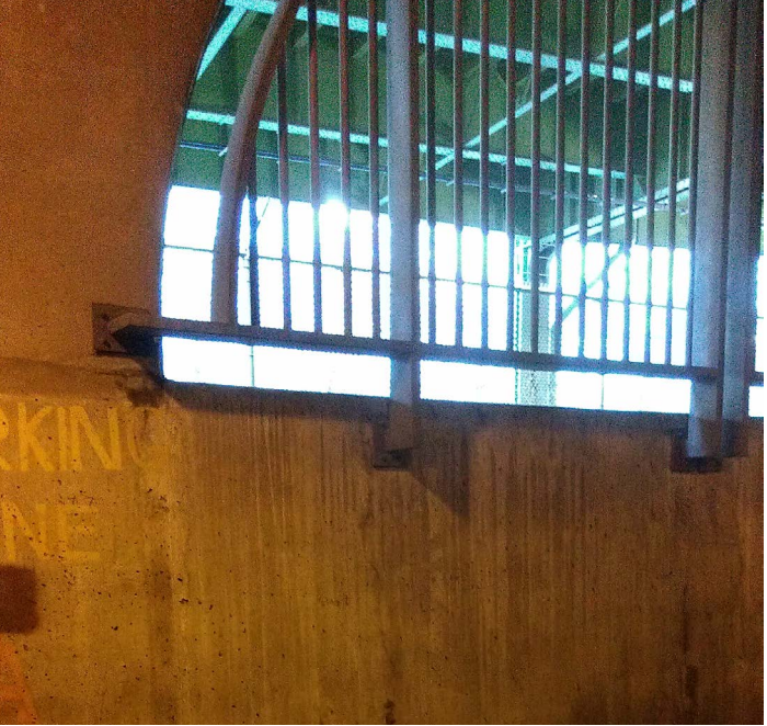
Arched windows around the perimeter of the ground level (EL 5) are considered pathways for flooding.
