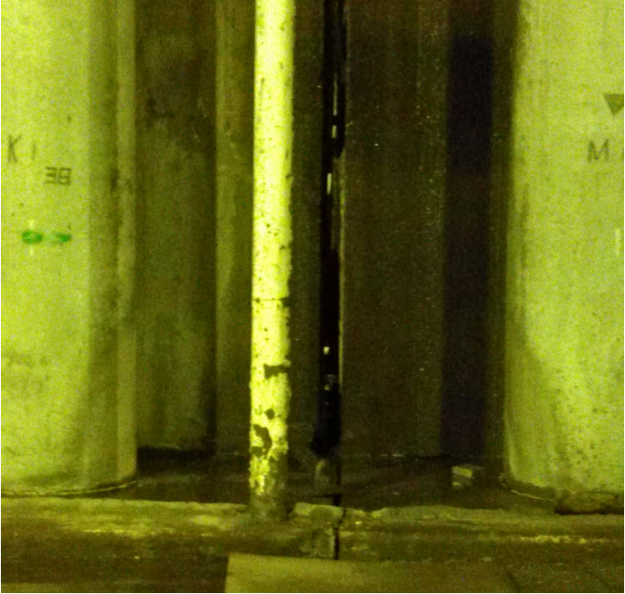
Expansion joints are flood pathways as experienced during Hurricane Sandy.
