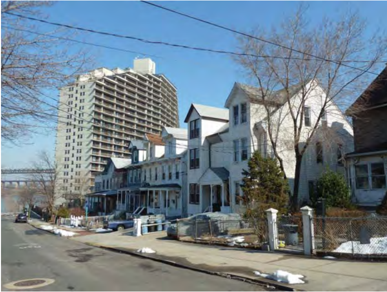
9. Northeast view on 9th Street between 26th and 27th Avenues
