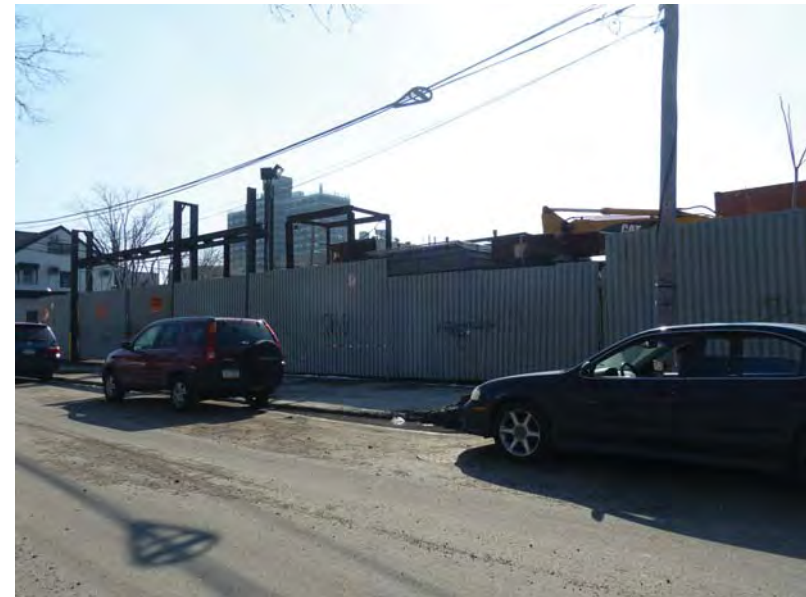
24. South view from 26th Avenue between 2nd and 3rd Streets
