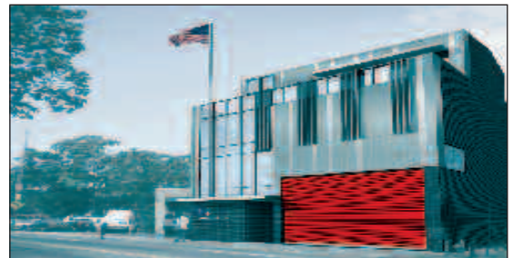
Bronx EMS Station 27 serves Riverdale and Kingsbridge.
