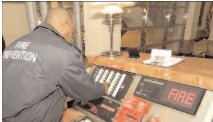
Bureau of Fire Prevention Inspector examines and tests fire alarm warning system in high-rise office building.
