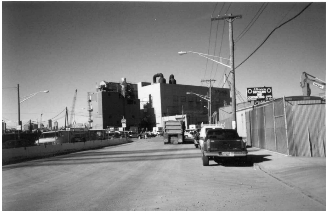
Figure 20.7-1 : View toward site from Green Street.
