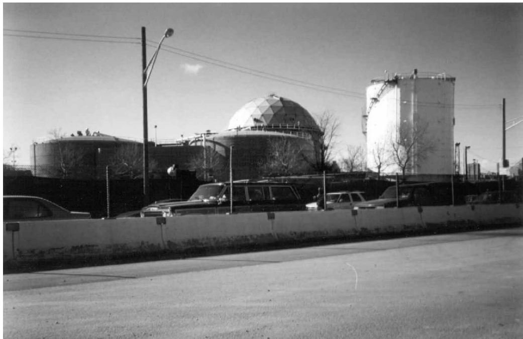
Figure 20.7-2: Newtown Creek WPCP, looking west along Green Street.
