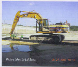
Excavator parked in a spill containment berm in the JPR basin.
