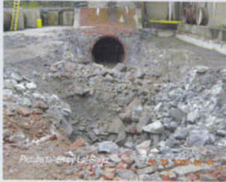
Excavation is progress.
