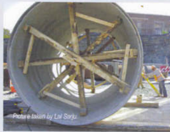
A 20-foot section of the pipe being delivered to the Jerome Park Reservoir site.
