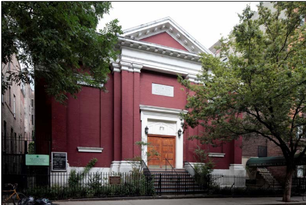
Evangelical Lutheran Church of St. Mark 323 East 6 th Street
