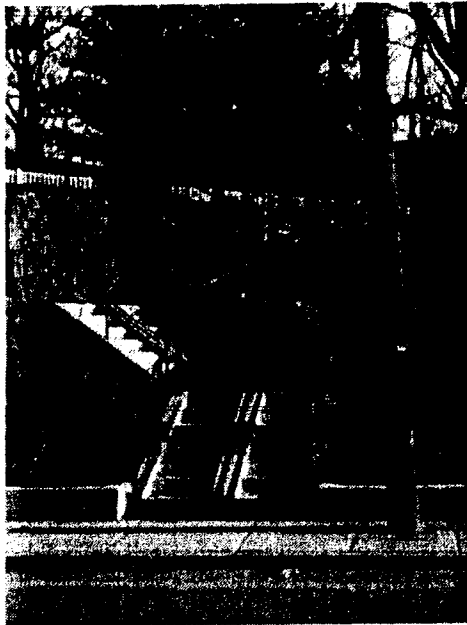
Figure 1: Example of bicycle stair trough
