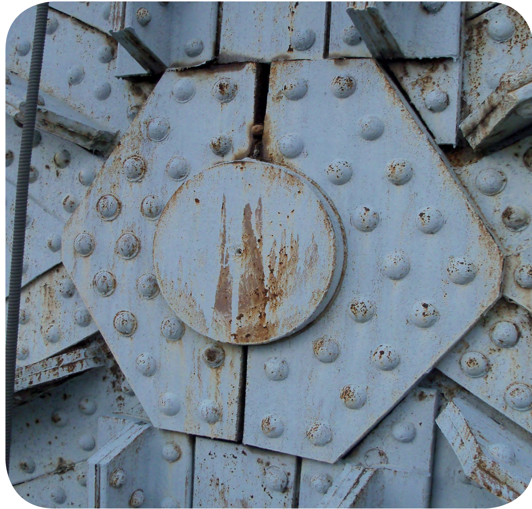
Close-Up Photo of Decorative Steel at Arch Top
