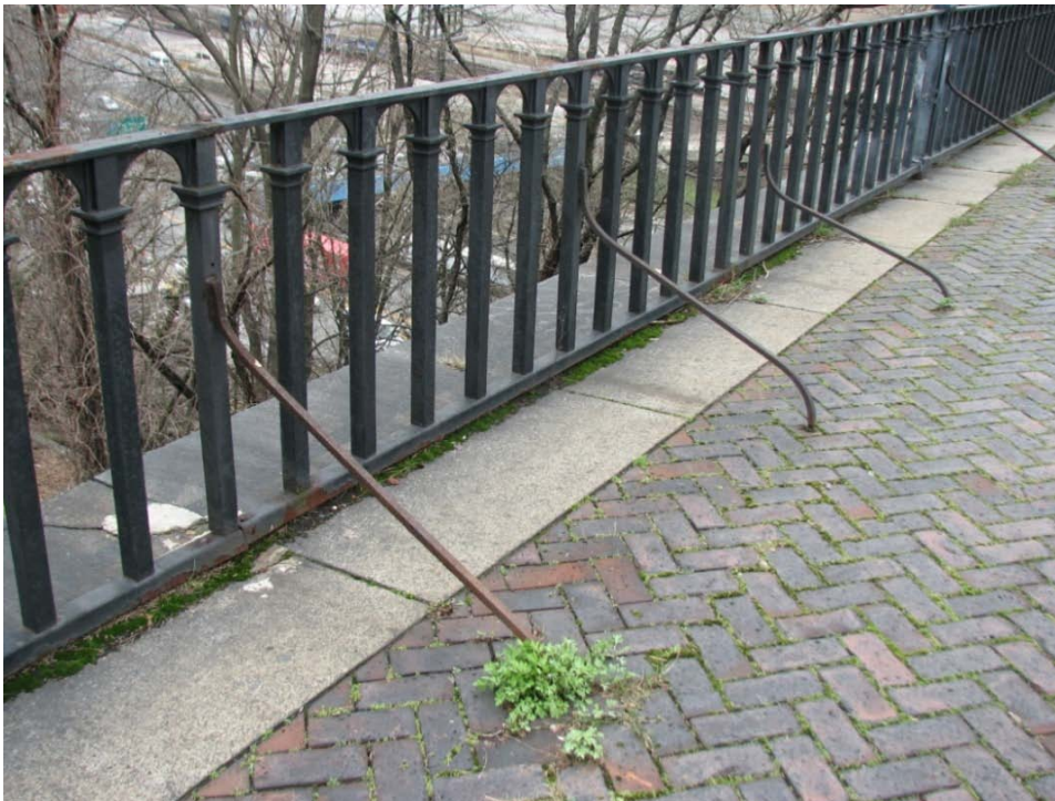
FIGURE 26. View of non-historic metal bracing at the 1864 railings.
