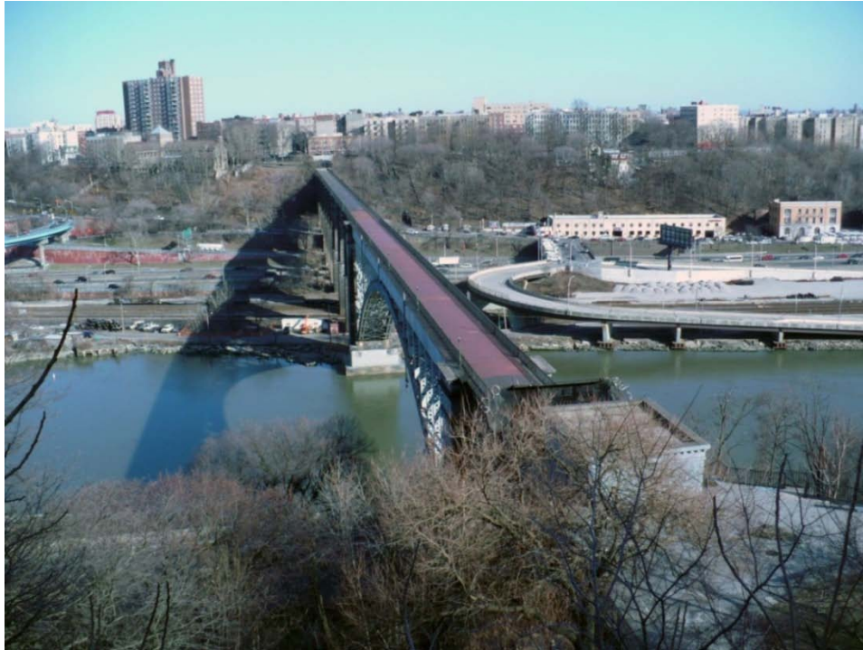
FIGURE 7. Aerial view of the walkway looking toward The Bronx with the Manhattan gatehouse and plaza in the foreground
