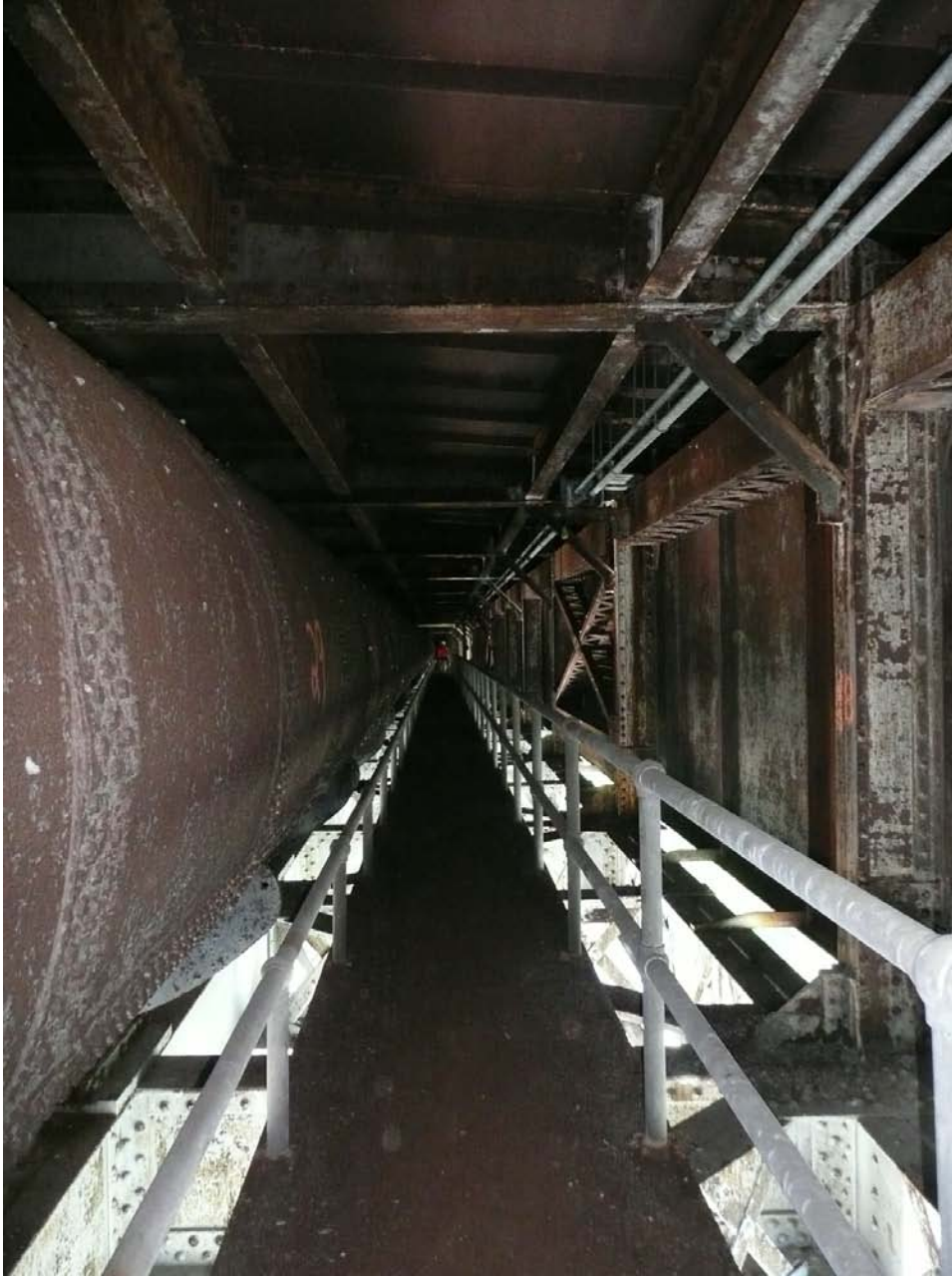
FIGURE37. View of the aqueduct and walkway at the metal arch
