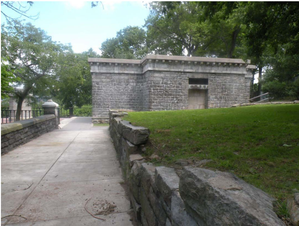
FIGURE 18. View of the south elevation of the Bronx gatehouse and surrounding plaza, including the foundation remnants of the office building
