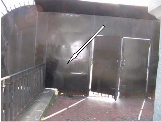
Photo LCM #7: Black over silver paint present on west abutment security gate. This paint is also present on the east abutment security gate.
