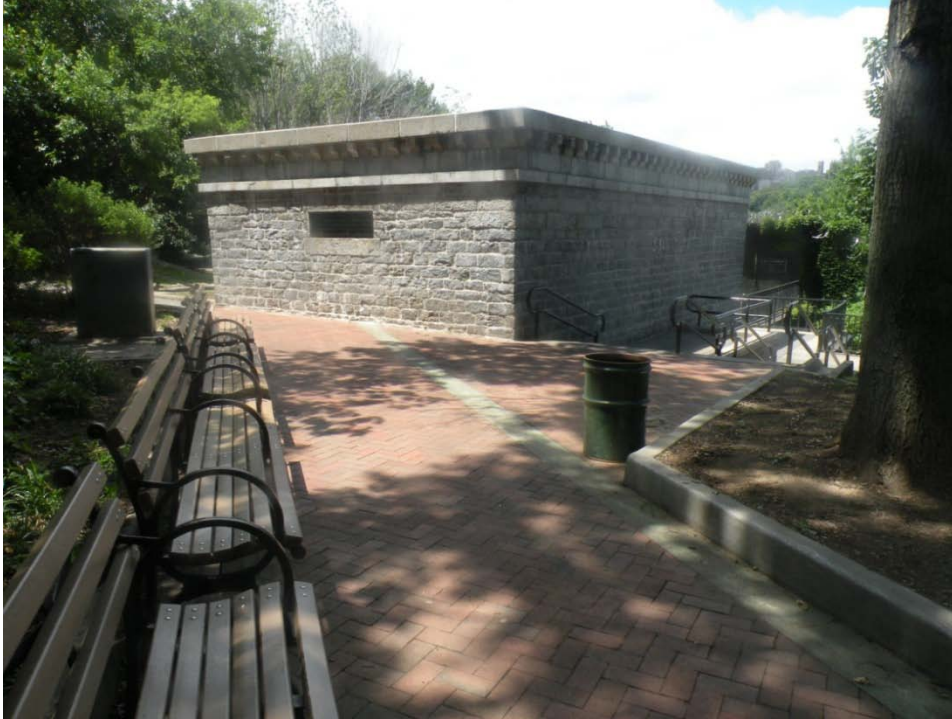
FIGURE 17. View of the east and north elevations of the Bronx gatehouse and surrounding plaza
