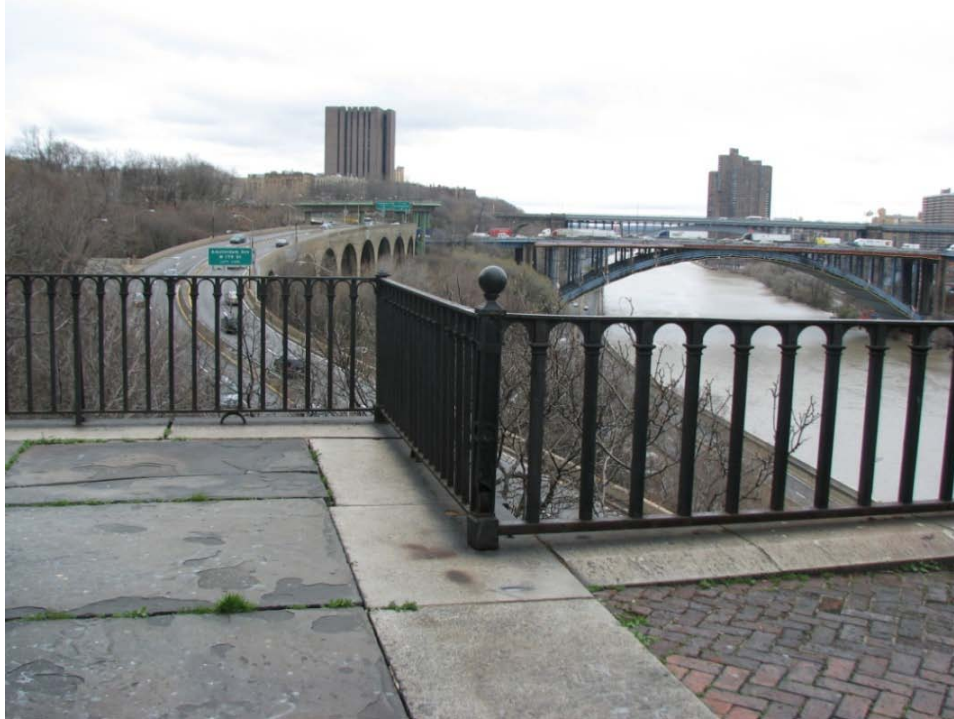
FIGURE 19. Detail view of the 1850 railing (left and center) and 1864 railing (right) at the Manhattan gatehouse plaza. Note the variance in picket spacing and formation of the arches.
