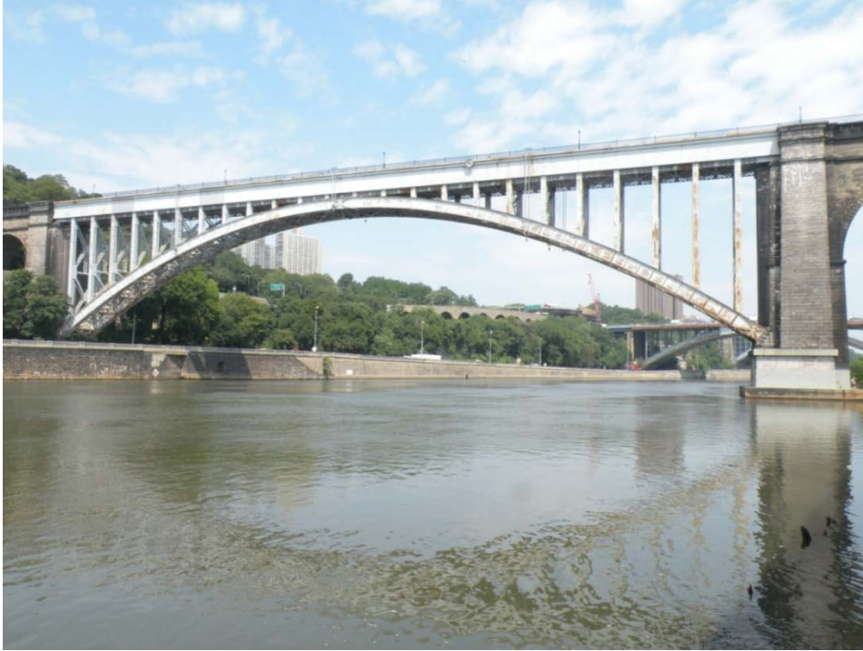
FIGURE 5. View of the south elevation of the metal arch
