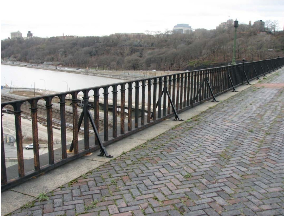
FIGURE 25. View of historic metal bracing at the 1864 railings.
