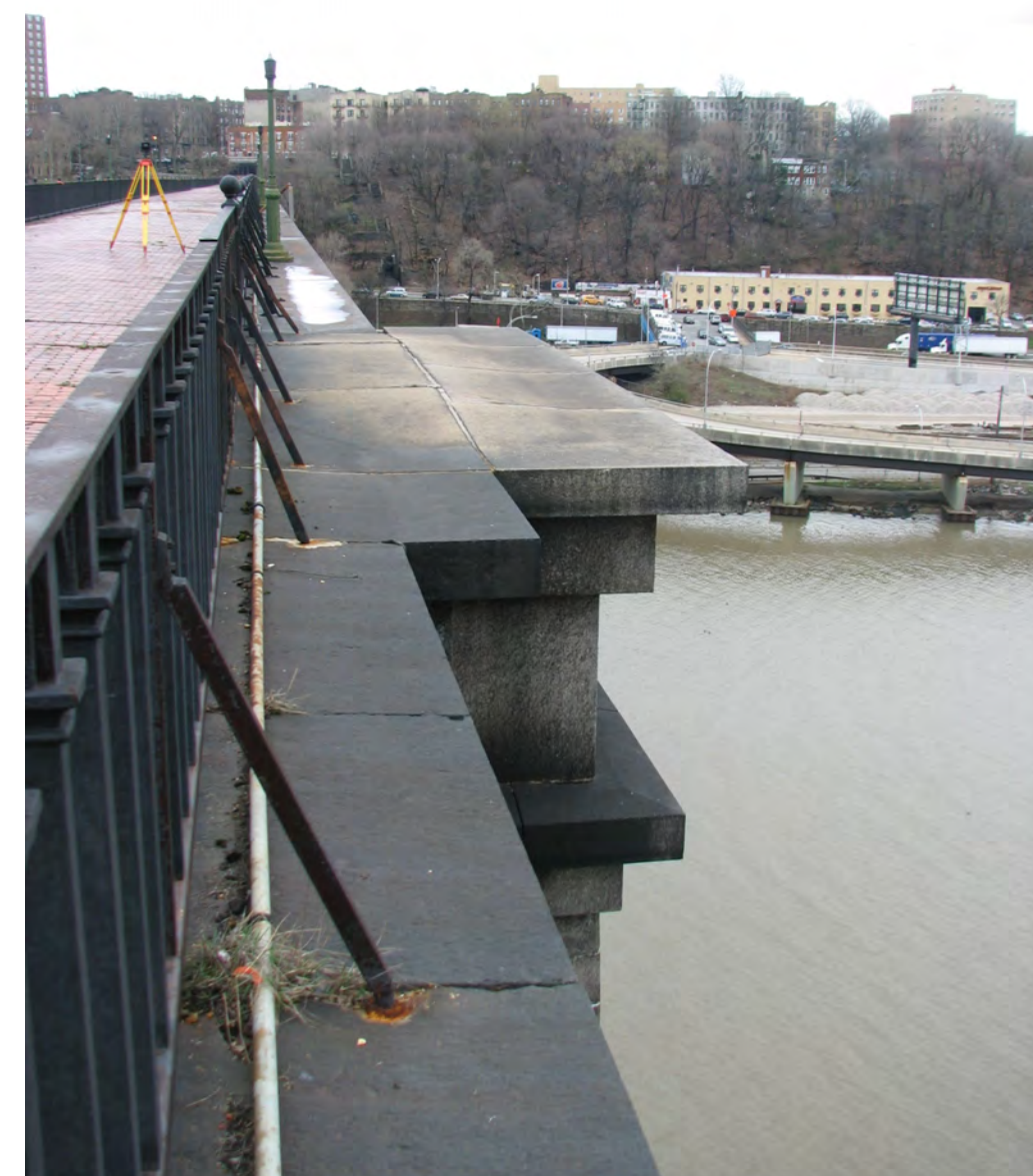
EXISTING CONDUIT AT GRANITE COPING
