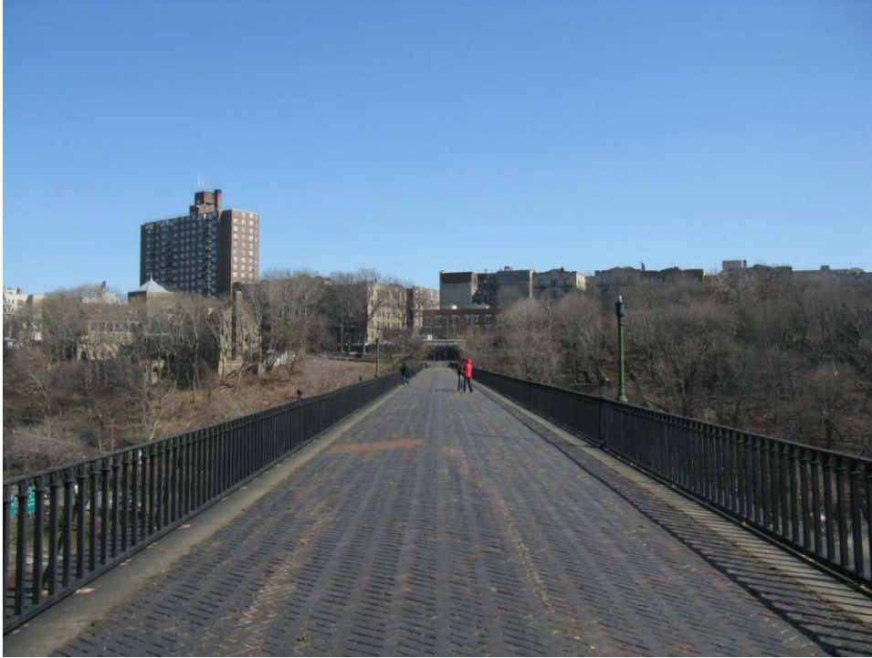
FIGURE 13. View of the walkway looking toward The Bronx
