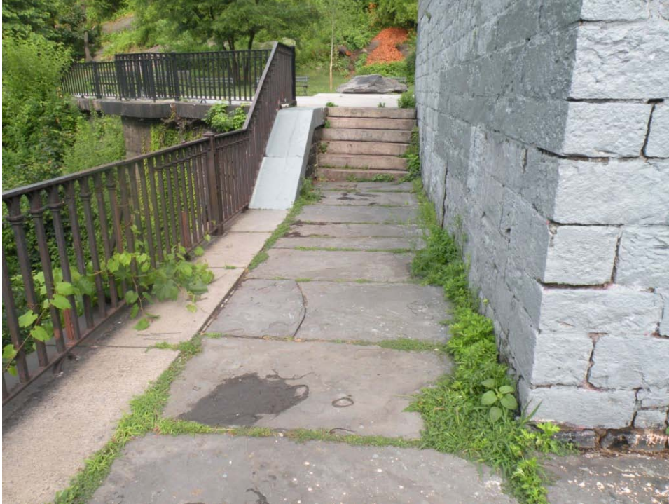
FIGURE 27. View of bluestone pavers and granite steps at south side of Manhattan gatehouse
