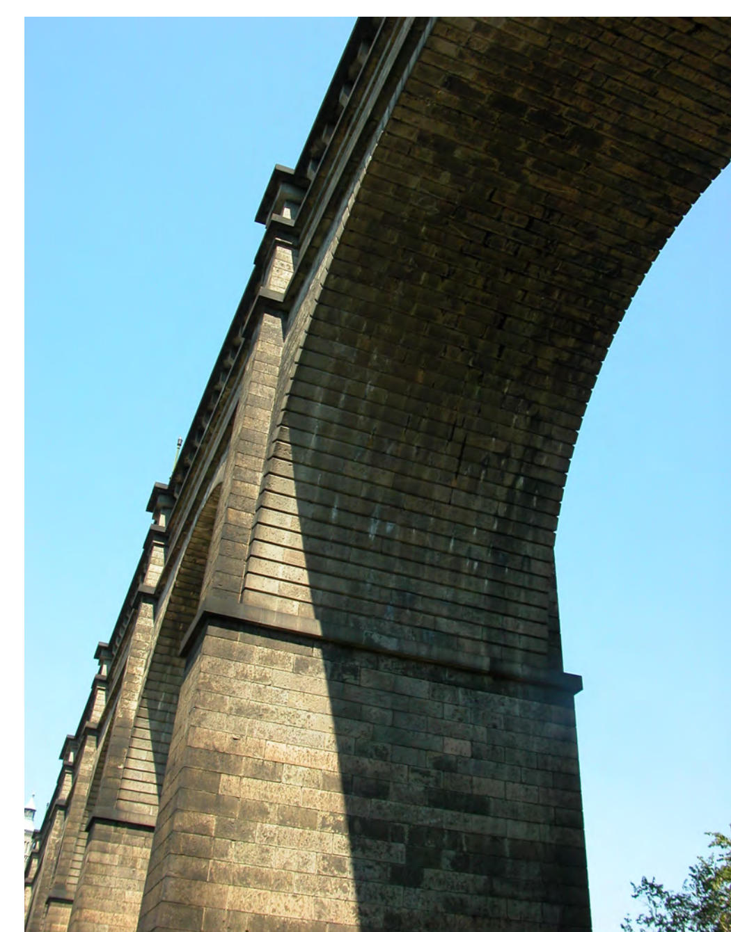
UNDERSIDE OF TYPICAL MASONRY ARCH
