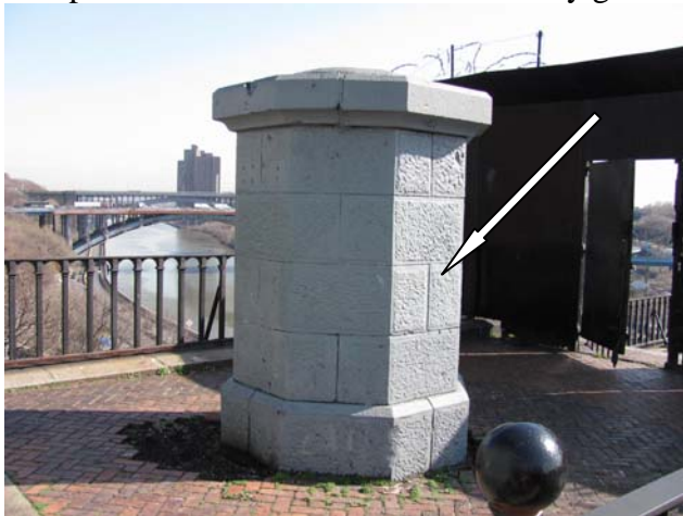
Photo LCM #8: Gray over brown paint present on masonry tower located between the security gate and the Westgate house.
