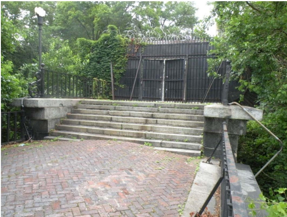
FIGURE 14. View of the Bronx side steps and security gate as seen from the walkway
