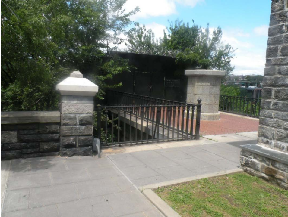
FIGURE 15. View of the Bronx vent, vent plaza and security gate
