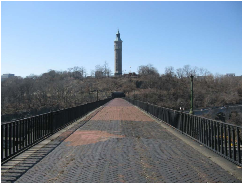
FIGURE 12. View of the walkway looking toward Manhattan
