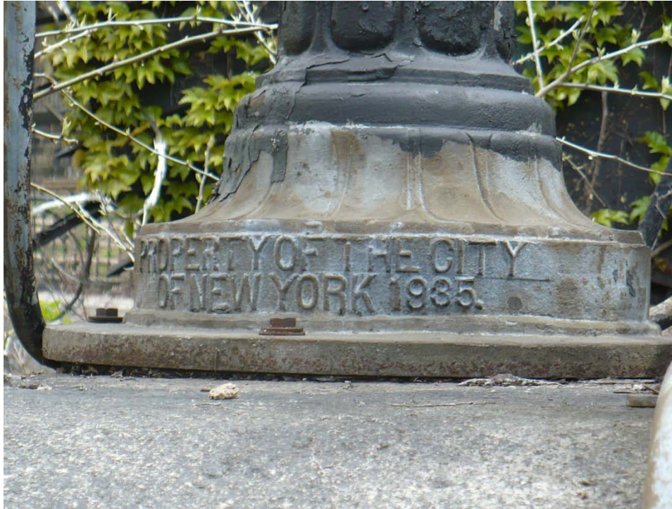
FIGURE 30. Close up view of the identification stamp found on the existing light poles.
