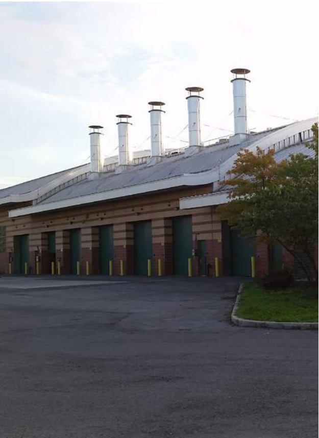
Paerdegat Basin CSO facility
