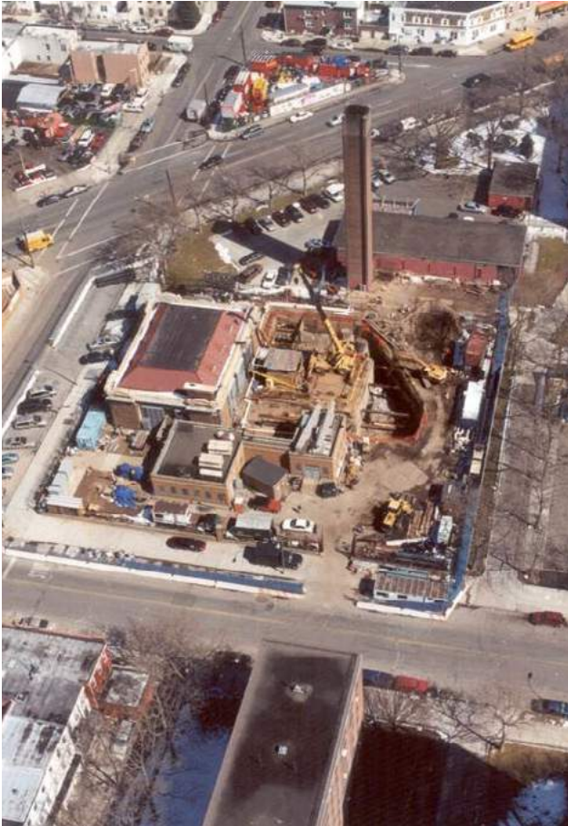
Construction at Avenue V pump station
