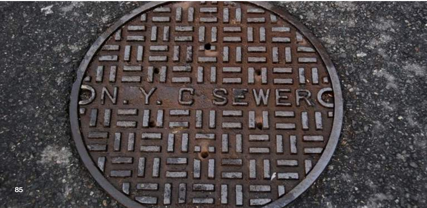
NYC sewer manhole
