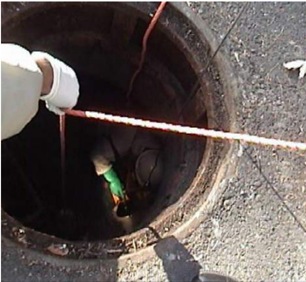
DEP staff begins sewer investigation
