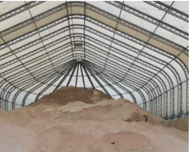
DSNY salt shed
