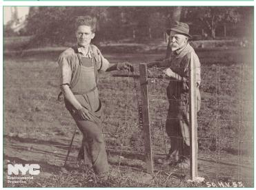
Employees of the Knox Fence Company construct wire fencing at Hillview Reservoir in Yonkers. First the line wires were strung, then vertical stays were fastened using a special tool that held the stay to the line wire and clamped a wire lock around them. The board with a small level attached to it rode on the wires to maintain the spacing of the line wires and plumb the stays. October 22, 1915. For more photos from DEP's archives, visit the <u>Out of the Archives album</u> on our Flickr page.
