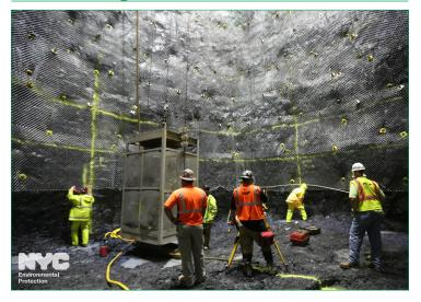
DEP's work on the Delaware Aqueduct Bypass Tunnel is continuing safely and according to schedule. Workers are currently mining two shafts on either side of the Hudson River to gain access to the subsurface, which will allow tunneling to begin next year. Shaft 5B in Newburgh is currently built to a depth of 740 feet, while Shaft 6B in Wappinger is at roughly 580. They will be 900 and 700 feet deep respectively.
