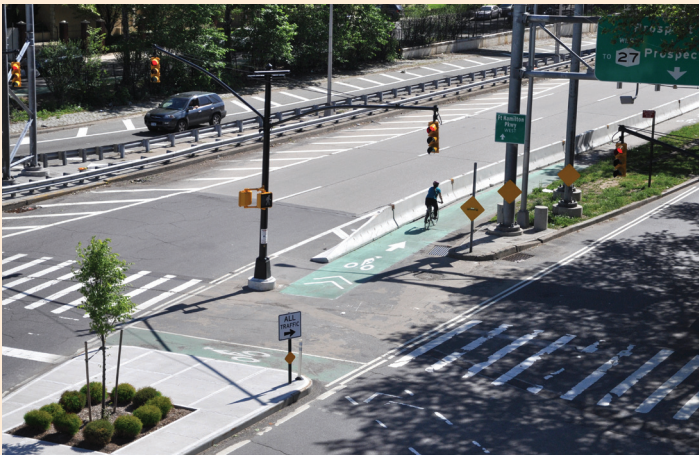
A bicycle lane was added on Fort Hamilton Parkway to expand the bicycle network and provide connections to existing bicycle lanes to the west of Prospect Park.
