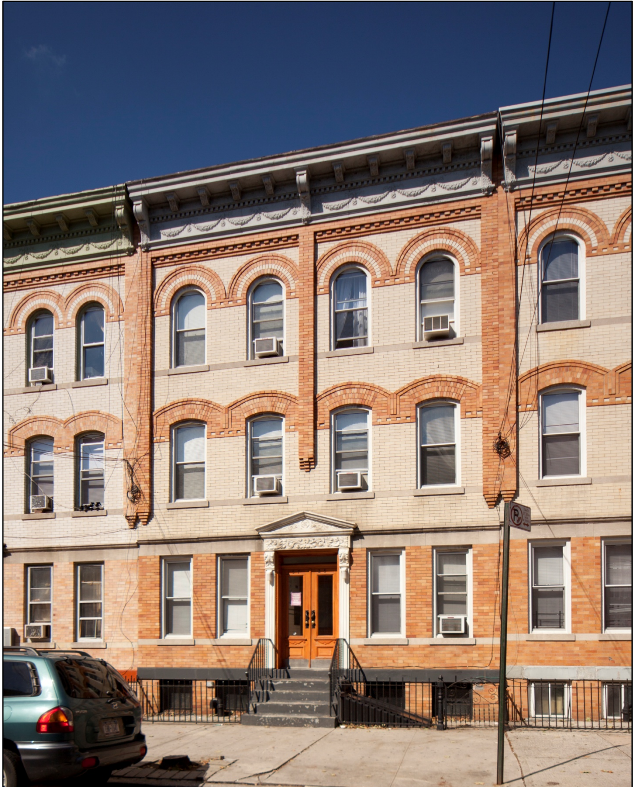
Figure 22: Intact upper stories on Catalpa Avenue. Photo: Christopher D. Brazee, 2010.
