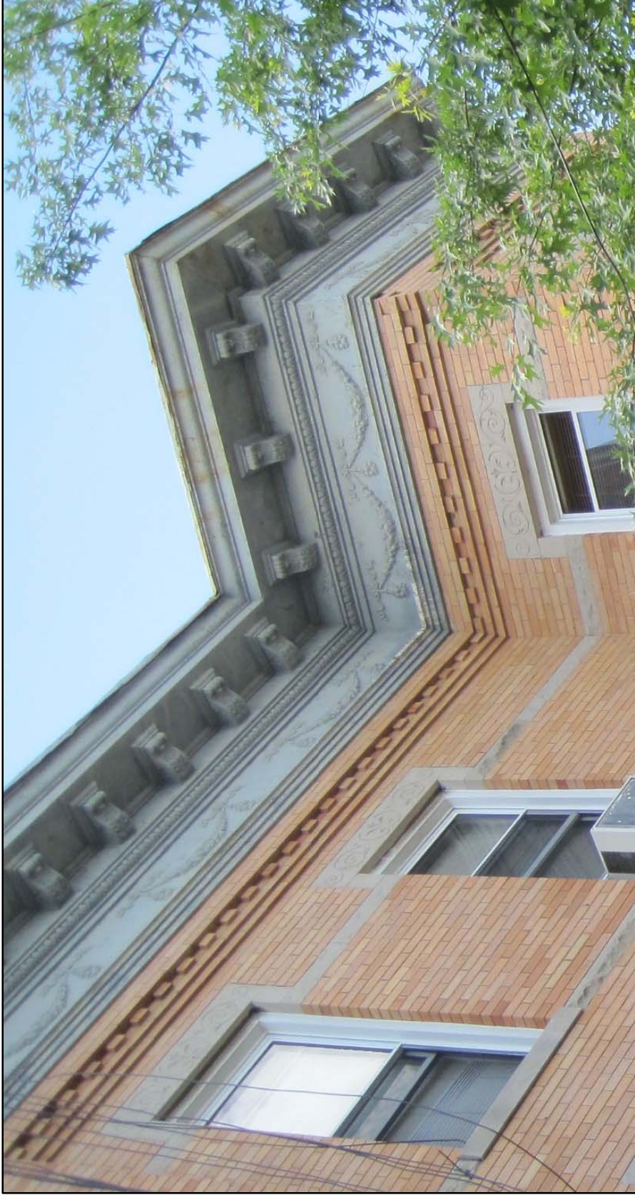
Figure 8: 862 Woodward Avenue, detail of pressed-metal cornice with swags and garlands. Photo: Tara Harrison, 2010.
