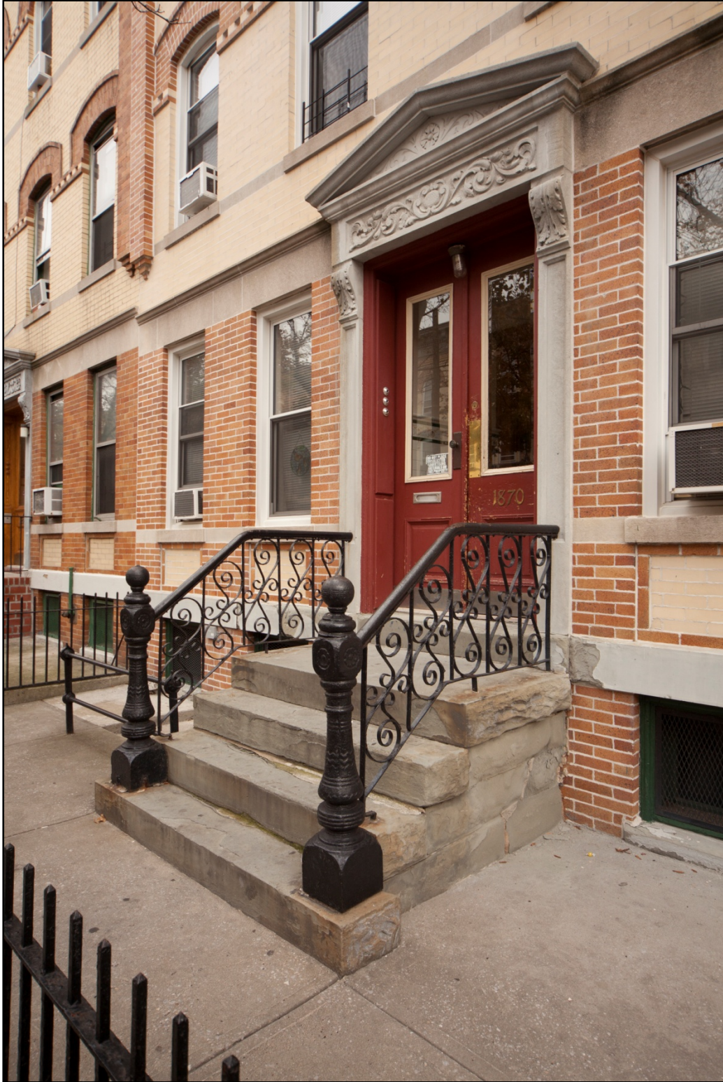
Figure 6: 1870 Putnam Avenue, detail of bluestone stoop with historic ironwork. Photo: Olivia Klose, 2010.
