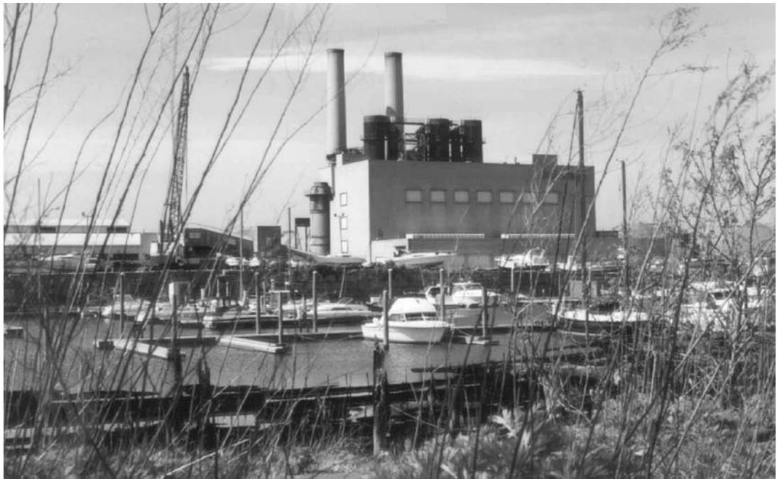
Figure 5.7-1: View northward from Bay 43rd Street. (Photo 2000)
