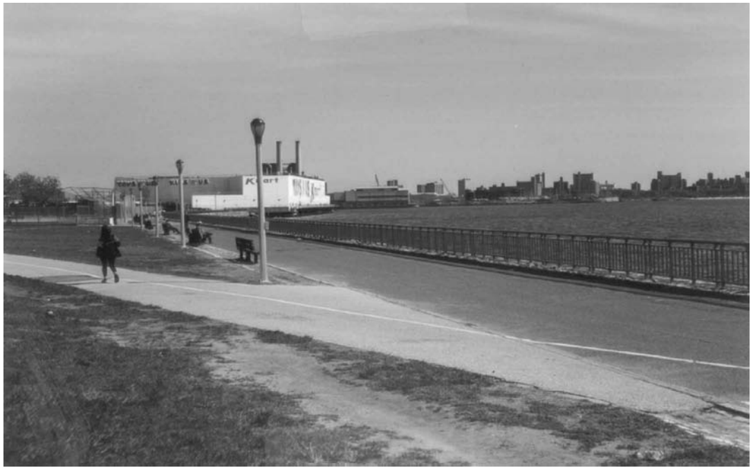
Figure 5.7-3: MTS as viewed from the Shore Park at approximately 19th Avenue. (Photo 2000)
