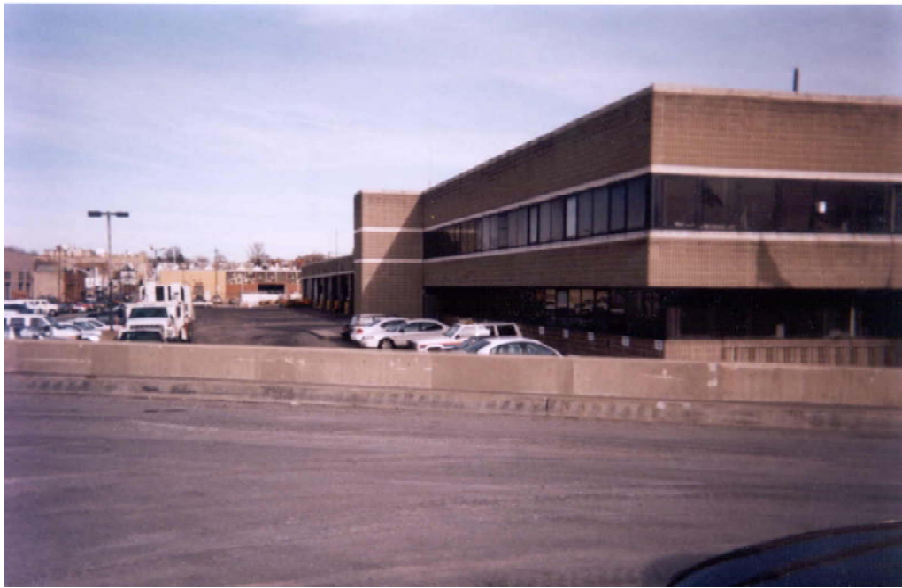
Figure 11.7-3 : View north from the site at 31st Avenue.
