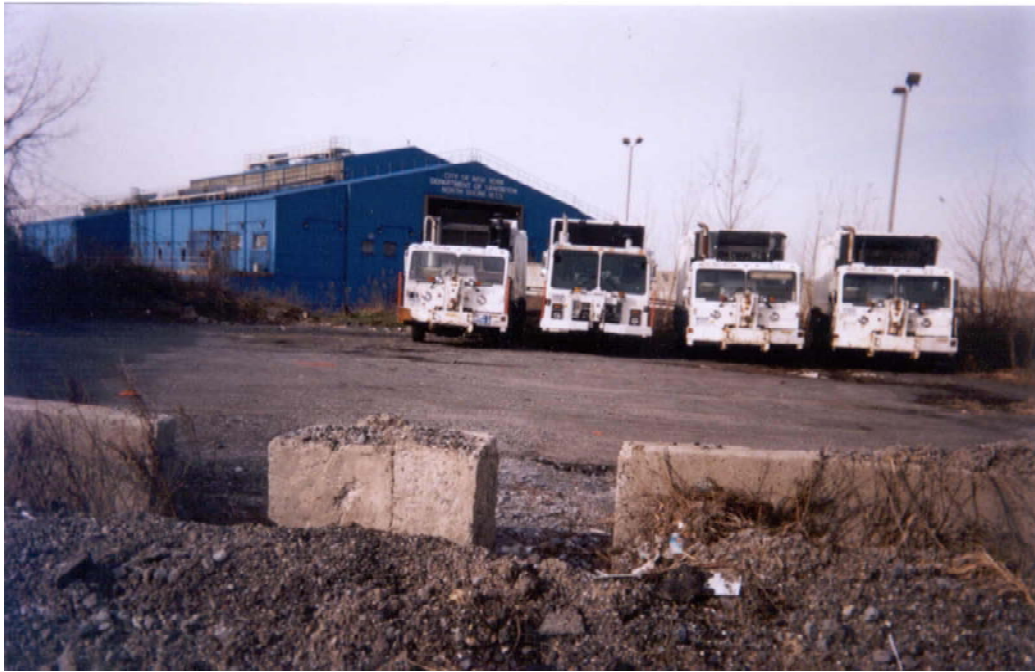
Figure 11.7-1 : View of MTS from 31st Avenue.
