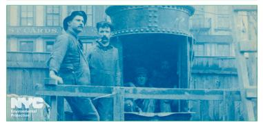
A Mattson compressed air lock with three men inside was photographed back on October 20, 1911. The equipment was used during the sinking of a City Water Tunnel No. 1 shaft in the East Village. Caissons were constructed to pass through up to 100 feet of water-bearing material overlying the bedrock, and the air lock enabled safe passage for workers between areas of differing air pressure.
