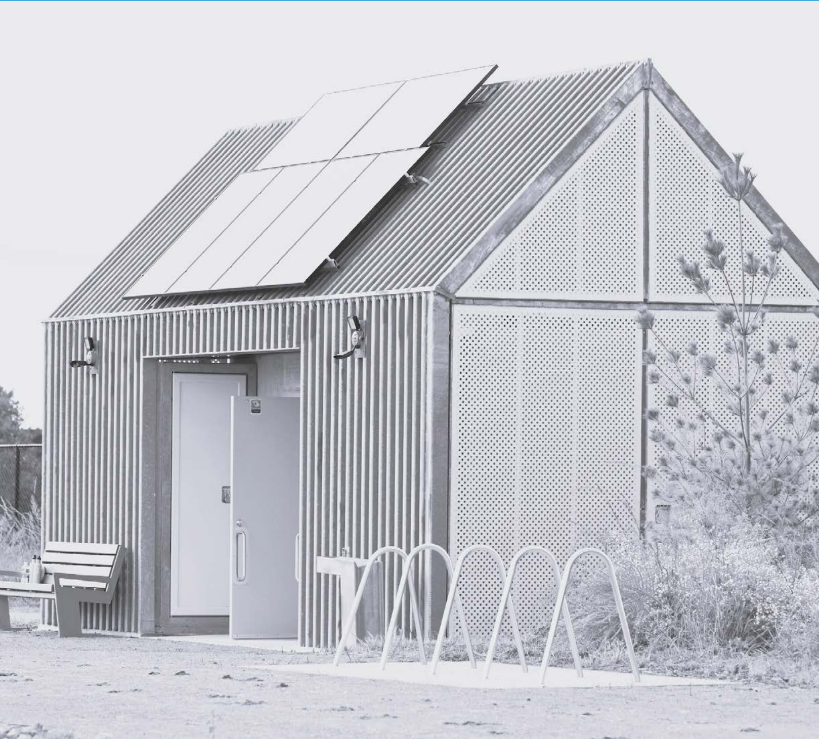
Public Restroom Building Exterior, Freshkills Park
