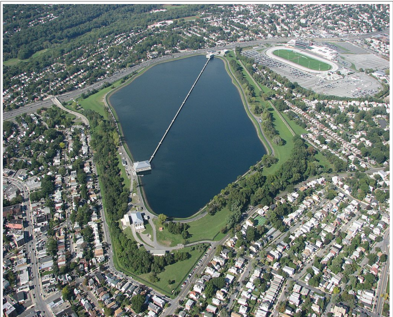
Figure 3.33. Hillview Reservoir aerial view of dividing wall. Photo by DEP Police.
