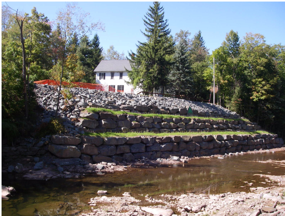
Figure 4.15 Schoharie Avenue streambank stabilization following construction.
