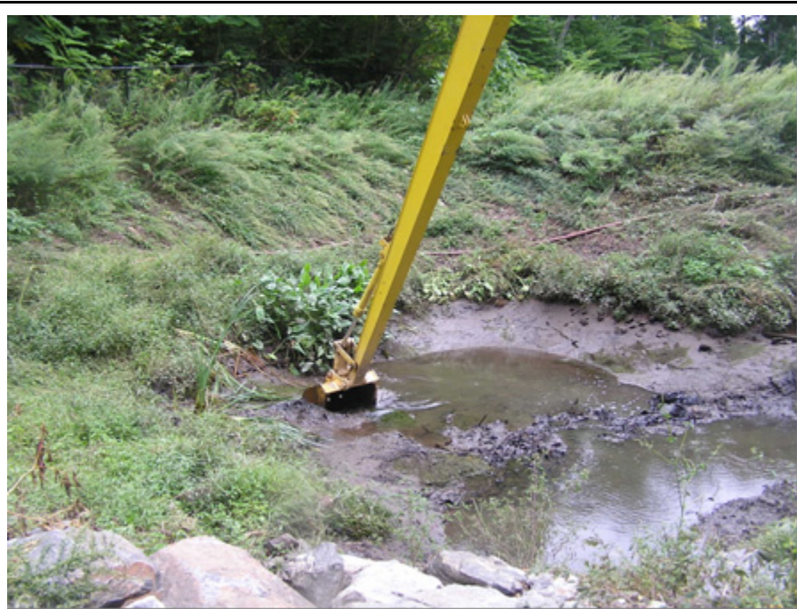
Figure 4.22 Accumulated sediment being removed.
