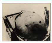
Then: Each of the three sections of the Delaware Aqueduct has a designated drainage shaft containing a pump chamber so that the tunnel may be dewatered. These shafts each contain an access drift which is closed by a watertight, cast-bronze door as seen in the image below. (hdq.d.2003; 1/10/1940)
