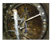
Now: Today, the bronze access door is a key element in ongoing work to repair the Delaware Aqueduct. In order to ensure that the tunnel can be dewatered safely, extensive research is being done by DEP engineers and contractors on the structural history and installation of the bronze access door. (Photograph by Ted Dowey; 1/23/2010)
