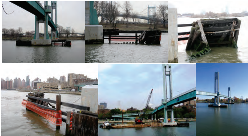
2014 - Wards Island Pedestrian Bridge – Collapsed Fender. July 2015 – Work Barge. November 2015. (2015 Credit: Jitendra Patel)
