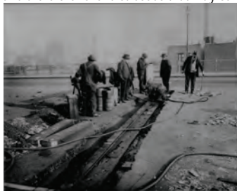
Constructing an Expansion Joint on the Riverside Drive Viaduct in 1918.
