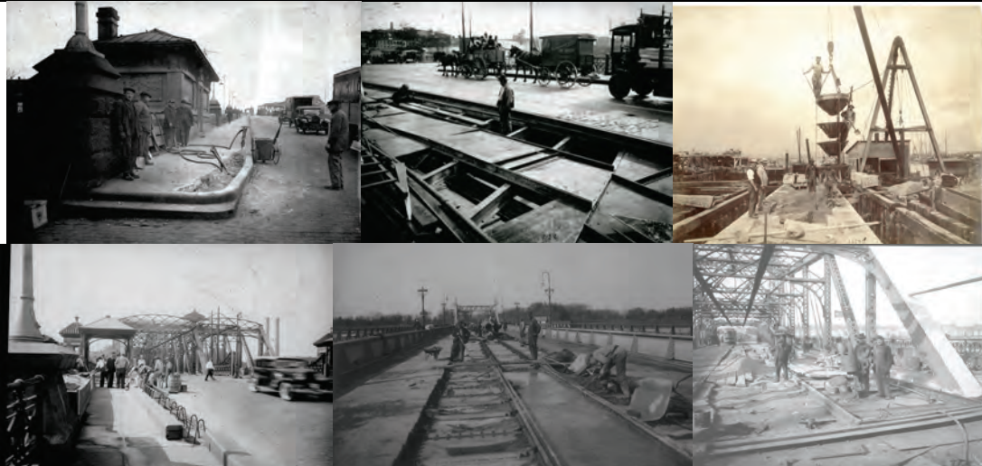
Willis Avenue Bridge Curbing and Road Repair in the Early 1920's. Madison Avenue Bridge Center Pier Under Construction in September 1909, and Constructing New Guardrail in September 1934. City Island Bridge Concreting in 1912. University Heights Bridge Roadway Repair in 1923.
