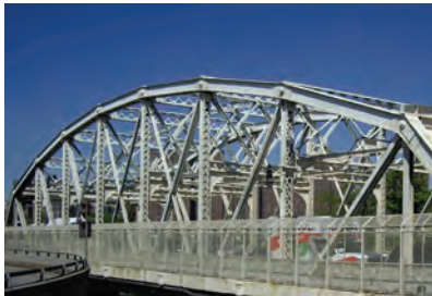
Macombs Dam Camelback Truss.
