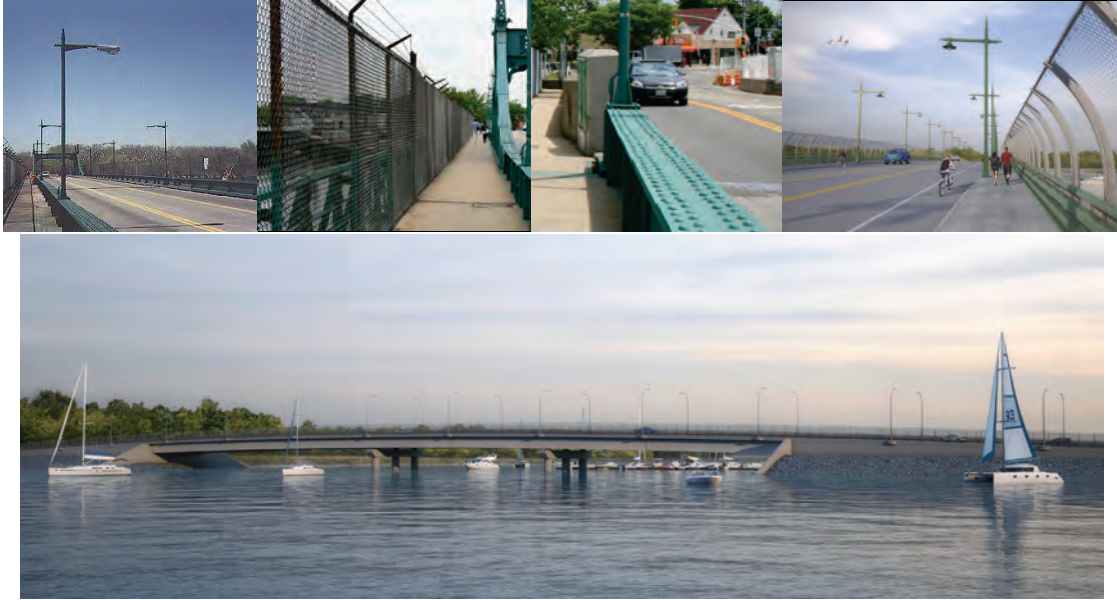
Existing and Proposed City Island Road Bridge Furnishings: Lighting, Fence, and Rail. Side View Rendering of New Bridge.
