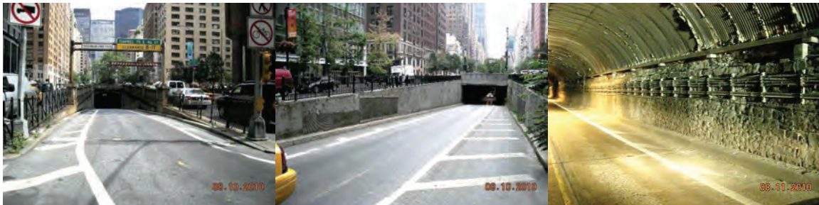
Two Views of Park Avenue Tunnel in 2010. (Credit: NYSDOT)
