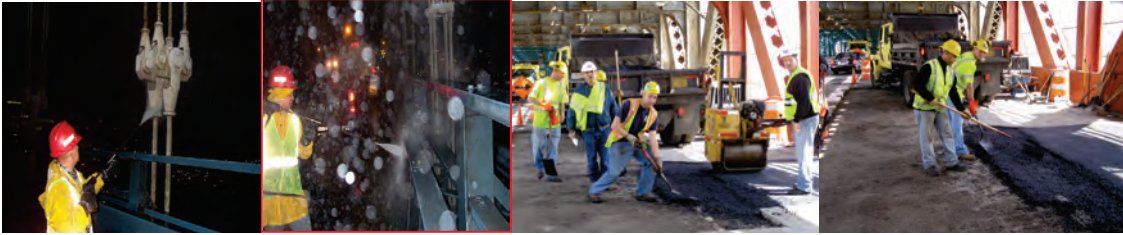
Power Washing the Corrosive Deicing Solvents Within the Range of the Roadway Splash Zone on The Manhattan Bridge in October 2007. Particular Attention is Directed to Cleaning the Gusset Plate. (Credit: Albert Hong) Performing Wear and Tear Resurfacing Work on the Roosevelt Avenue Bridges in April 2010: Assistant City Highway Repairer Victor Magagna, Supervisor Highway Repairer Joseph Palemine, Assistant City Highway Repairer Jonathan Adorno (Obscured), Assistant City Highway Repairer Anthony Montalbano, and Area Supervisor Highway Maintenance Edward Pedersen. Assistant City Highway Repairers Jonathan Adorno and Victor Magagna. (Credit: Joseph Flood)
