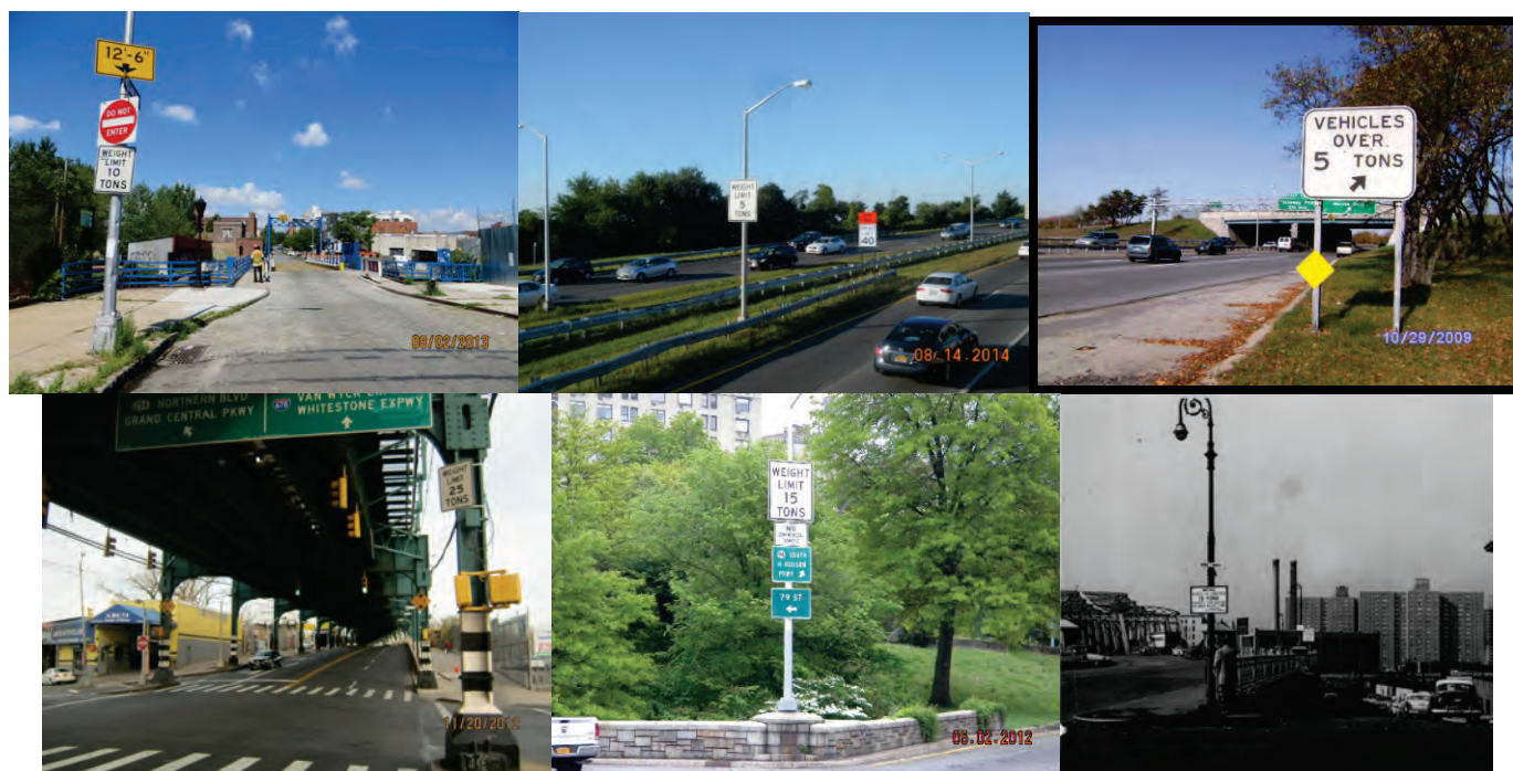
Carroll Street, Gerritsen Inlet, Mill Basin, Roosevelt Avenue Bridge and 79 th Street Ramp Posted Weight Restriction Signs. (Carroll Street, Gerritsen Inlet, Roosevelt Avenue and 79 th Street Ramp Credit: NYSDOT) Madison Avenue Bridge Posted Weight Restriction in Effect in 1959.
