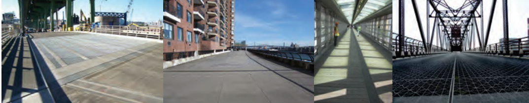
Hamilton Avenue Bridge, East 81 st to East 90 th Street Promenade over FDR Drive, Chambers Street Pedestrian, and Roosevelt Island Bridge Decks. (Hamilton and FDR Drive Credit: NYSDOT)
