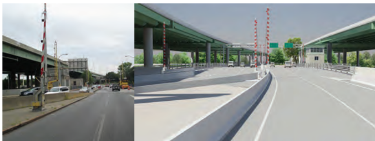
Looking East – Towards Current And Proposed Bridge.
