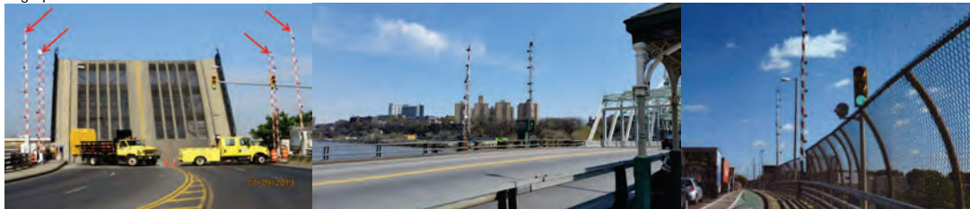
Metropolitan Avenue Bridge over English Kills Warning Gates. (Credit: NYSDOT) West 207 th Street/West Fordham Road Bridge Warning Gate. Greenpoint Avenue Bridge over Newtown Creek Southwest Warning Gate.
