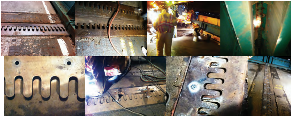
July 2013 PIA Safety Flag on the City Island Bridge. The repairs, conducted after a record-breaking heat wave, involved opening the joint plates and installing plug welds, which helped correct the plates' position and recreated the proper gap to allow the bridge to expand and contract safely. Finger Joint Before the Repair. Open Finger Joint. Division Crews Repairing the Joints. View Beneath the Finger Joint. The Joint Plates are Placed to Check for the Proper Gap. Leveling the Plate Before Welding. Close-Up of a Plug Weld. After 17 Plug Welds, the Finger Joints Sit Flush on the Roadway.
