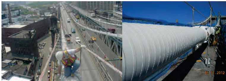
Inspector on Manhattan Bridge Cable. Cable B. (Credit: NYSDOT)
