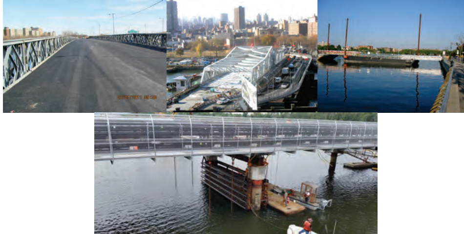
2011: Fresh Creek Temporary Bridge. 2004: Almost Completed New Third Avenue Span and Temporary Bridge. (Credit: Daniel Hom) 2005: Pontoon Bridge Used During the Emergency Reconstruction of the Ocean Avenue Pedestrian Bridge over Sheepshead Bay. (Credit: Russell Holcomb) 2015: City Island Temporary Bridge.
