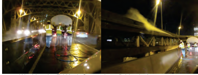
Washing the Ed Koch Queensboro Bridge in August 2011.
