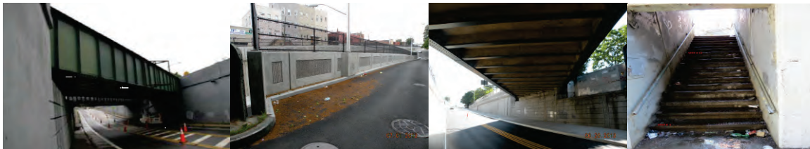
71 st Avenue Bridge over Cooper Avenue. Left Concrete Parapet/Guide Rail. Span 1 Bridge Framing. (Parapet and Span Credit: NYSDOT) Stairway at Right Side of Beginning Abutment.
