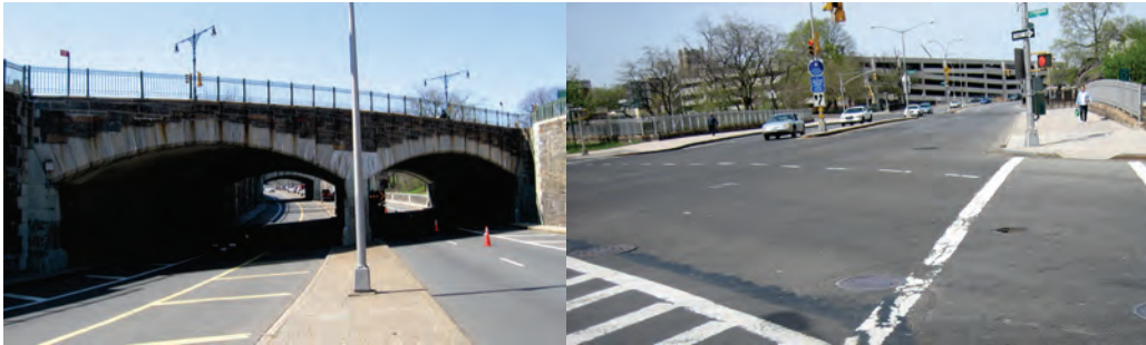
Southern Boulevard Bridge over East Fordham Road.
