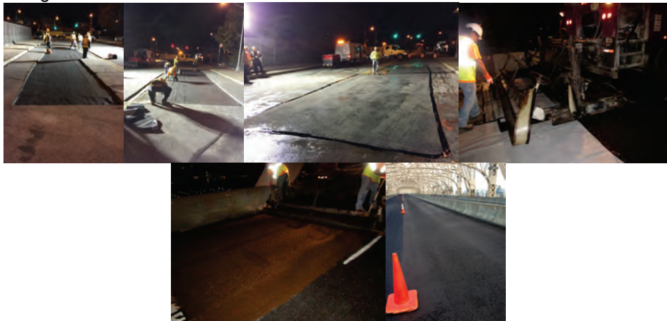
November 2014: Wearing Surface Repairs at 149 th Street over the Cross Island Parkway. Applying the Waterproofing Membrane. The Finished Patch. (Credit: Steve Mezzacappa) Resurfacing the Deck of the Queens-Bound Upper Roadway of the Ed Koch - Queensboro Bridge in June 2014. (Credit: Sunil Desai)
