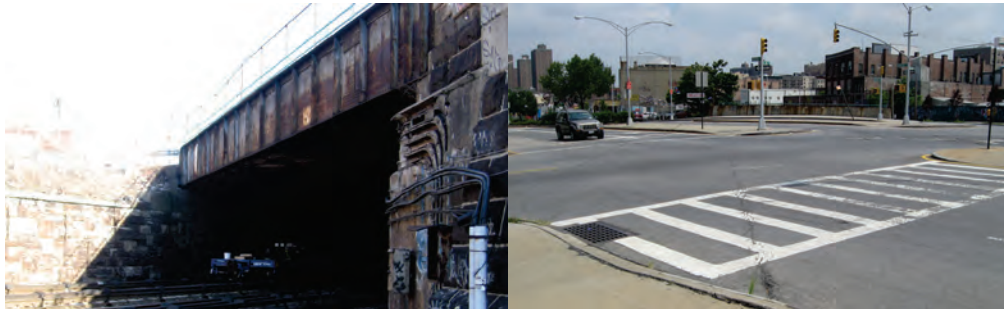
East 165 th Street Bridge over MNRR.
