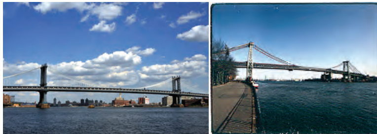
Manhattan Bridge. (Credit: Bernard Ente) Williamsburg Bridge. (Credit: Peter Basich)
