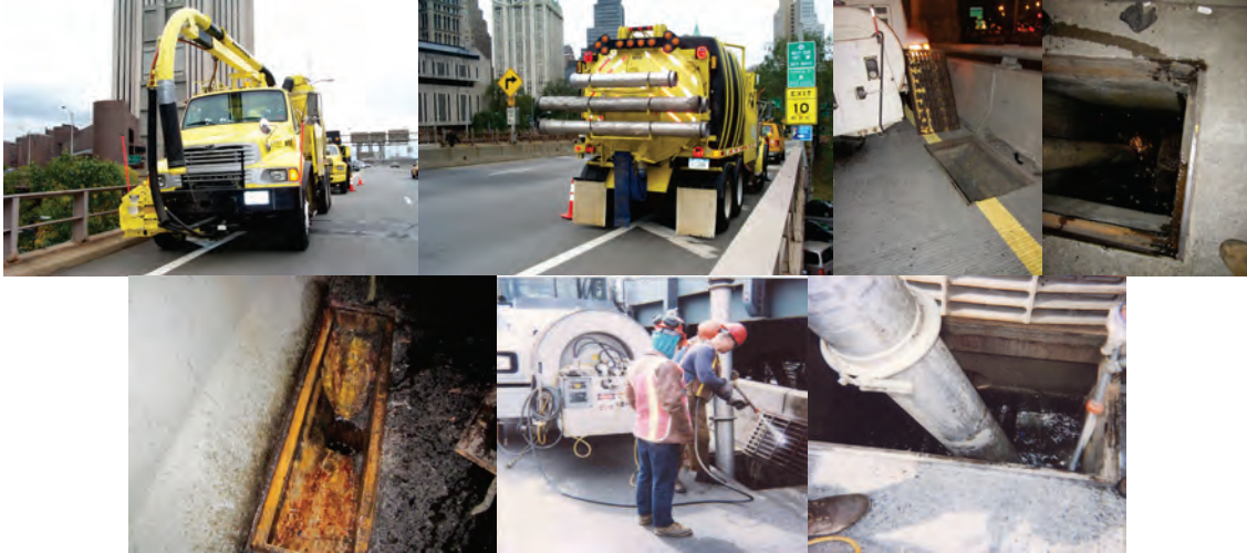
Drain Truck on Brooklyn Bridge Ramp. (Credit: Peter Basich) Drain Cleaning on the Williamsburg Bridge in September 2011. (Credit: Shaikh Islam) Cleaning Catch Basins on the Manhattan Bridge.
