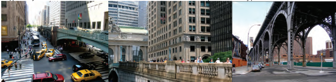
Park Avenue Viaduct Bridge. Experiencing the Viaduct in a Whole New Way During Summer Streets 2012. Riverside Drive Viaduct.
