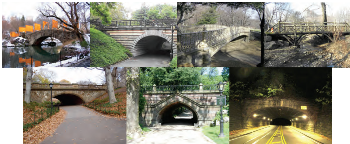
Gapstow Bridge (East 62 nd Pedestrian Bridge) During the Exhibition The Gates, Project for Central Park, 1979-2005 . (Credit: Russell Holcomb) Center Drive Bridge (Playmates Arch) in 2008. West 62 nd Pedestrian Bridge (Pinebank Arch). West 77 th Street Pedestrian Bridge (Ladies Pond Bridge). East 77 th Street Pedestrian Bridge (Glade Arch) in 2010. Greywacke Arch (East Drive Bridge Opposite East 80 th Street) in 2011. East Drive Bridge over Transverse Road #3 in 2015.
