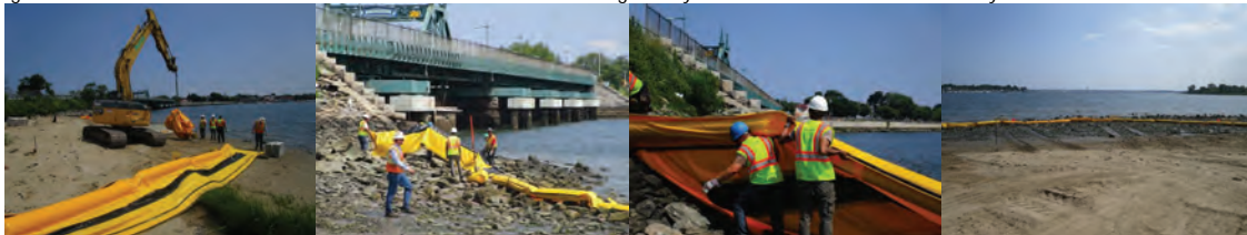
Installation of a Turbidity Curtain to Protect the Shore During Construction of the Temporary City Island Bridge in 2014.
