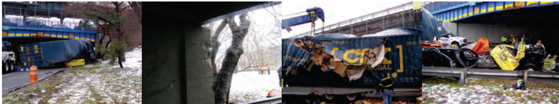
Damaged Bridge, Cargo Container, and Contractor Truck After An Over-Height Trailer Struck the Bridge in January 2012.
