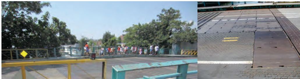
Union Street Bridge - Schoolchildren Crossing in 2012. (Credit: NYSDOT) 2014: Eleven Steel Plates Covering the Steel Grid Deck.
