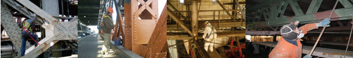
Williamsburg Bridge in June 2010: Application of Finish Coat at North Truss Diagonal. Salt Splash Painting on the Williamsburg Bridge. (Salt Splash Credit: Fouad Althaibani). Inspection of Blasting Surfaces Inside the Franklin Square Arch Containment in September 2010. Brooklyn Bridge Main Span Painting in December 2010.
