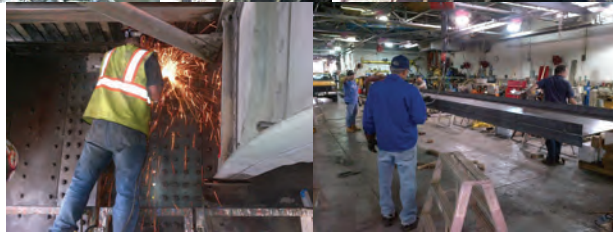
August 2013 Red Flags on the Ed Koch Queensboro Bridge. A truck caught fire on the bridge and damaged three stringers that support the eastbound upper roadway. Replacement of the two damaged stringers and the repair of a third were completed in October 2013. All work was performed by in-house forces. August 2013: Firefighters Examining the Damage. Repairing the Bridge Included Custom Designing the Steel Beams, as Well as Fabrication and Installation. Division Ironworkers Fabricated Two 26-Foot-Long, 1.5-Ton Beams in Their Brooklyn Shop.
