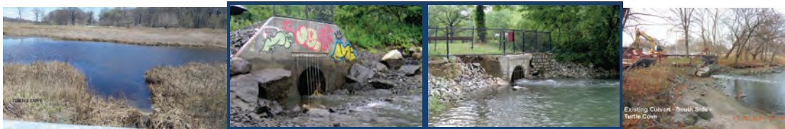
Turtle Cove. Existing Culvert – South Side.
