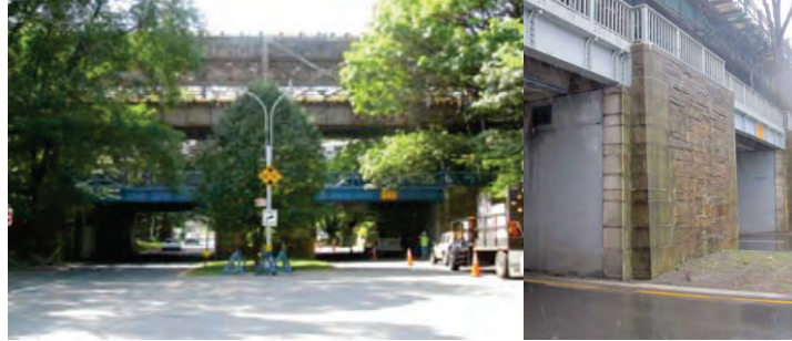
Roosevelt Avenue Bridge Over Flushing Meadow Park Road. Left Side Span 2.
