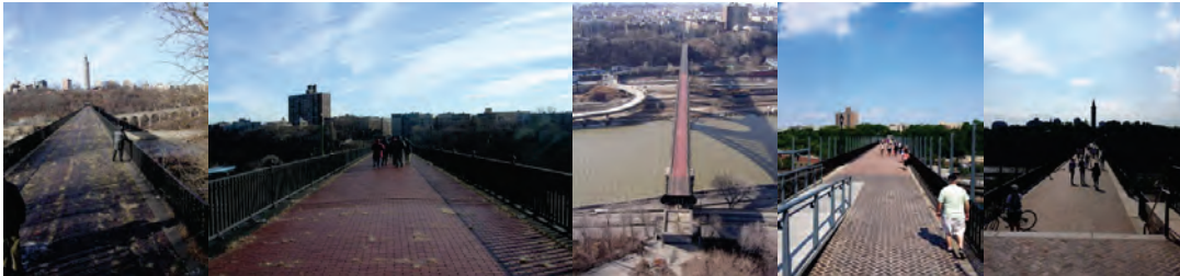
High Bridge Walkway in January 2004 and June 2015. The Brickwork Dating to the 1860's was Restored at Either End, With the Center Section was Completed With Replicas. (Credit: Gordon I. Goldberg)
