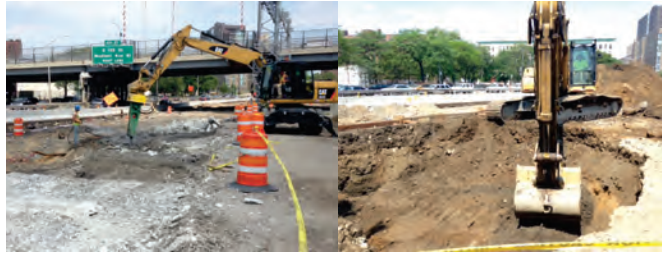
February 2015: Removing the Massive Reinforced Concrete Substructure Near the Third Avenue Bridge. Excavating and Removing Big Rocks. (Credit: Artemio Angeles)
