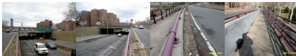
The Three Structures of the FDR Drive at Houston Street Overpass. 2014: Main Bridge – Left and Right Elevations. South Approach Ramp - Span 2, Left Side Safety Walk and Curb. North Approach Ramp - Span 2, Top of Cantilevered Pedestrian Walkway. (Credit: NYSDOT)
