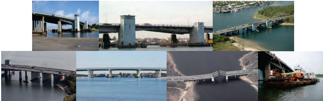
Current Belt Parkway Bridge Over Mill Basin. Aerial Views. Proposed Bridge. Open Bridge. May 2013 – Inspecting the Bridge From a Barge.
