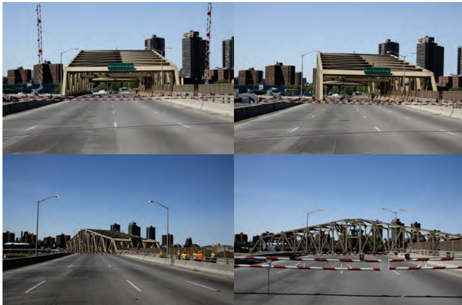
Sequence Showing the Span Opening as Seen From the Bridge.
