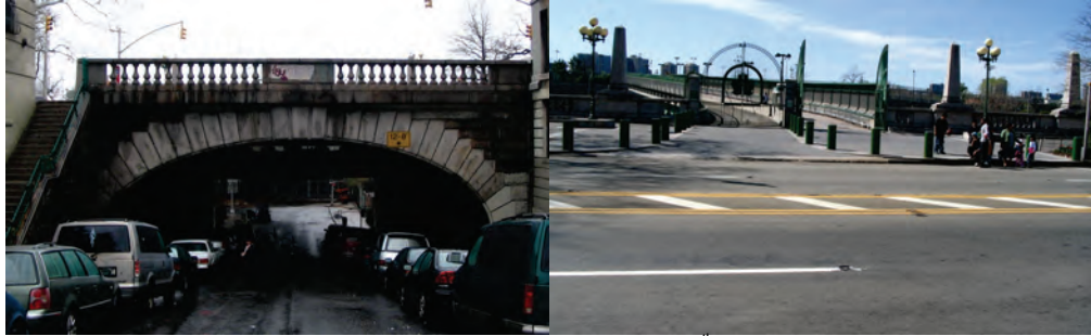
Riverside Drive Bridge over West 138 th Street.
