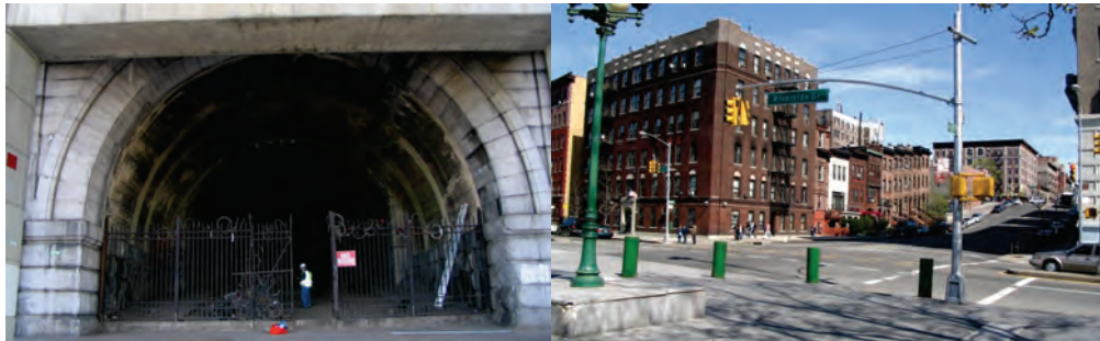
Riverside Drive Bridge over West 145 th Street.
