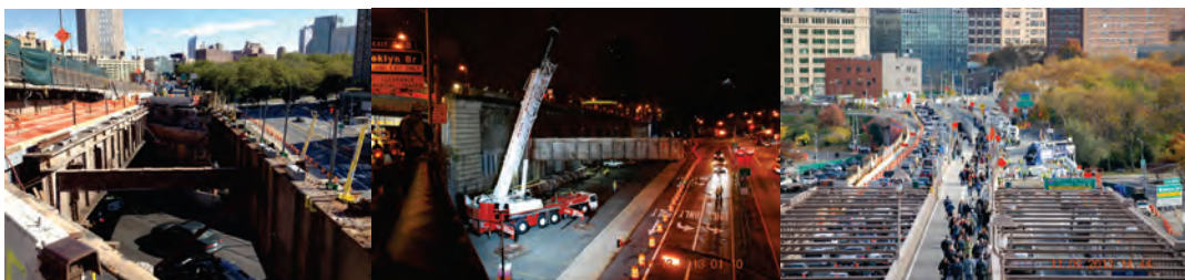
October 2013: Eastbound Brooklyn-Queens Expressway Traffic Flowing Under the Exposed Steel of the Eastbound York Street Structure. Removing the Fascia Steel From the Eastbound York Street Structure. November 2013: Concrete Placement at the Eastbound York Street Structure.
