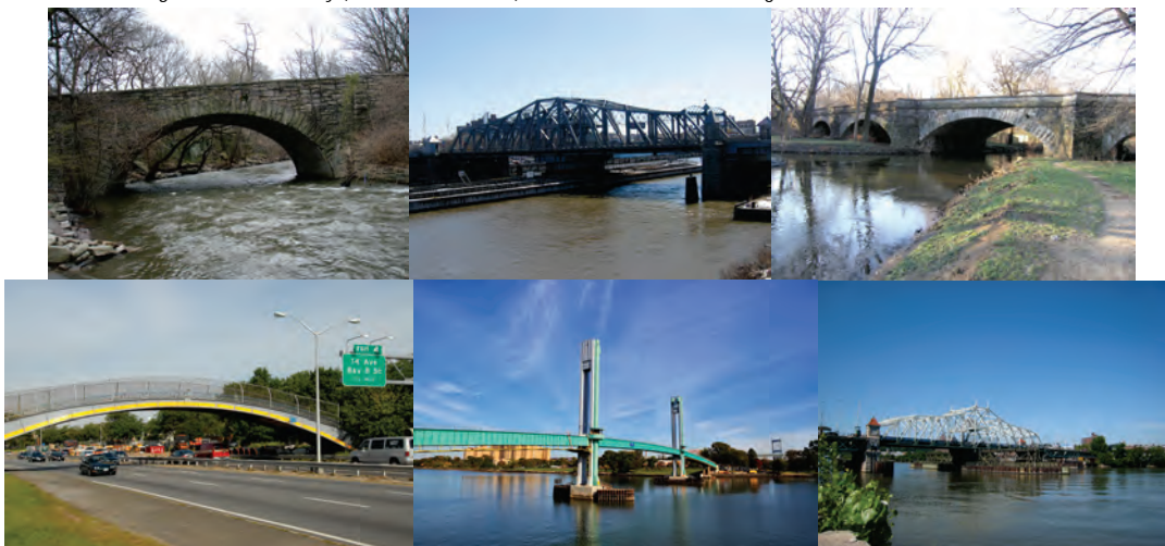
Southern Boulevard, Madison Avenue, and Mosholu Parkway Bridges. (Credit: Russell Holcomb) 17 th Avenue Pedestrian Bridge. (Credit: Peter Basich) Wards Island Pedestrian Bridge in October 2011. (Credit: Rafael Lopez) University Heights Bridge in July 2011. (Credit: Russell Holcomb)
