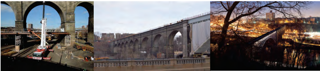
Late Fall 2013: Mast Climber Removal. Winter 2014: South View of the Bridge. (Credit: NYCDDC)
