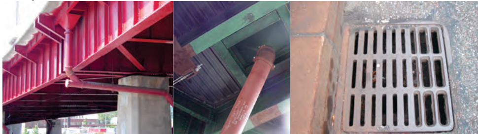
Scuppers on the Pulaski, Madison Avenue, and Brooklyn Bridges. (Credit: NYSDOT)
