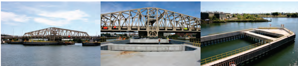
September 2012: Bridge Fender North Elevation Looking South. Bridge South Elevation Looking North. Pier 6 South Fender Looking South.
