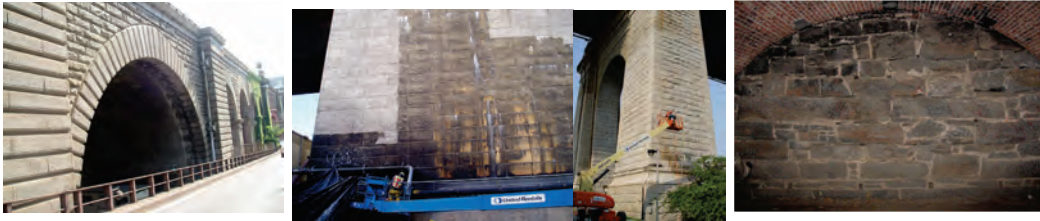
Brooklyn Bridge Cliff Street Arch Masonry. Cleaning the Masonry of the North Face of the Manhattan Bridge's Brooklyn Anchorage and of the North and East Faces of the Roosevelt Island Pier of the Ed Koch Queensboro Bridge. Masonry of the East Drive Bridge Over Eastwood Arch.
