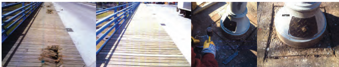
May 2015 Safety Flag: Borden Avenue Bridge Over Dutch Kills - Wooden Planks of Sidewalk Damaged After Vehicle Accident. East 14 th Street Bridge Over LIRR Bay Ridge –Ironworkers Fabricated and Installed the Bottom Cover of the Ventilation Post on the Right Sidewalk.
