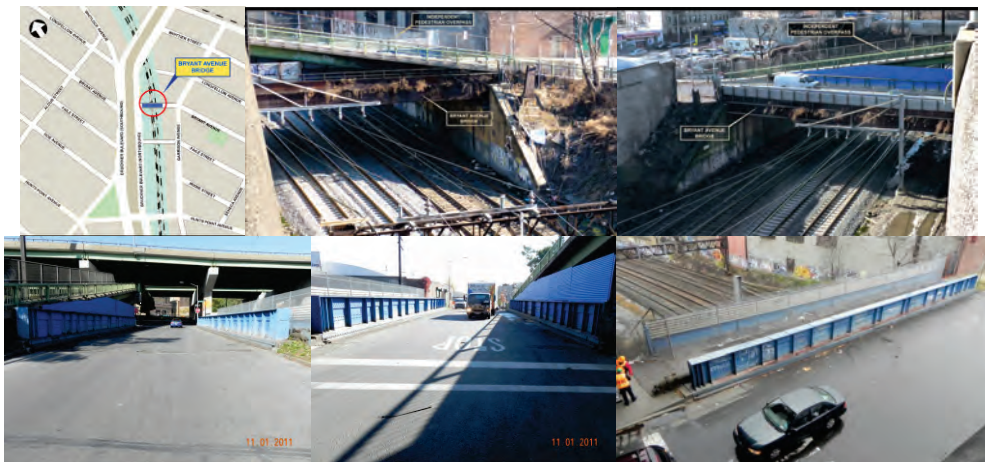
Location Map. Bridge Views Looking North and South. 11/1/11 Approach Begin and End. (Credit: NYSDOT) Bridge View From the Pedestrian Overpass.
