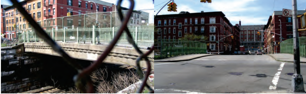
East 187 th Street Bridge over MNRR.
