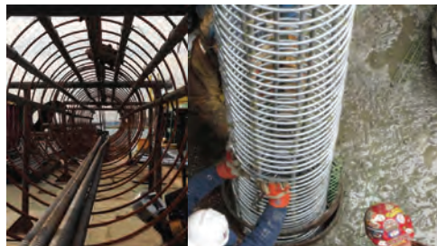
City Island and Gerittsen Inlet Bridge Rebar Cages.
