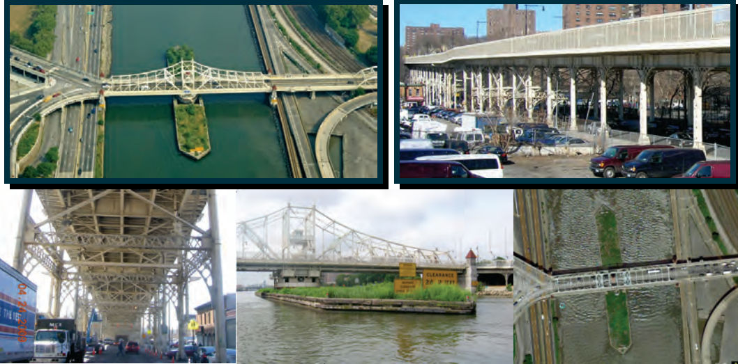
Aerial View. West 155 th Street Viaduct. The Timber Fender.
