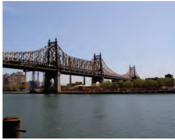
Ed Koch Queensboro Bridge (Credit: Russell Holcomb)
