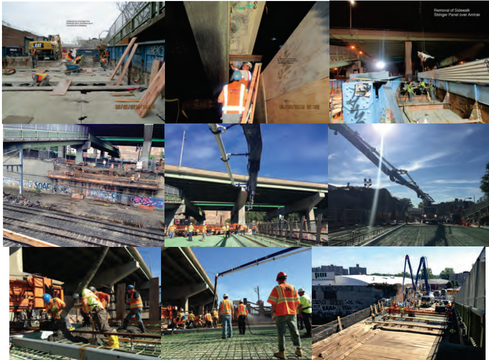
March 2015: Chipping Out Roadway Deck Concrete and Removing Shielding Concrete. May 2015: Installing Overhang Brackets on South Side of Pedestrian Walkway. Removal of Sidewalk Stringer Panel. Summer 2015: Existing Structure Removed. September 2015: Placing the Concrete for the Bridge Deck. The Concrete Pump Placed 110 Cubic Yards of Concrete Into the Deck. Covering and Protecting the Fresh Concrete with Wet Burlap.
