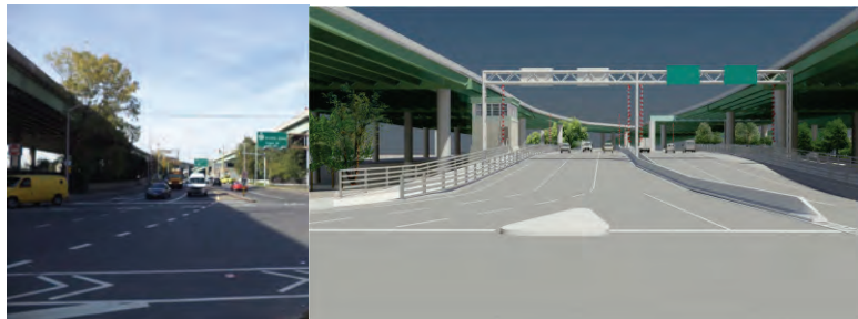
Looking West – Towards Current And Proposed Bridge.
