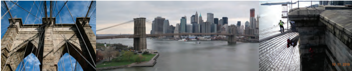
Brooklyn Bridge: 2009 Tower Closeup, 2010 View, 2010 Biennial Inspection. (2009 Credit: Emily Goodman, 2010 Credit: Jaglar Khinda, Inspection Credit: NYSDOT)
