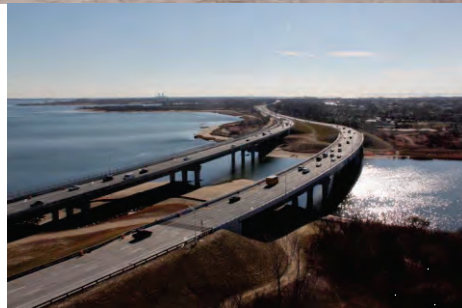
Old Paerdegat Basin Bridge. New Bridges in November 2013.
