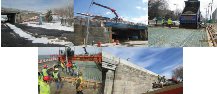
February 2015: Northwest Abutment and Wingwall Prior to Stonework Restoration. March 2015: Installation of Temporary Concrete Barrier on Eastbound Bridge in Response to a Red Structural Flag. Dumping Sub Base Soil for East Approach Deck. Placing and Finishing the Deck Wearing Surface for the Stage III Concrete Deck. Workers Resetting the Stone Facing on the Northwest Abutment and Retaining Wall.
