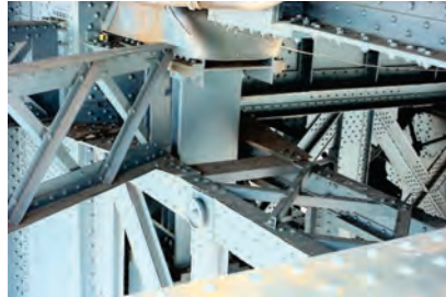
Truss Bearing on Manhattan Bridge. (Credit: NYSDOT)
