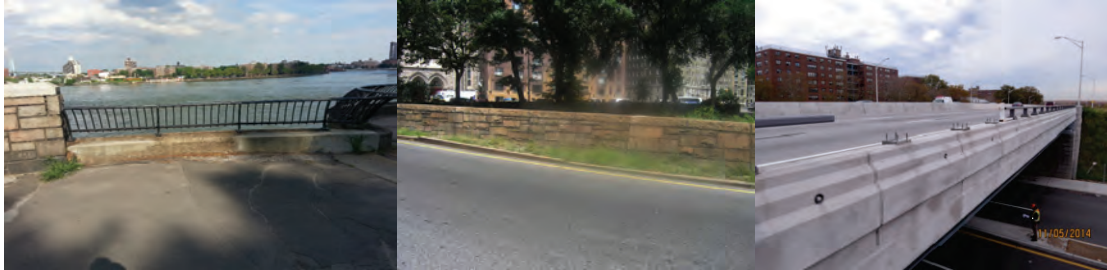
East 81 st to East 90 th Street Promenade over FDR Drive – Right Parapet at Span 45. West 65 th Street Entrance Eastbound over Bridle Path West End – View From End of Left Side Parapet. Belt Parkway Bridge over Rockaway Parkway – Right Side Parapet. (Promenade and Rockaway Parkway Credit: NYS DOT)
