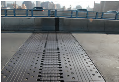
Manhattan Bridge Finger Dam. (Credit: Jagtar Khinda)
