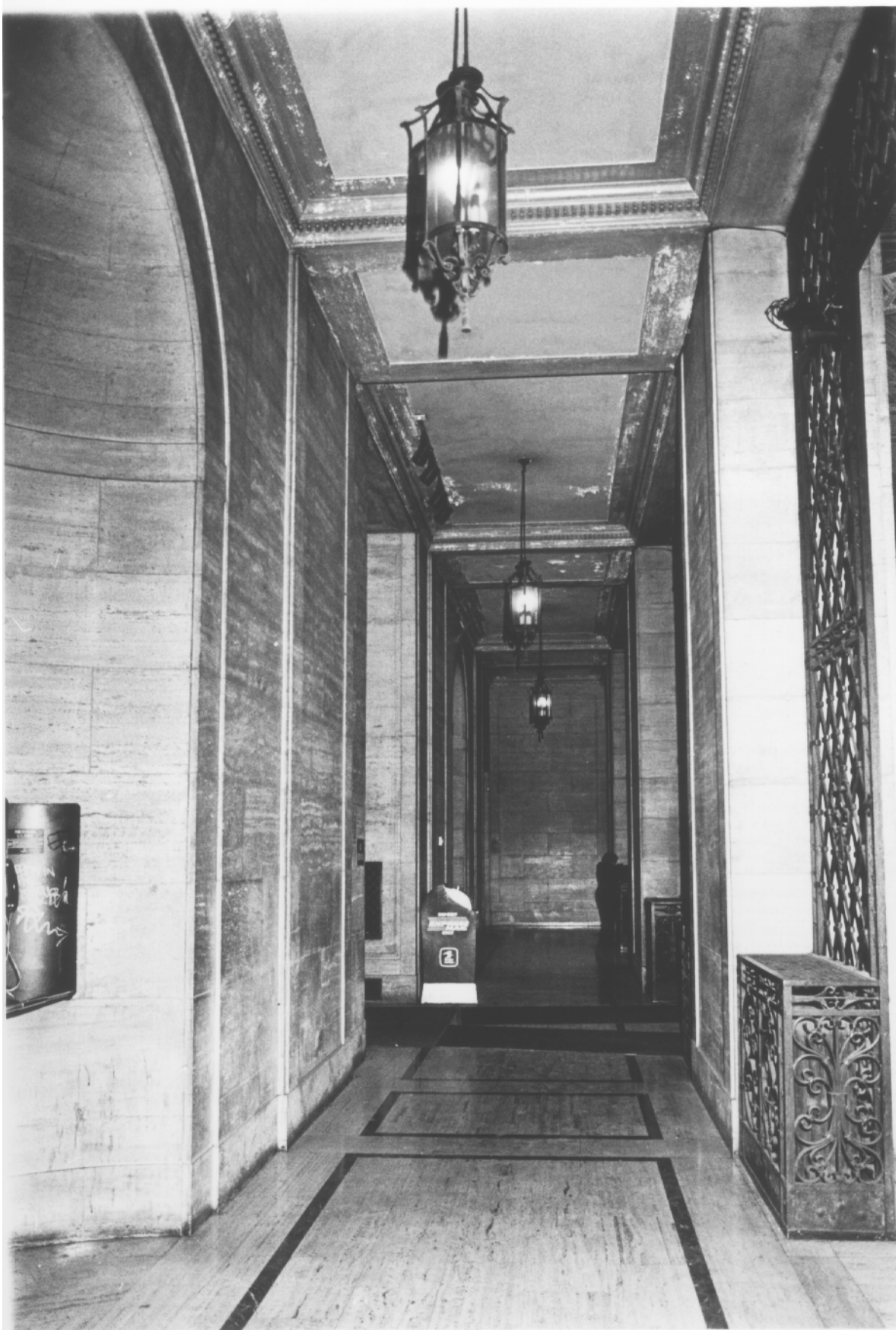
Fig. 9 Cunard Building Interior, Passageway
