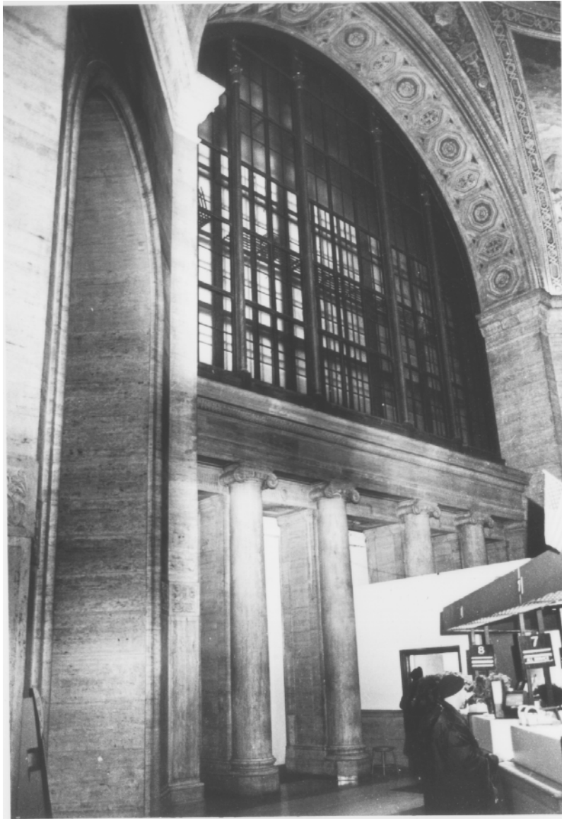
Fig. 11 Great Hall, detail of south elevation
