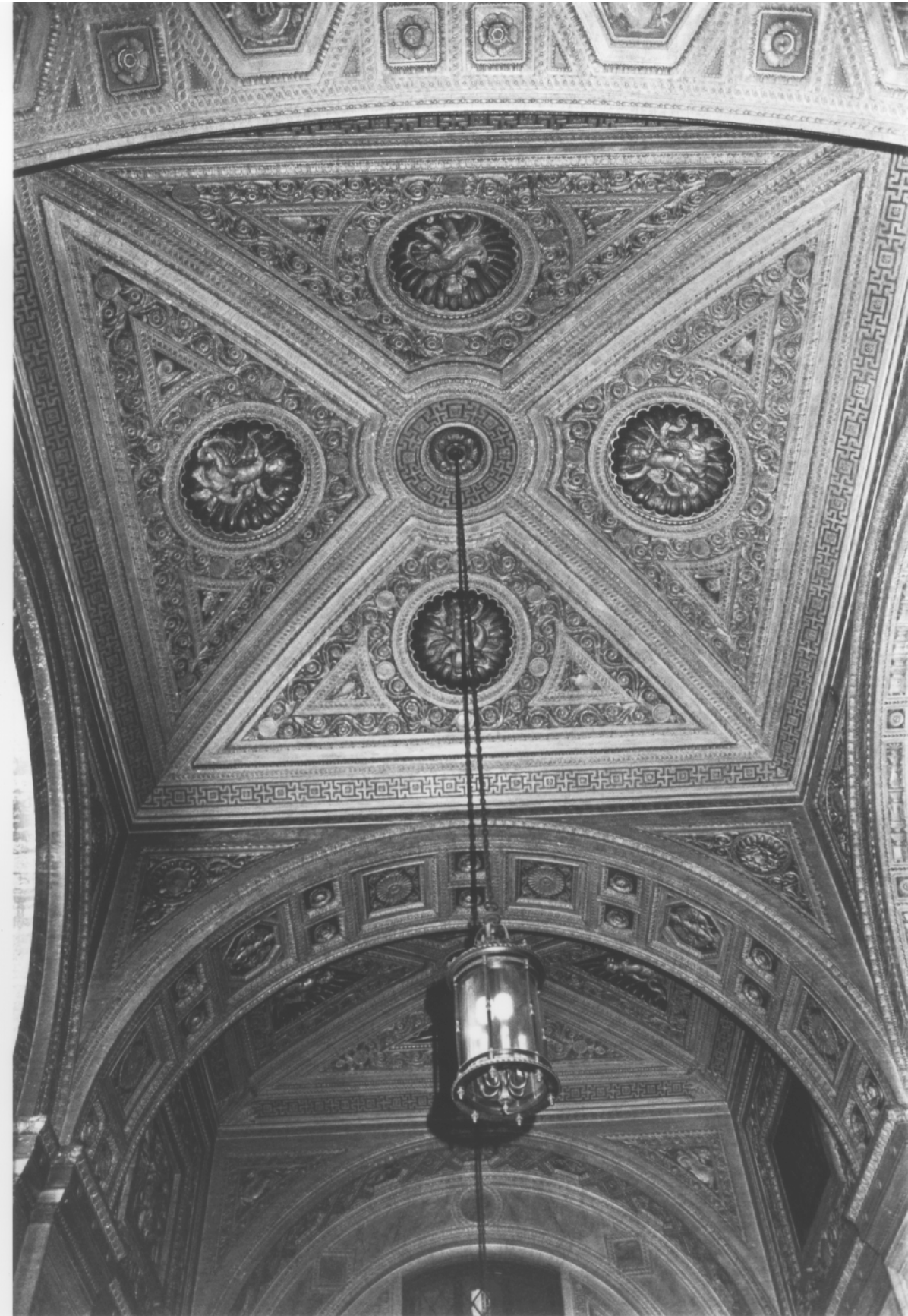
Fig. 7 Cunard Building Interior, Detail of ceiling in lobby
