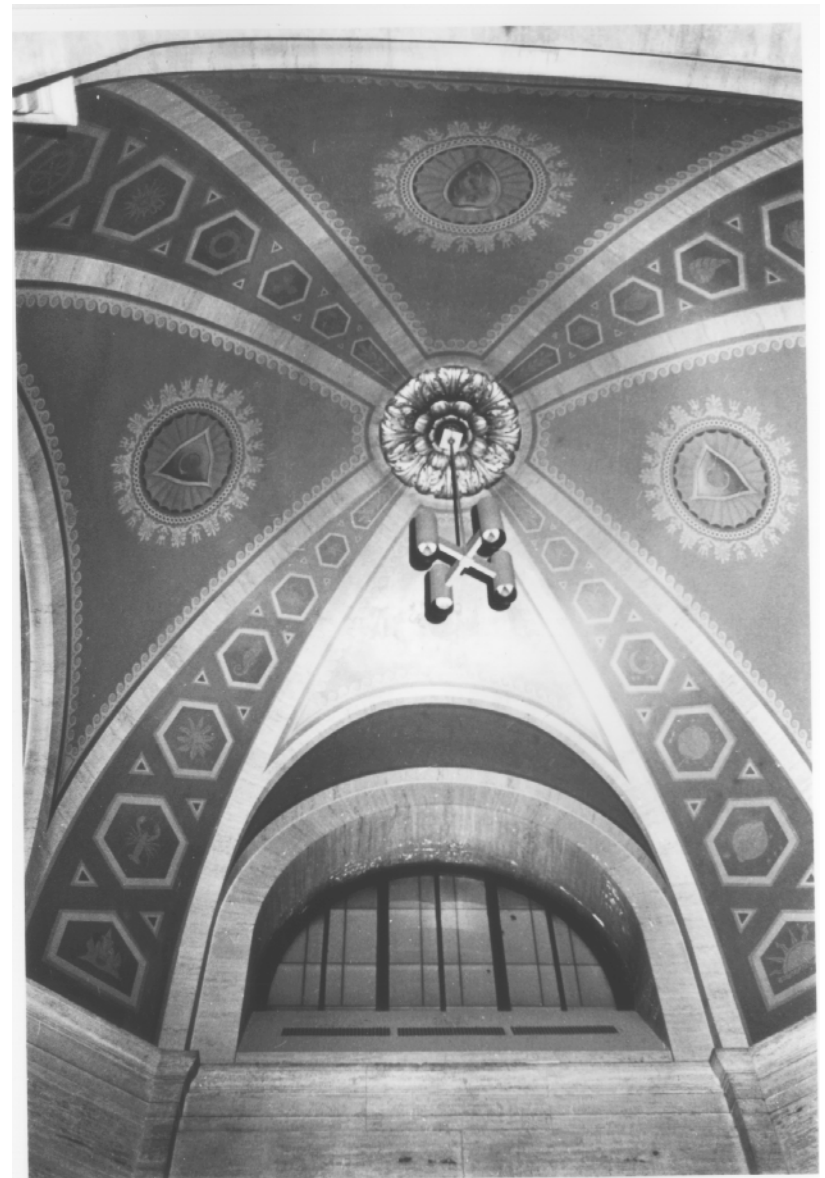
Fig. 16 Great Hall, dome of a "luminary square"
