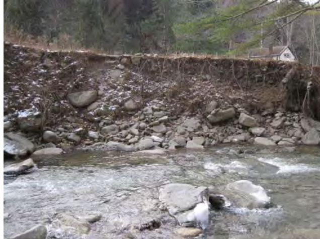
Photo 2: Bank scour on left bank downstream of unnamed private drive bridge.
