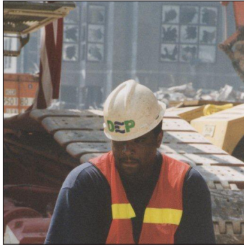
BWSO Construction Laborer Terrence Johnson, Manhattan Sewer Maintenance, at work at the WTC site.
