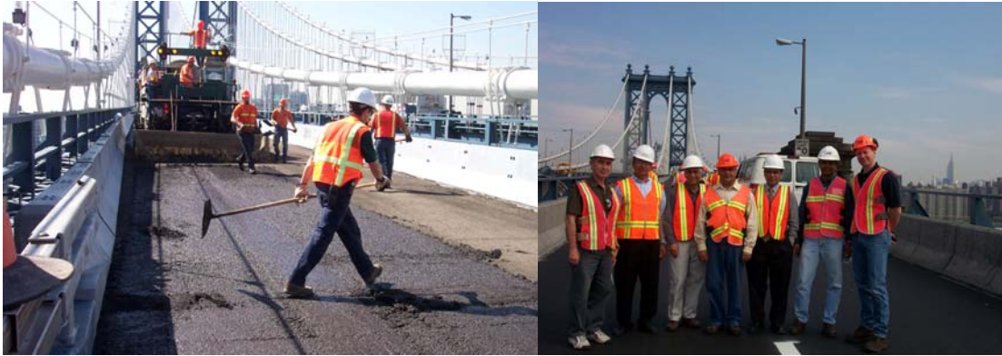
Microsurfacing of the Manhattan Bridge Steel Deck (Credit: Yuliy Zak)
