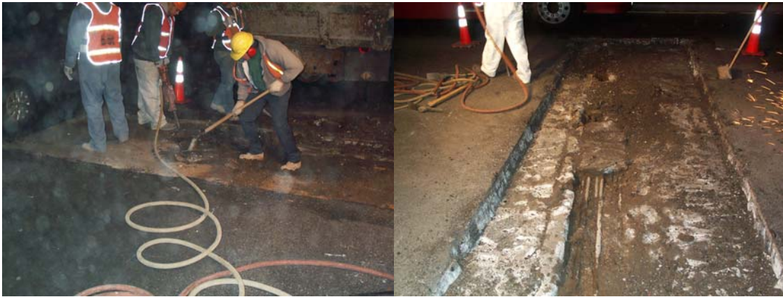
Breaking Out the Asphalt Under the Plate to Expose the Condition. Exposed Rebar at the Construction Joint. (Credit: Joseph Saverino)
