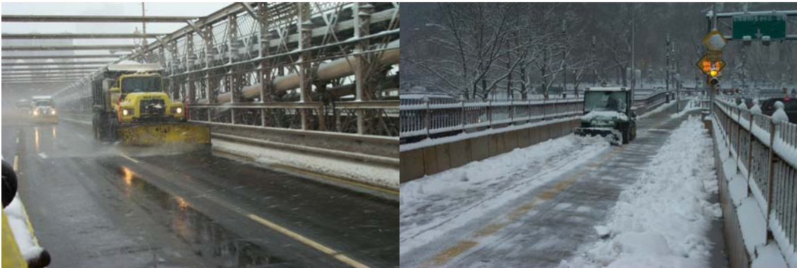
Applying Anti-Icing Chemicals & Removing Snow from the Brooklyn Bridge Walkway (Credit: Anthony Napolitano)
