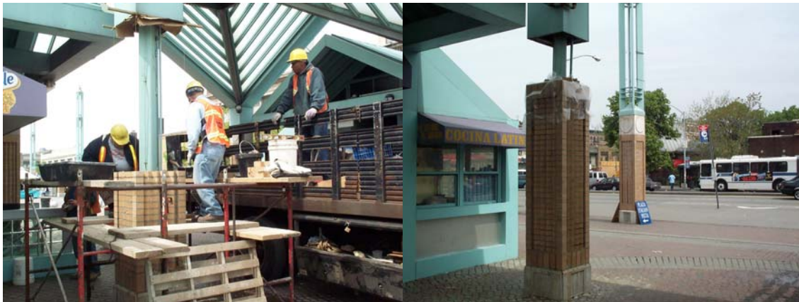
Bricklayers Luigi Cuffari and Paul Stolpiniski, and Highway Repairer Timothy Pope Rebuilding a Column. A Nearly Completed Column With Matching Existing Column in Rear. (Credit: Joseph Saverino)
