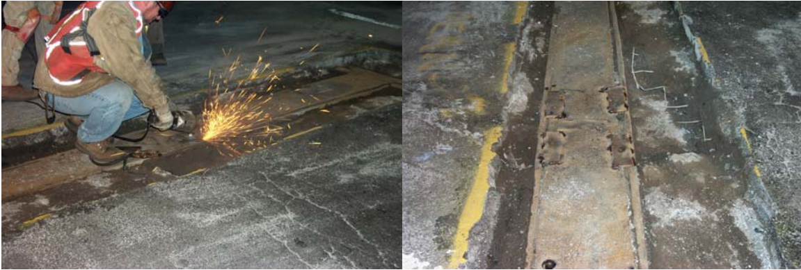
Repairing the Expansion Joint. (Credit: Anthony Napolitano)
