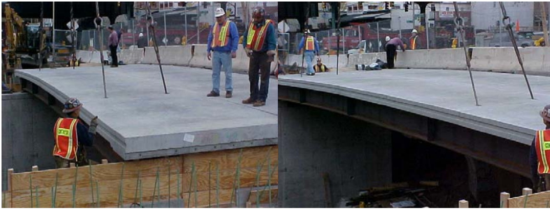
Installing the Precast Panels
