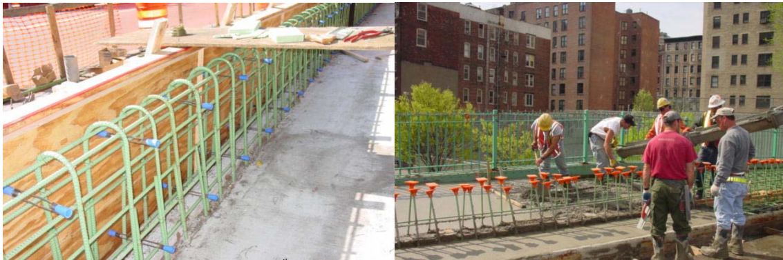
Formwork for the Concrete Barrier on 96 th Street to Protect the Public From Vehicular Traffic. Concrete Pour for the Sidewalk Replacement With Rebars Exposed for the Concrete Barrier (Credit: Nasir Khanzada)
