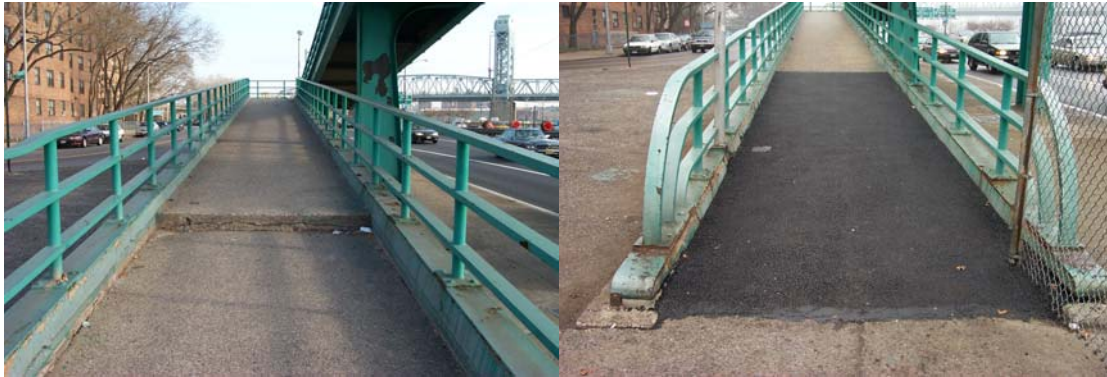
Southbound Ramp Before and After Safety Flag Concrete Repairs (Credit: Anthony Napolitano)
