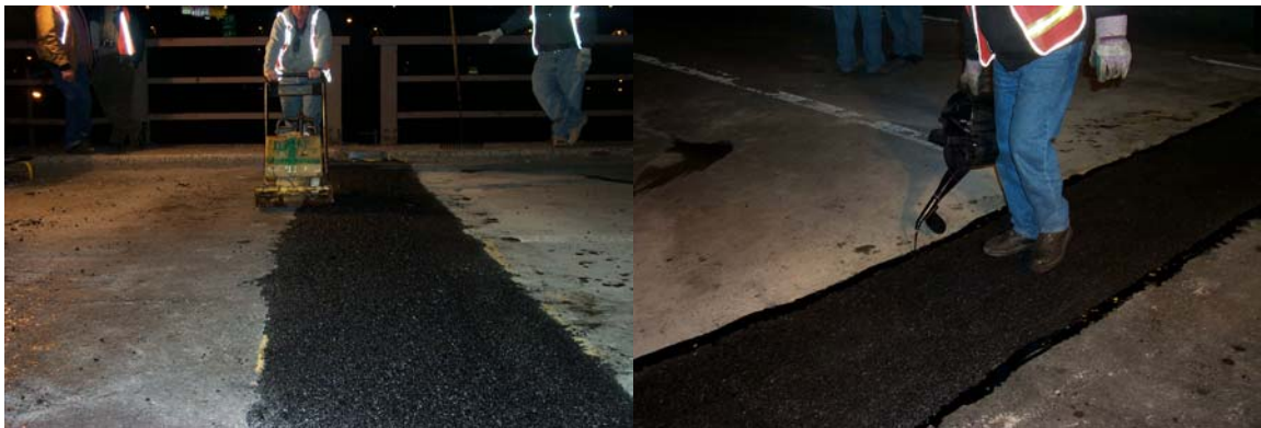
Placing Fresh Asphalt. (Credit: Anthony Napolitano)
