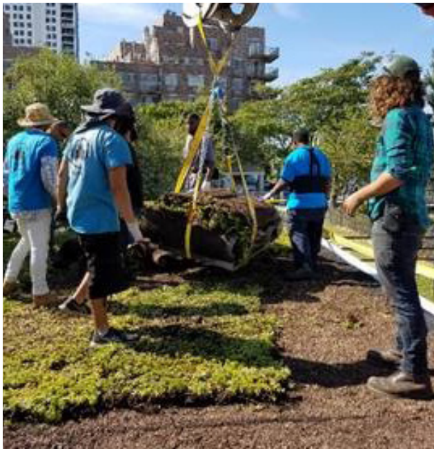
Green roof being installed at a Parks playground at Rockaway Beach
