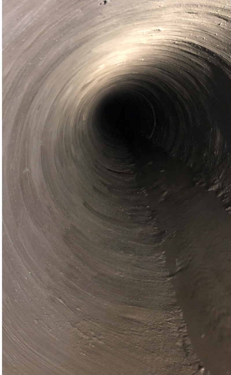
Brick sewer after geopolymer rehabilitation
