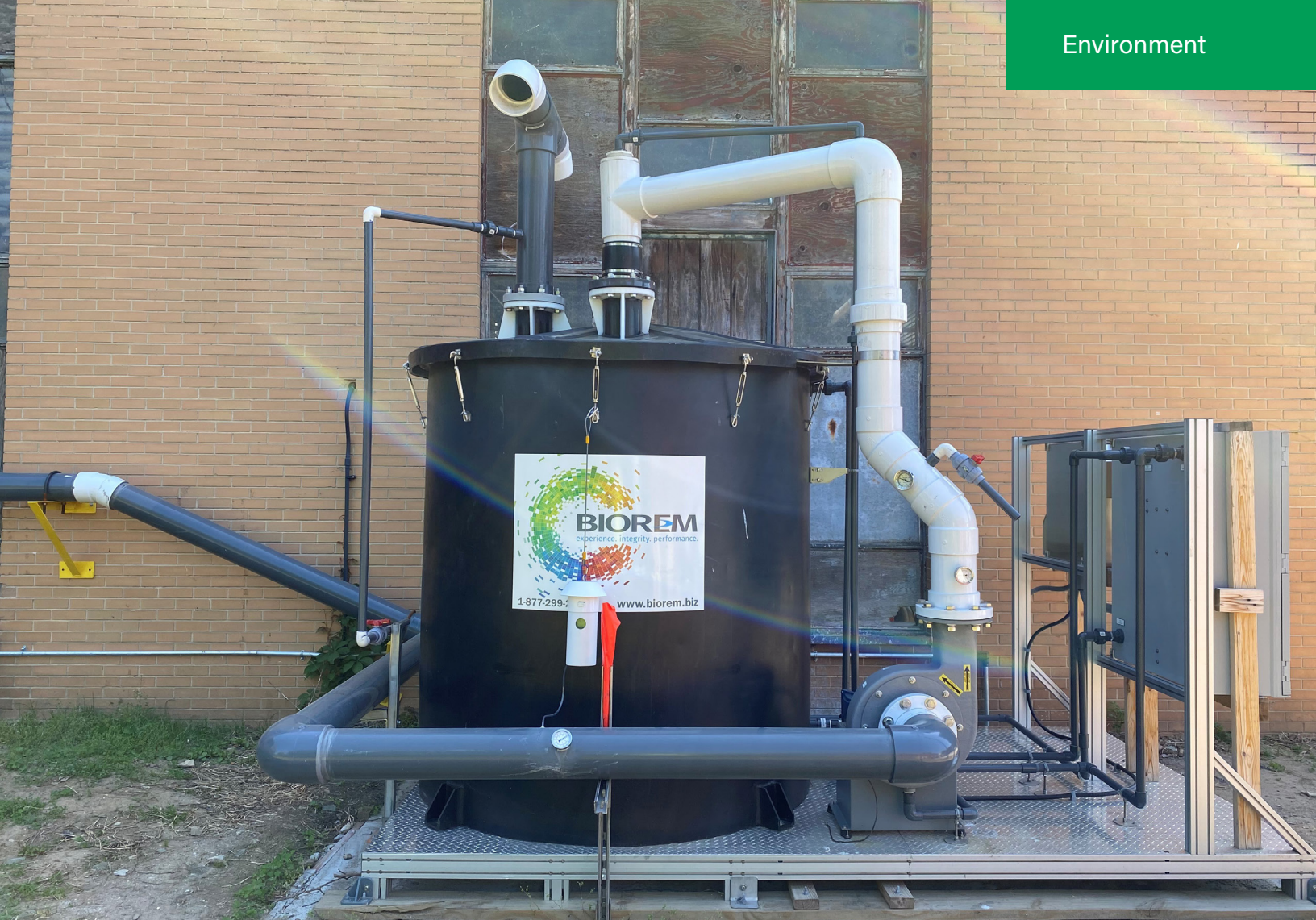
Biofilter at the Hunts Point WRRF
