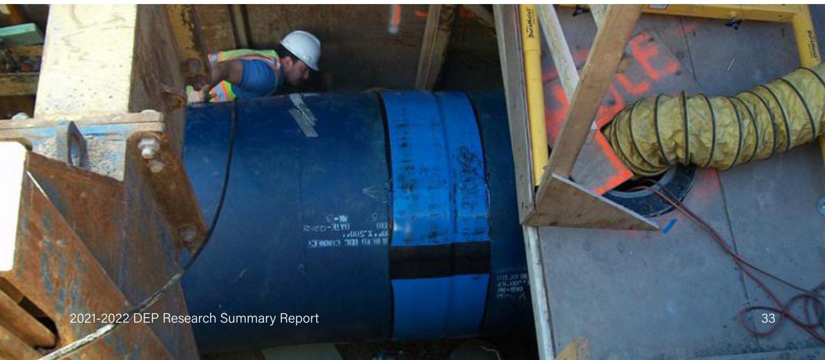
Polyurethane-coated steel trunk water main with heat shrink sleeve on joint
