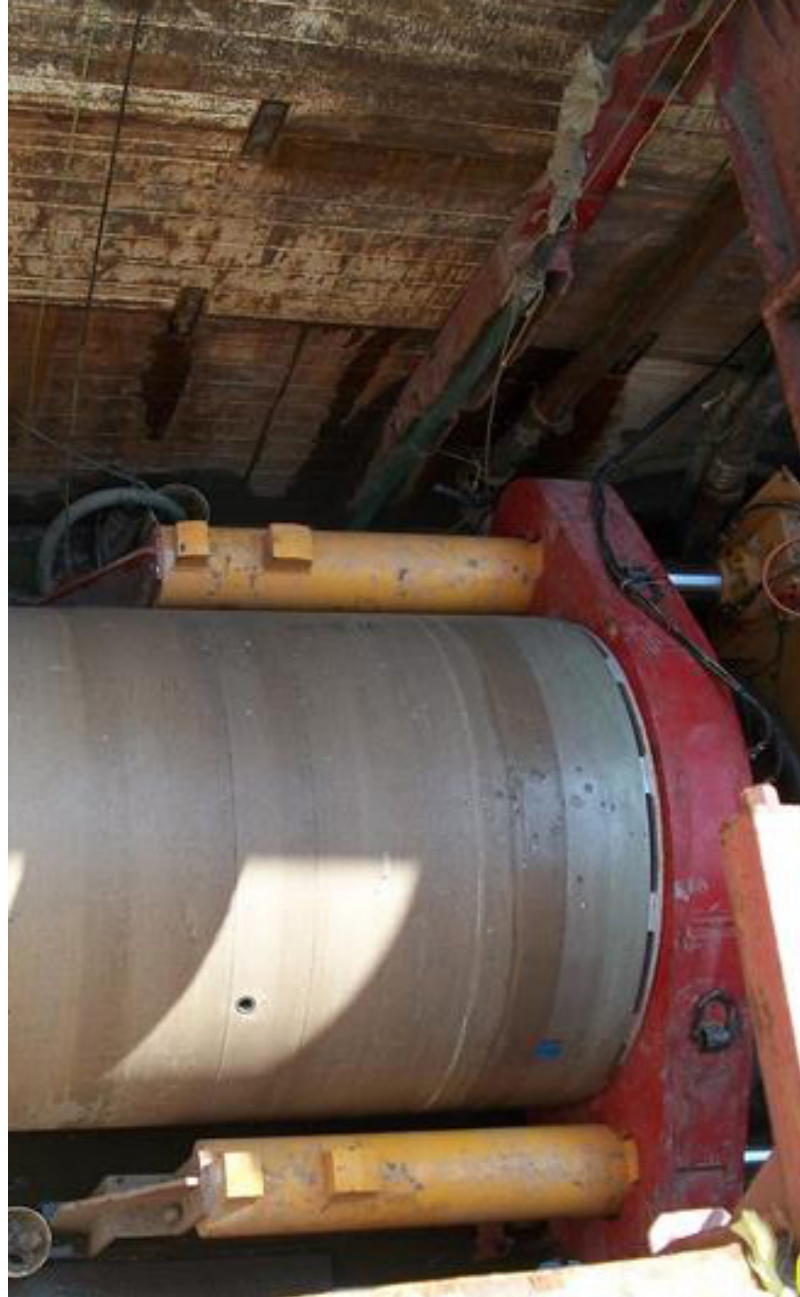
Microtunneling for CCFRPMP sewer installation
