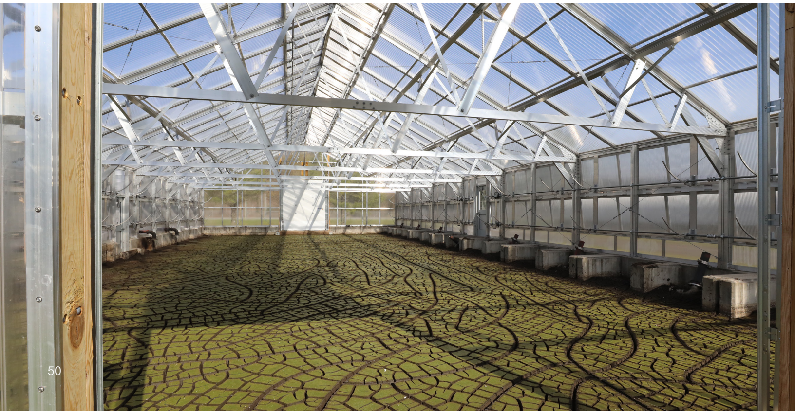
Sludge-drying greenhouses at the Margaretville Wastewater Resource Recovery Facility
