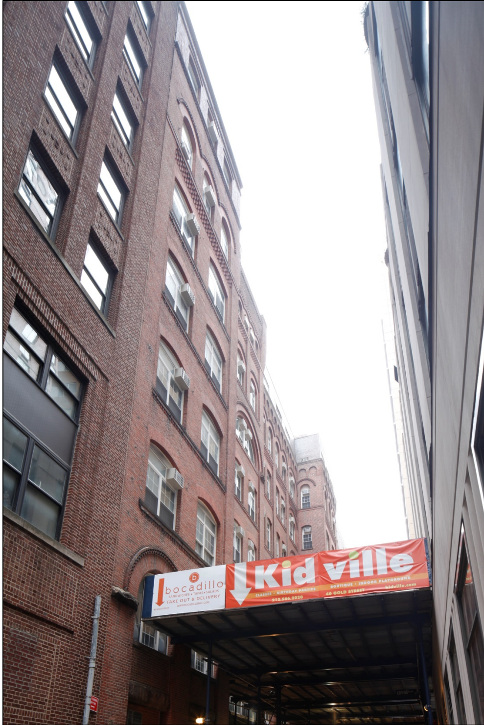
Excelsior Steam Power Company Building 33-43 Gold Street, Manhattan Block 77, Lot 24 in part Main facade Photo: Sarah Moses, 2016
