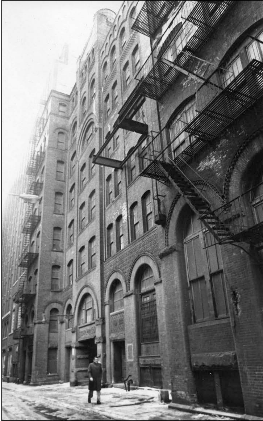
Excelsior Steam Power Company Building, circa 1977 LPC files
