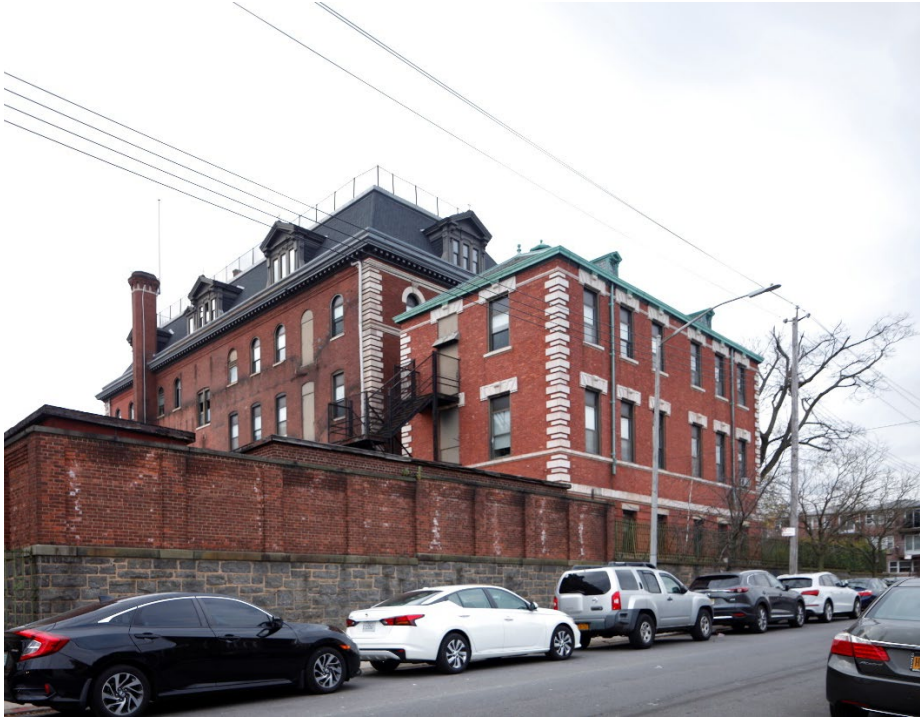
North Wing 63rd Street facade (rear) Jessica C. Baldwin, November 2020
