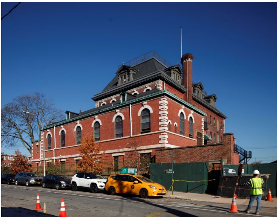
South Wing 64th Street facade (rear) Jessica C. Baldwin, November 2020
