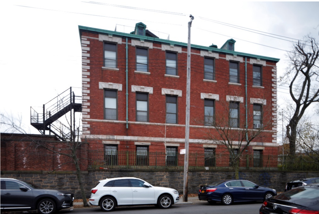
North Wing 63rd Street facade Jessica C. Baldwin, November 2020
