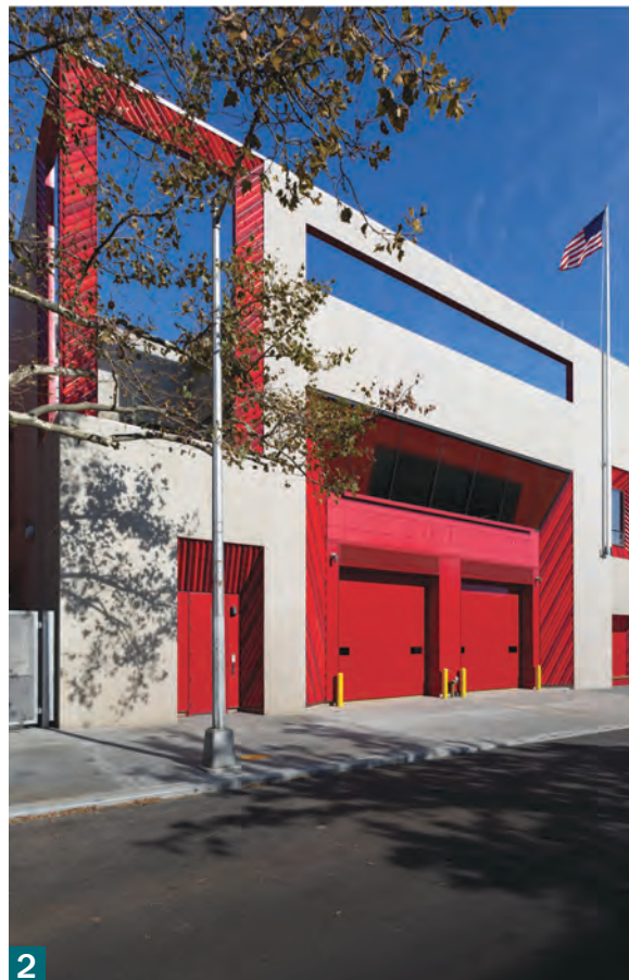
1. and 2. Construction of a firehouse, Rescue Company 2, Sterling Place between Howard Avenue and Saratoga Avenue, Brooklyn; Department of Design & Construction
