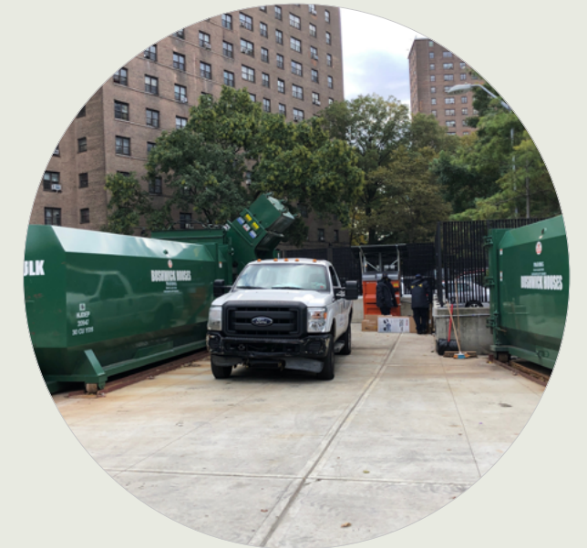
New bulk crusher at Bushwick Houses.
